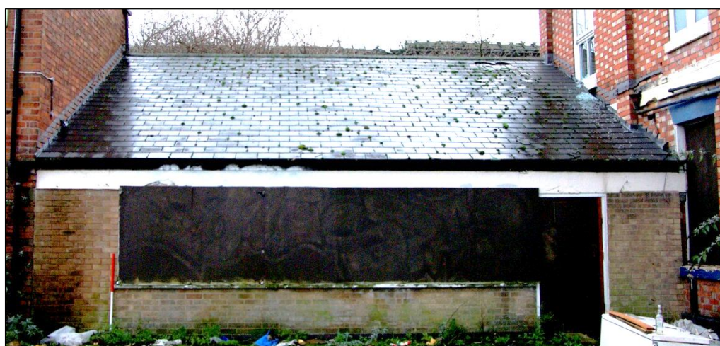
Figure 33. The stables and low extension, looking south with 1m scale
