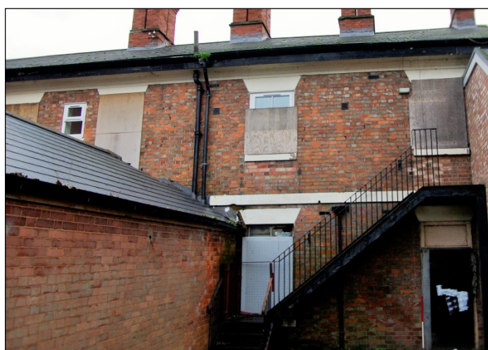
Figure 15. The eastern range seen from Newport Street, looking east, 1m scale.
