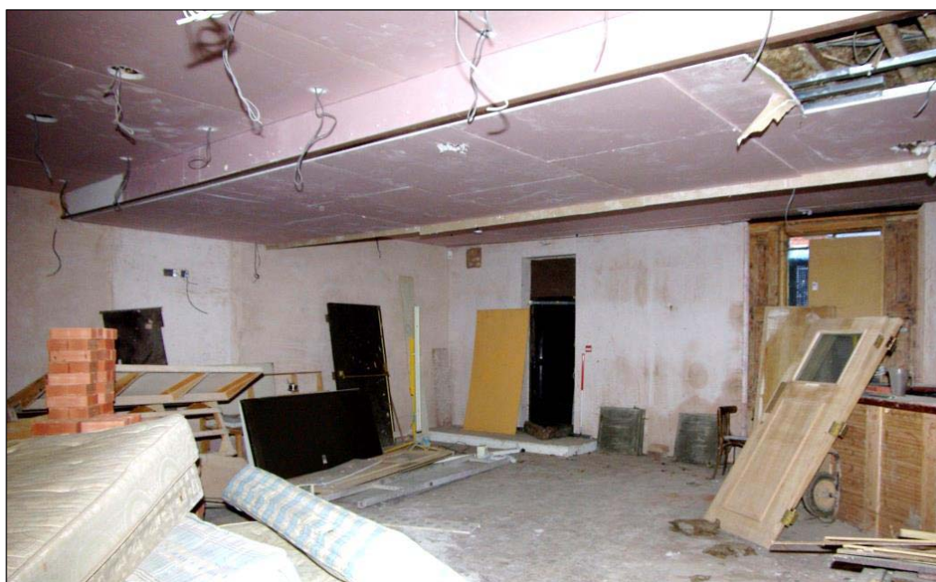
Figure 19. The southern lounge looking south west with 1m scale
