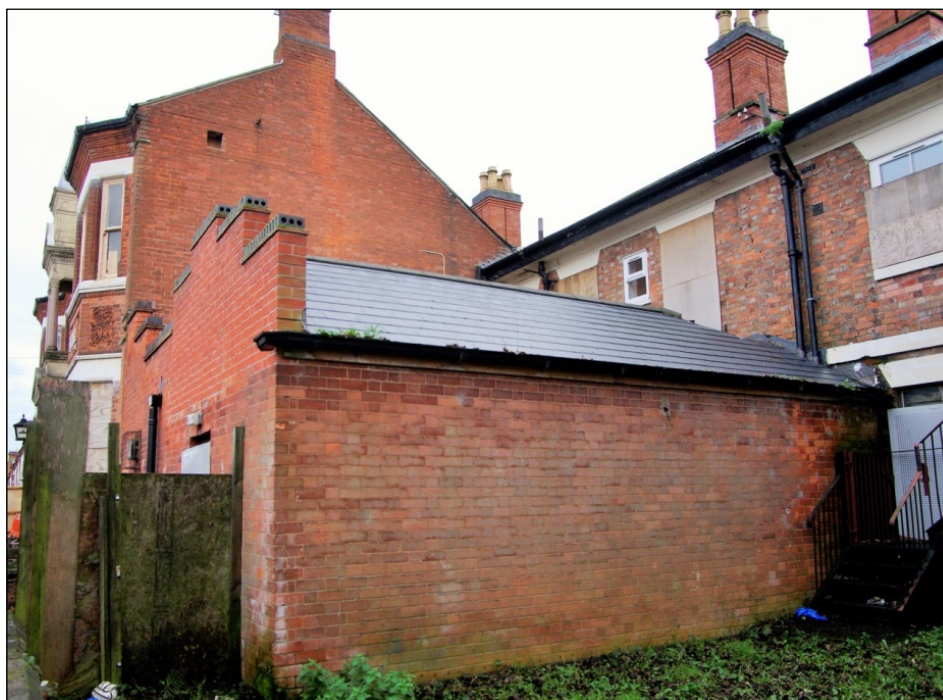
Figure 27. South facing elevation of the west range, looking north east
