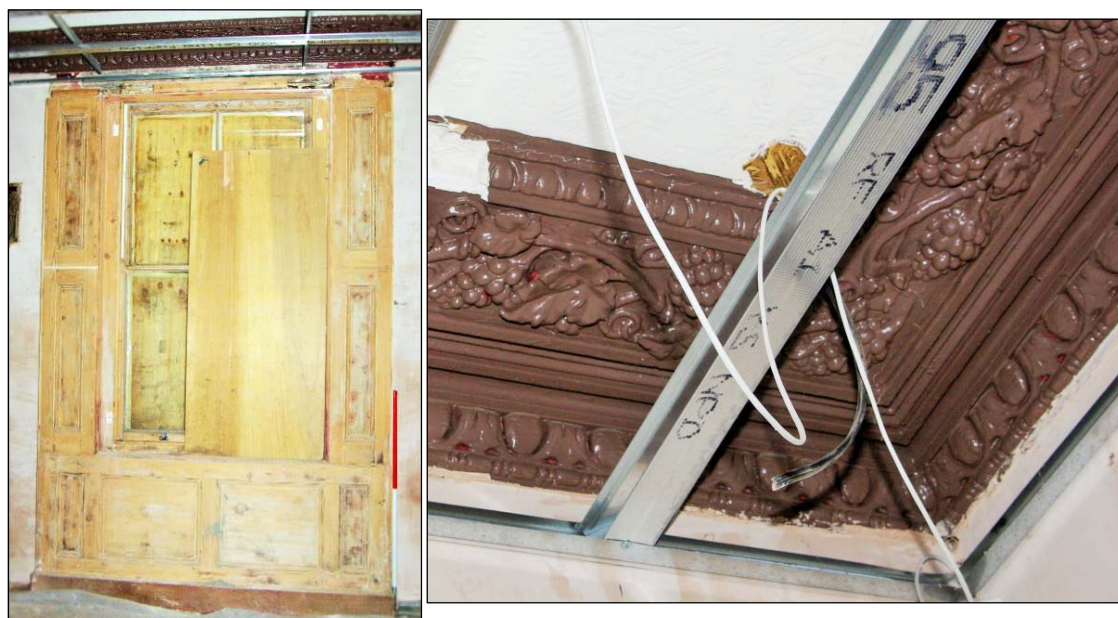
Figure 20. Surviving early details in the southern lounge, the panelling, looking east, with 1m scale (left) and cornicing (right)
