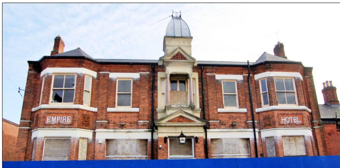
Figure 11. The west range, west elevation, fronting on to Newport Street, looking east.
