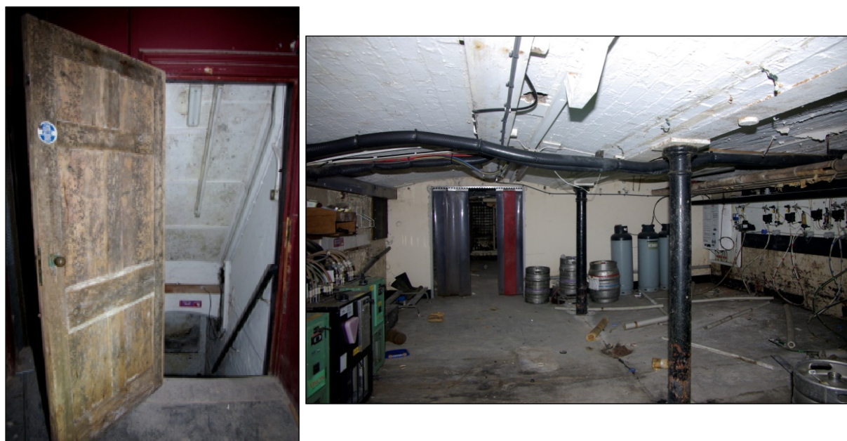
Figure 29. The basement stairs, looking north and the vaulted cellar, looking south
