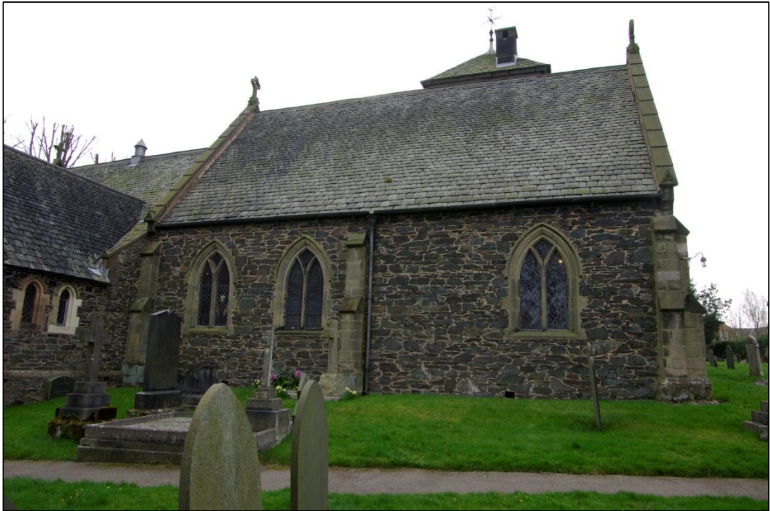
Figure 12. North wall, location of proposed single storey extension. Looking south.
