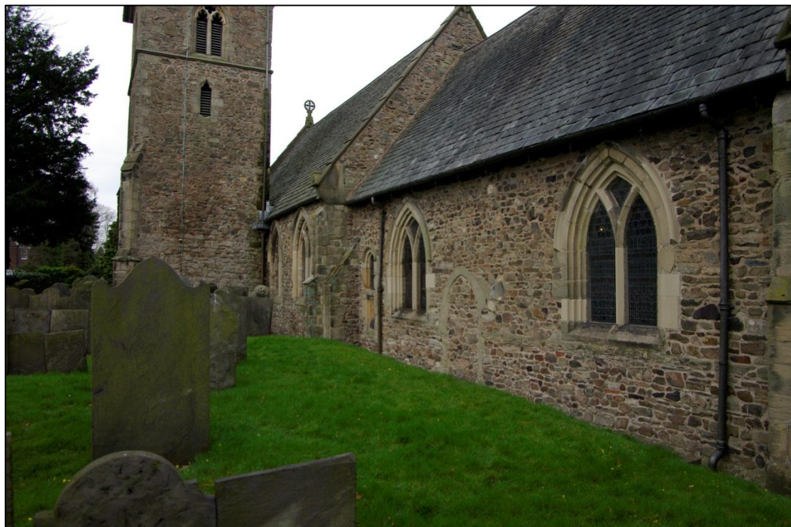
Figure 9. South elevation, looking north-west.
