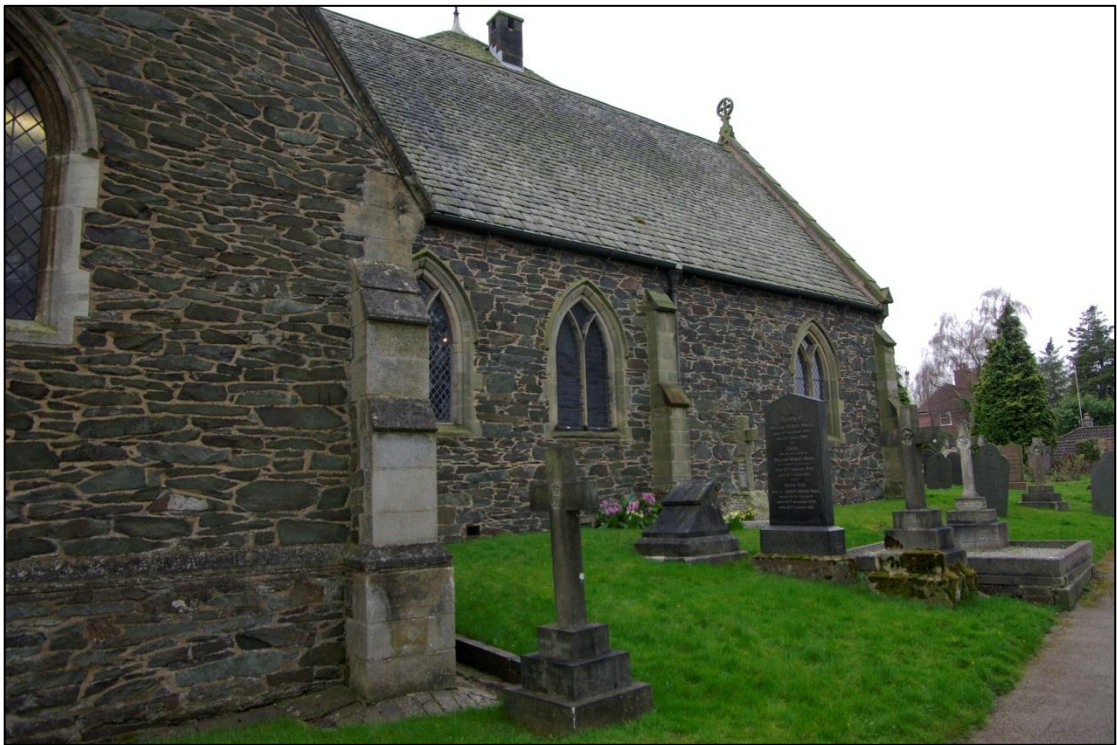
Figure 11. North elevation of nave, looking south-west.
