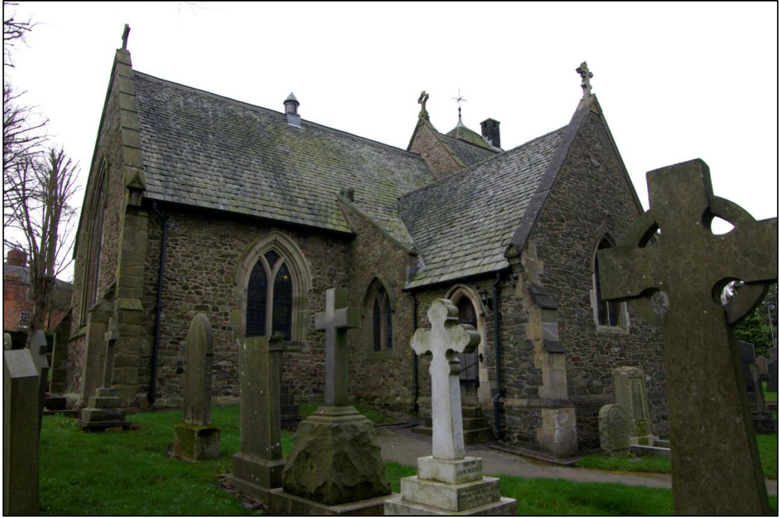
Figure 10. Vestry of 1927, looking south-west.
