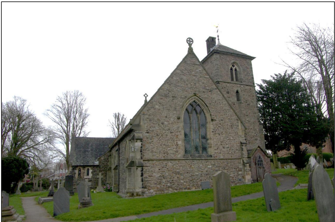
Figure 15. West elevation, looking east.
