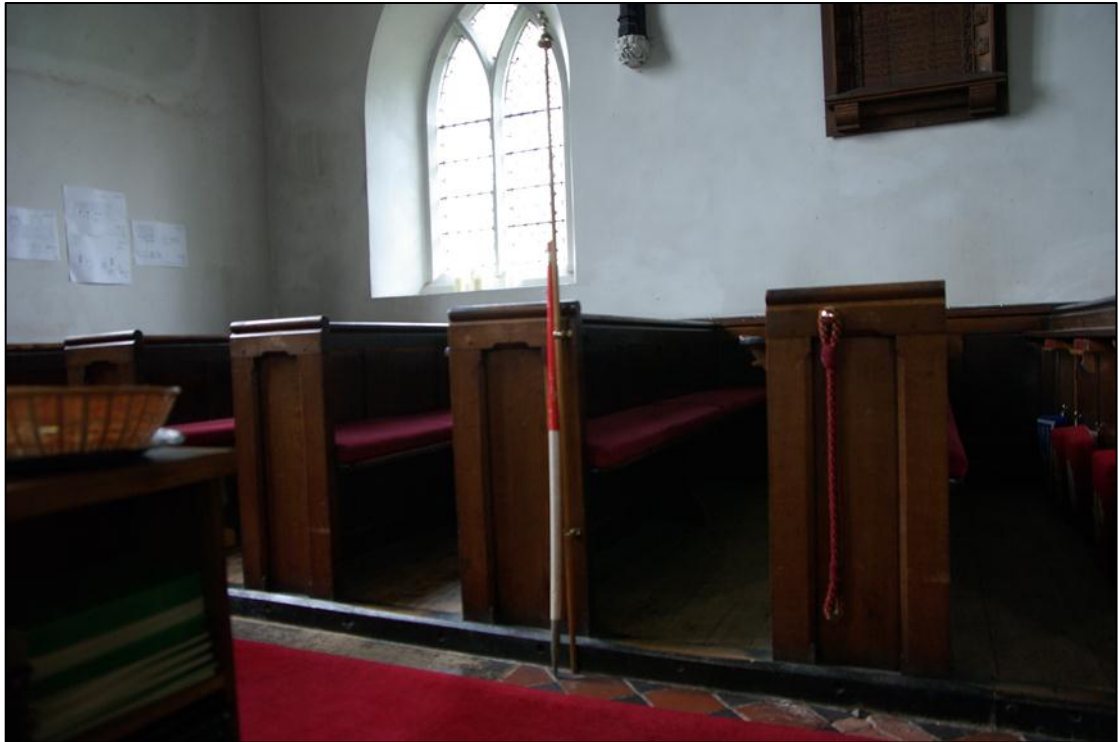
Figure 20. As above, with mid-19th century pews to be removed.
