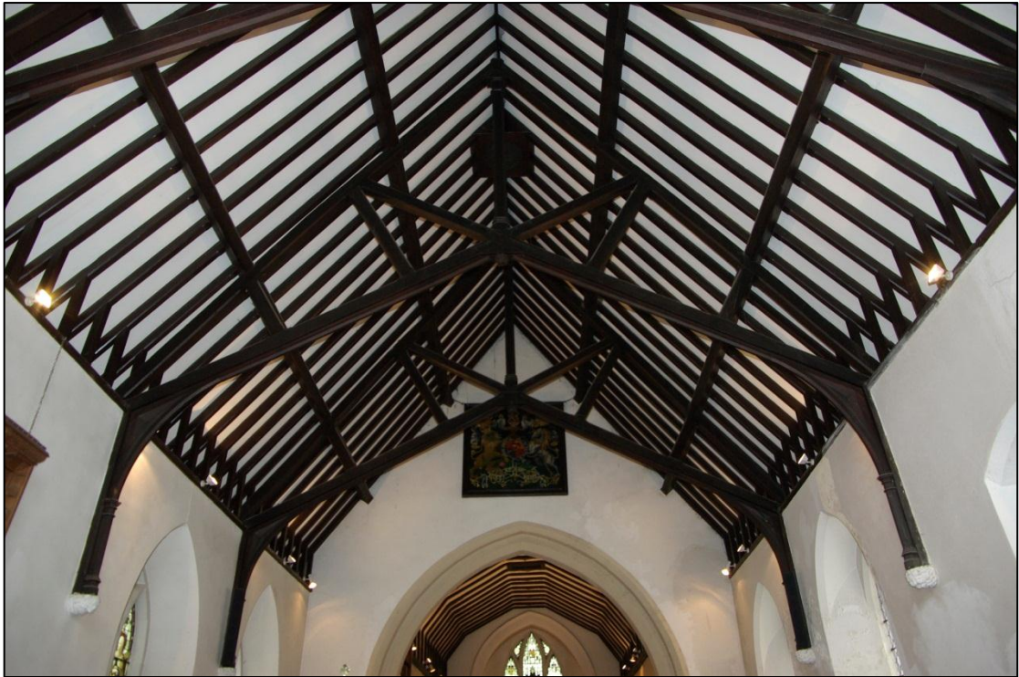
Figure 18. Scissor roof trusses over nave, looking east.
