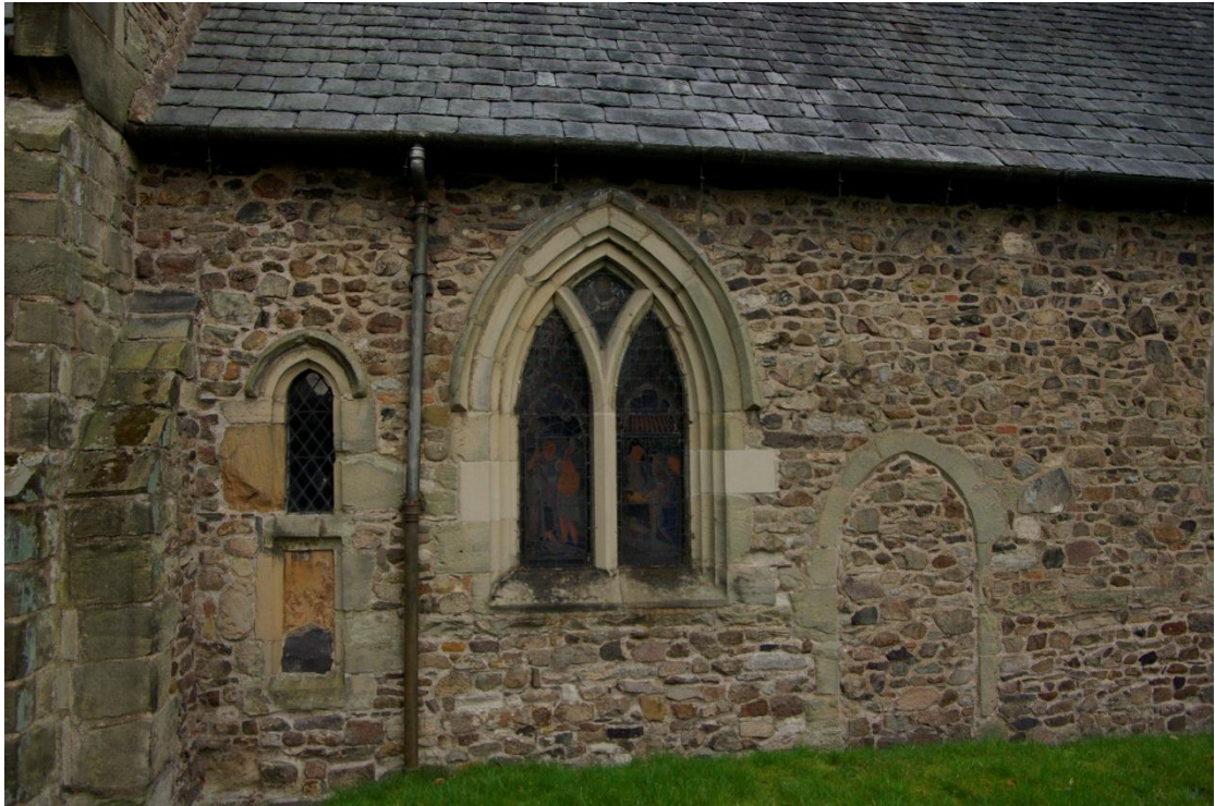
Figure 8. Windows and blocked openings on south elevation.
