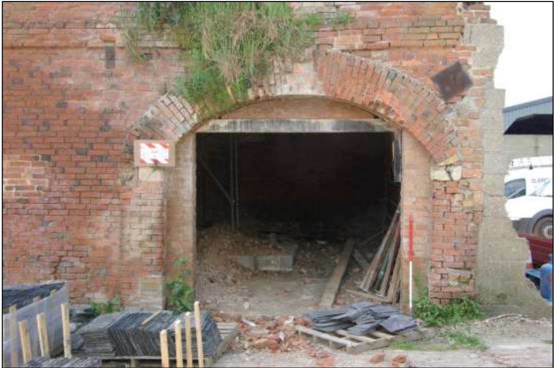
Figure 9. Entrance to cart-shed, looking south.
