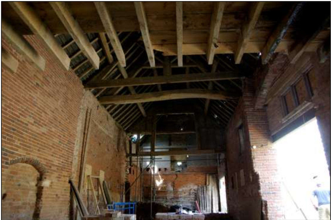
Figure 21. Barn interior, looking west, with winnowing door on left hand side.
