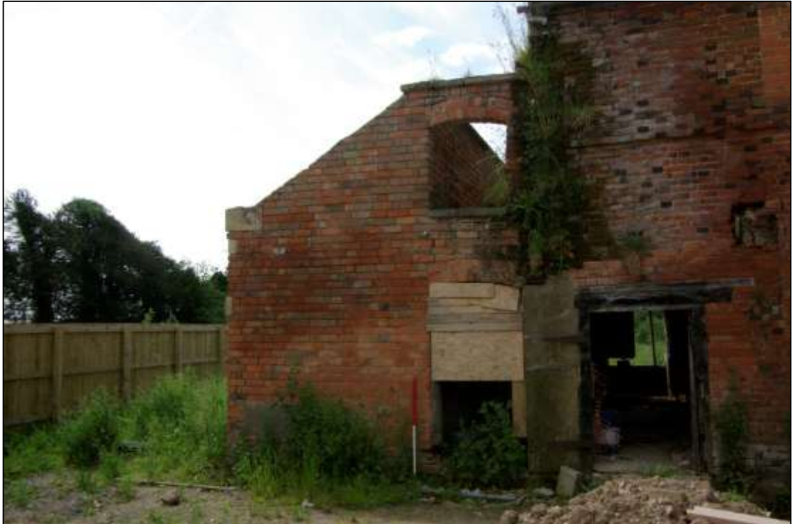
Figure 17. North facing elevation of auxiliary building. Looking south.
