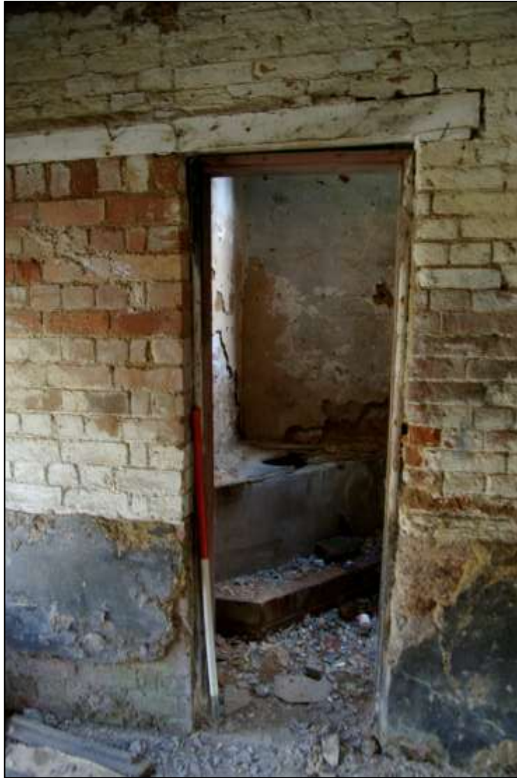
Figure 22. Privy toilet located in auxiliary building, looking west.
