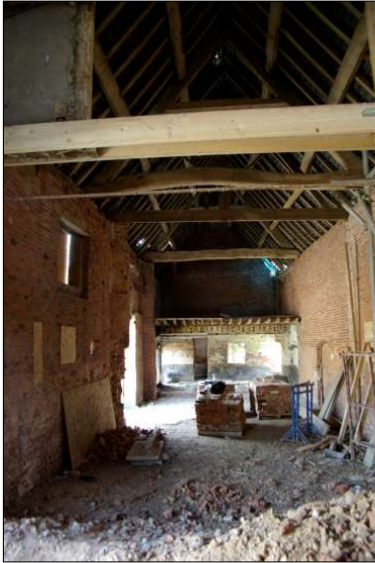
Figure 19. Barn interior, looking east.
