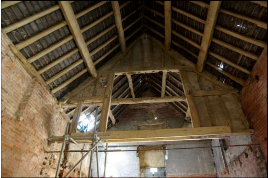
Figure 20. Truss 4, looking west.
