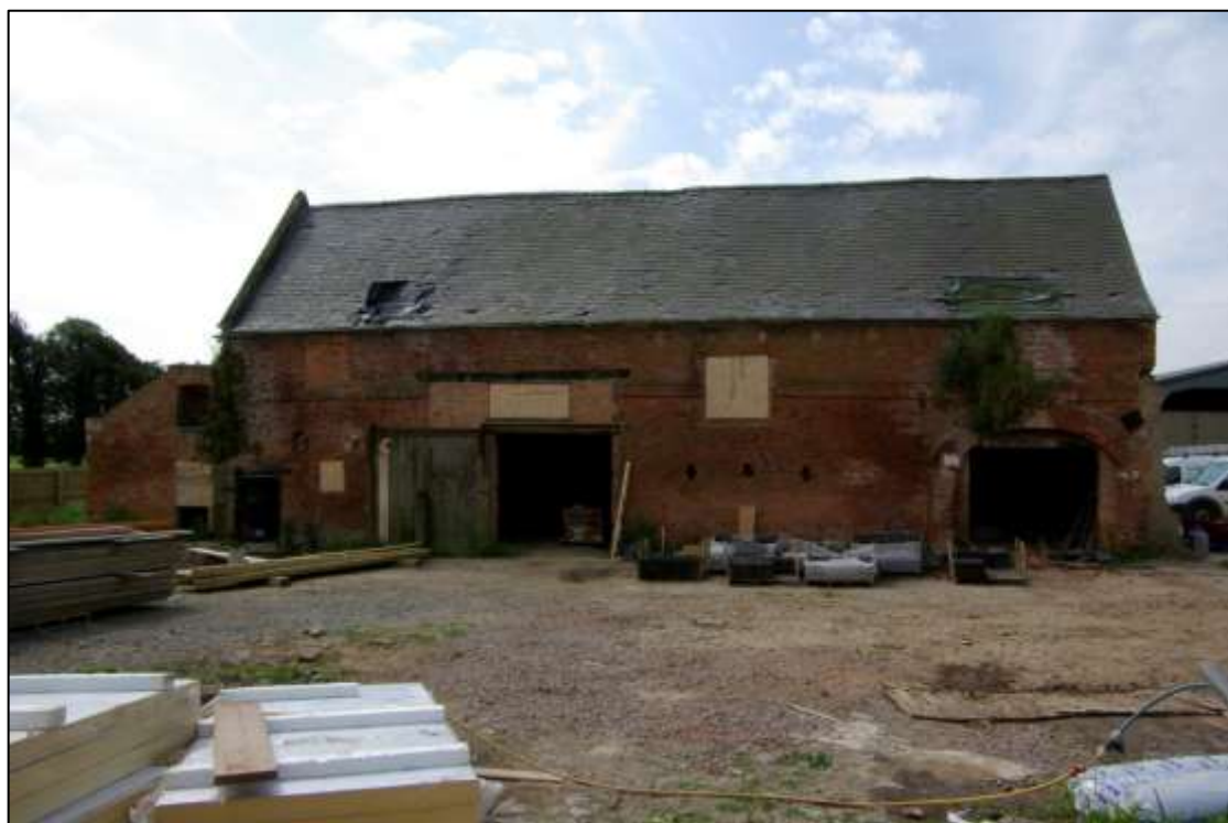
Figure 8. North-facing farmyard elevation, looking south.
