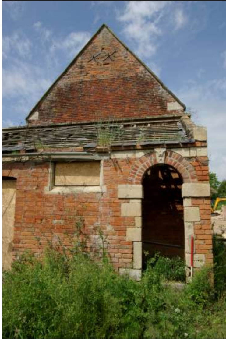
Figure 14. Auxiliary structure against eastern gable end. Looking west.
