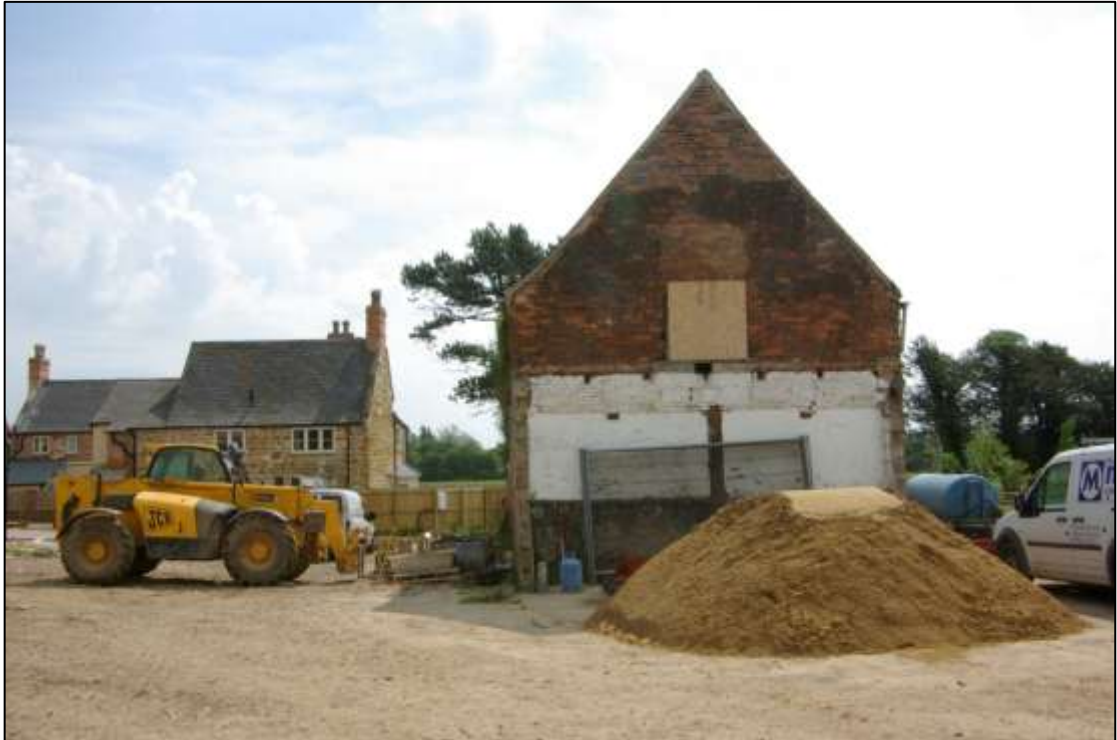
Figure 11. West-facing gable-end, looking east.
