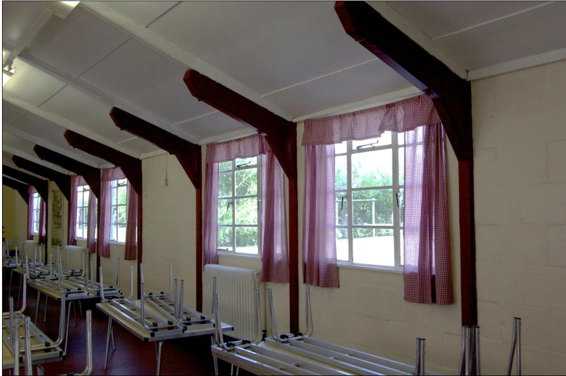
Figure 11. Crittal-style windows, looking north-west.
