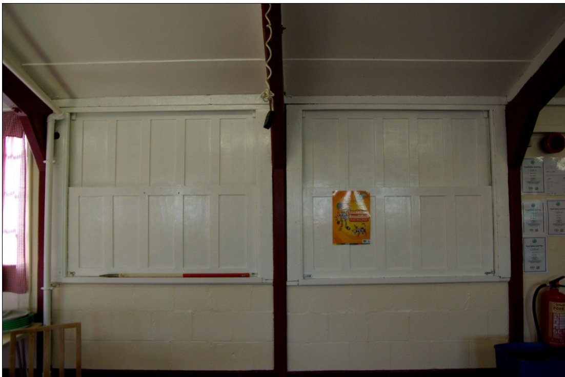
Figure 12. Timber shutters to serving hatch, looking south.
