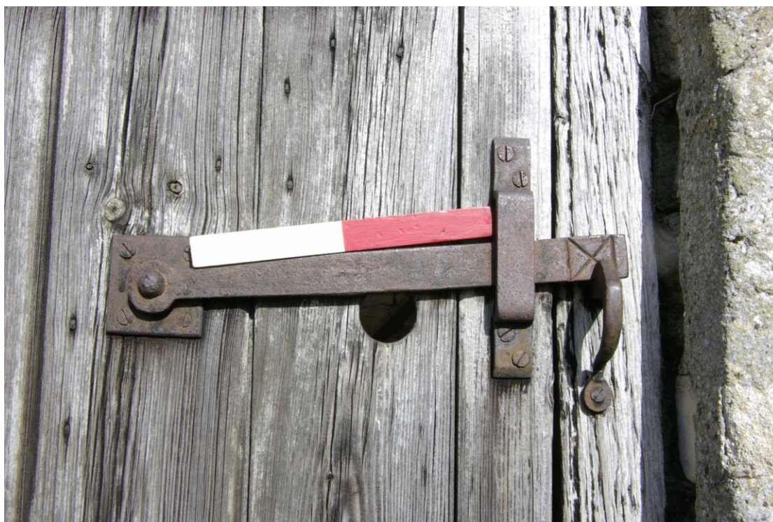
Figure 16 Latch on converted stable door 10cm scale
