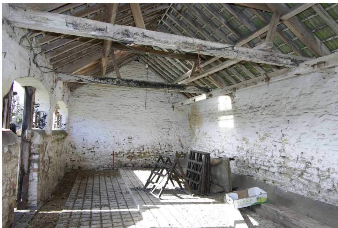
Figure 22 Building 1, west room of enclosed rooms Looking north west. 1m scale. Note beam with hooks/latches attached to underside of truss on right of picture
