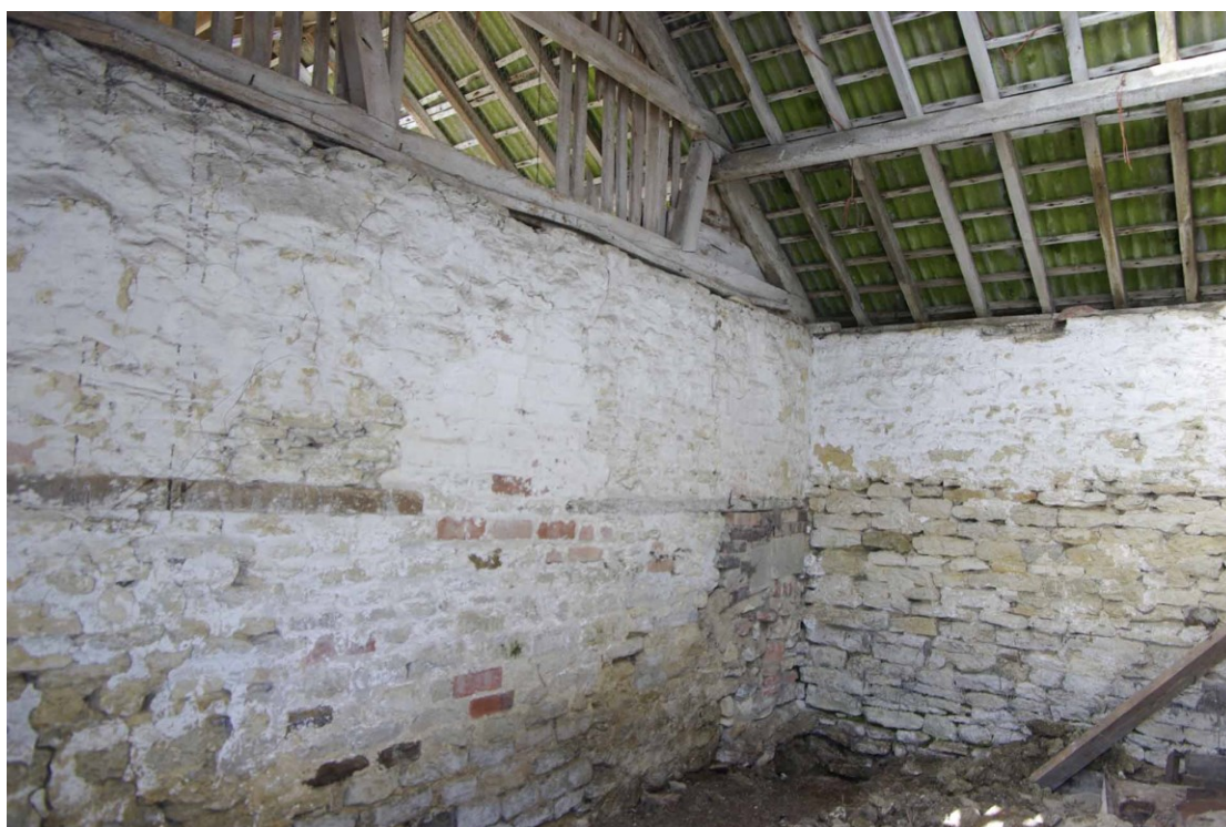
Figure 18 Building 1, inserted wall creating stable room from open bay Looking north west
