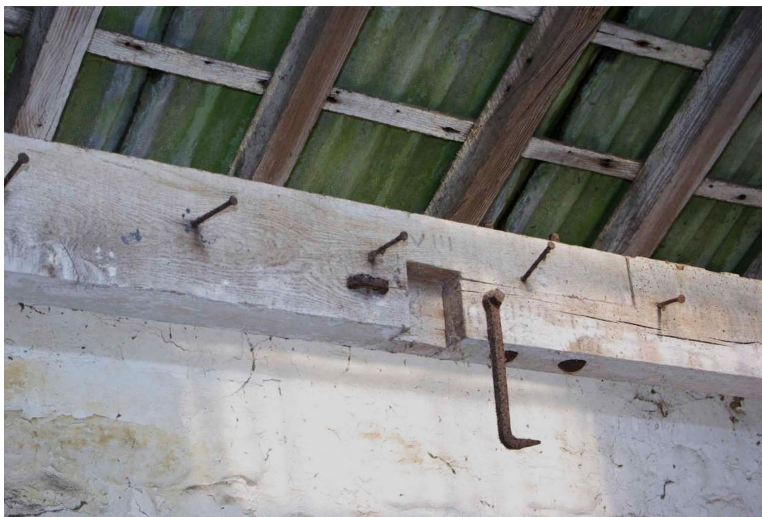
Figure 24 Building 1, numbered hooks/latches
