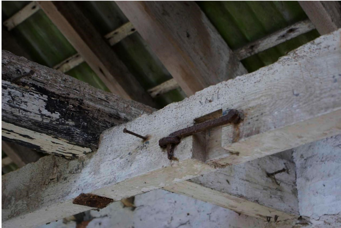
Figure 25 Building 1, numbered hooks/latches
