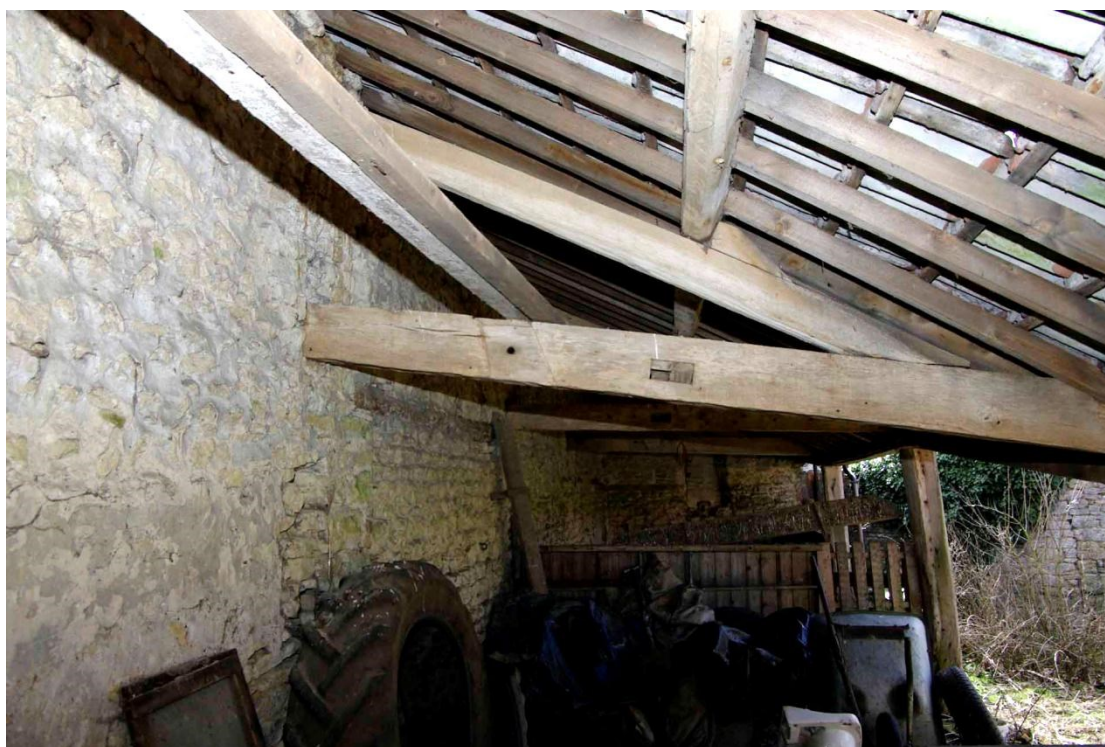
Figure 44 Building 3b roof structure Looking south. Note re-used timbers
