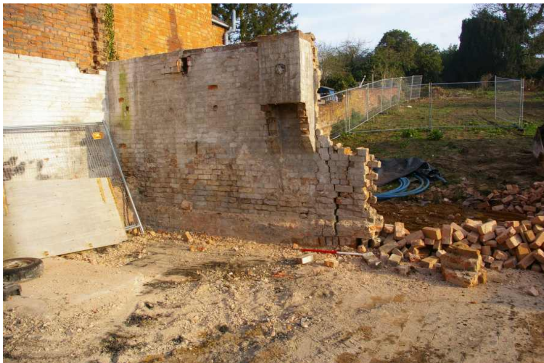
Figure 25 North wall during demolition Looking north west. 1m scale
