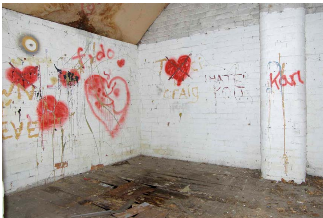
Figure 23 First floor, east room Looking north-east
