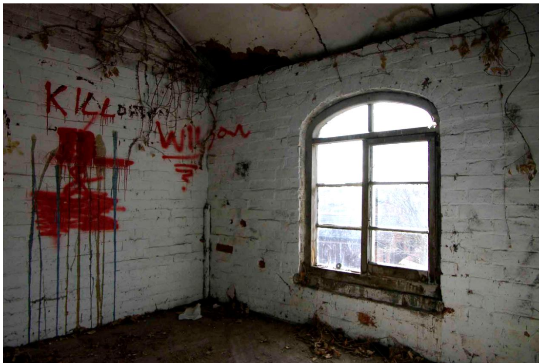
Figure 24 First floor, east room Looking south-east
