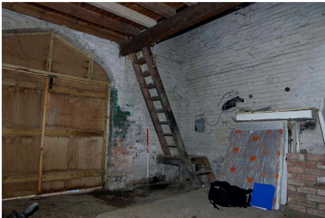
Figure 18 Ground floor, west room Looking south-west. 1m scale
