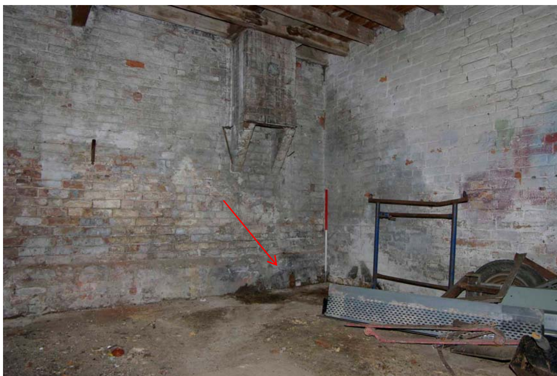
Figure 19 Ground floor, west room Looking north-east. 1m scale Note truncated chimney and ground floor arch (arrowed)
