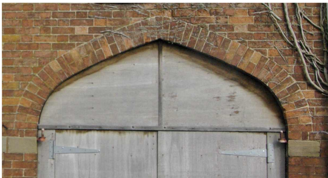
Figure 10 Arch and pintle detail
