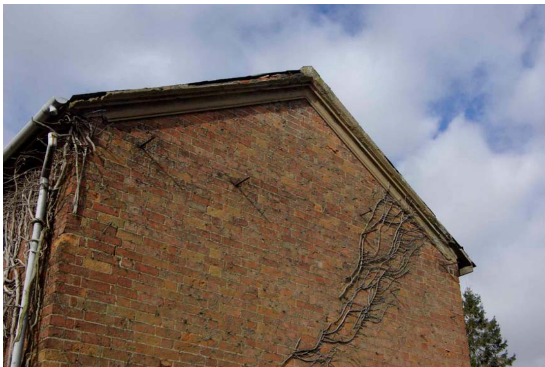
Figure 12 Moulding detail on east facing elevation
