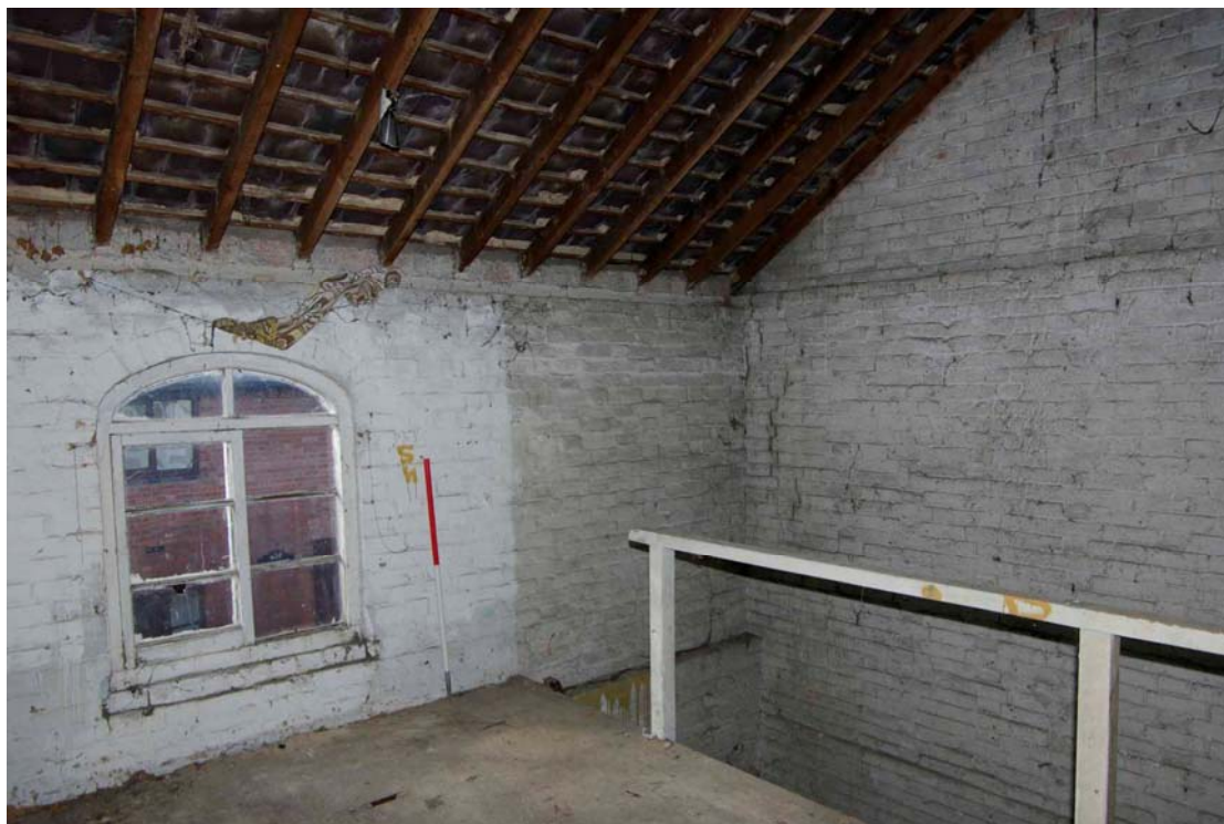
Figure 20 First floor, west room Looking south-west. 1m scale
