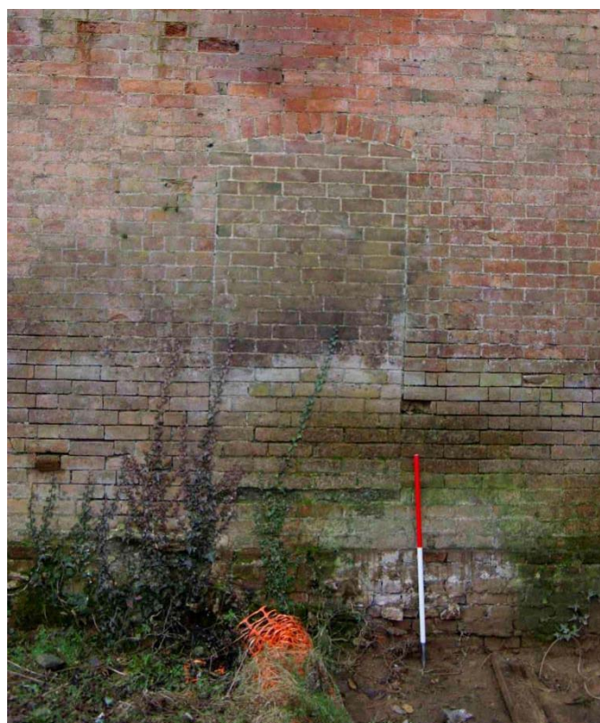
Figure 14 Blocked doorway, north-facing elevation Looking south. 1m scale
