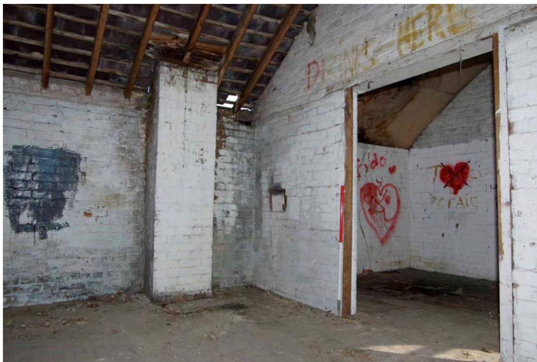
Figure 21 First floor, west room Looking north-east. 1m scale
