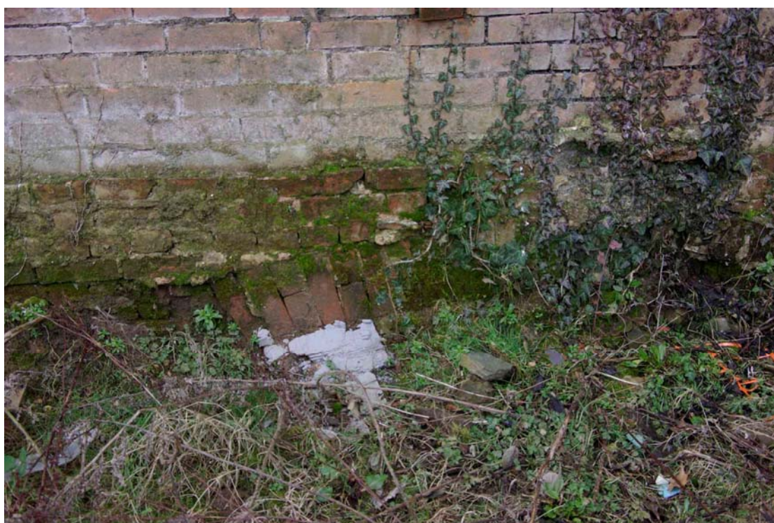
Figure 15 Arch at ground level on north-facing elevation Looking south
