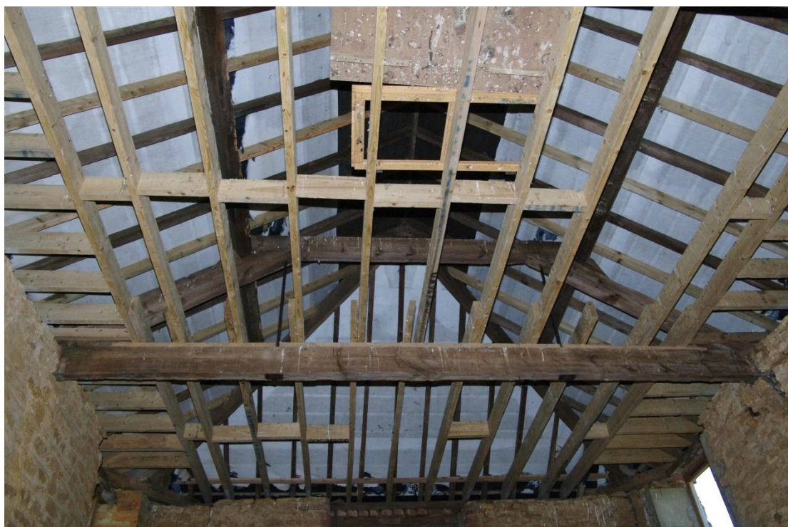
Figure 21 Old Barn, roof structure Looking south
