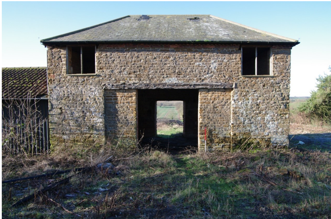
Figure 9 Old Barn, east facing elevation Looking west. 1m scale
