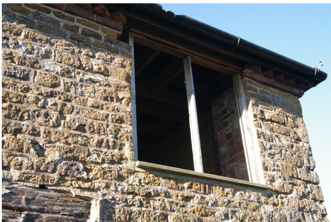
Figure 11 Old Barn, east facing elevation window detail Looking north-west. Note the sawn stonework at either side of the window and how the window cuts the brick eaves
