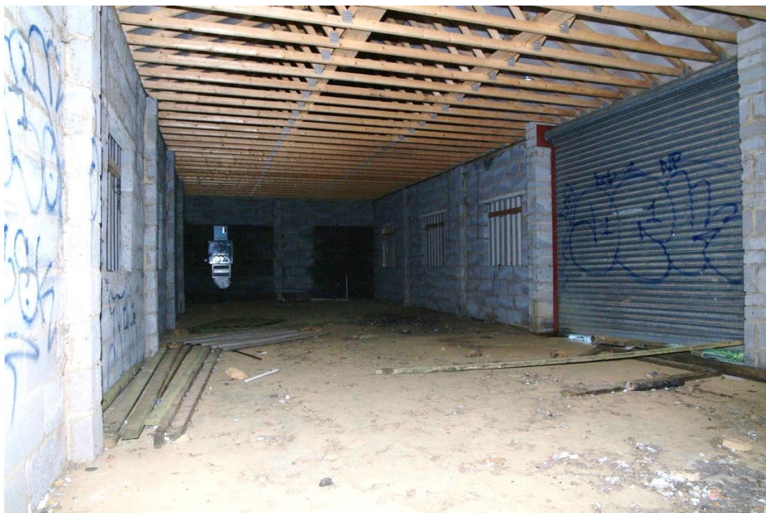
Figure 24 Modern barn, inside Looking south-west
