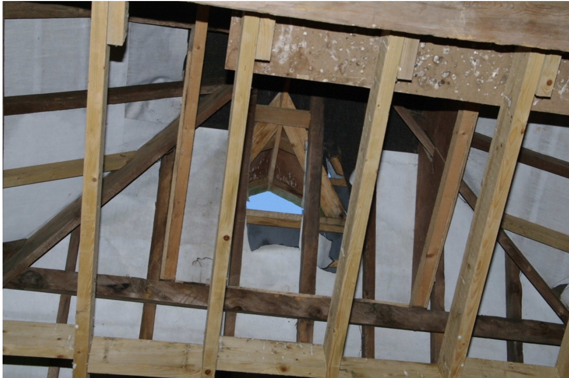
Figure 22 Old Barn, vent in roof Looking north
