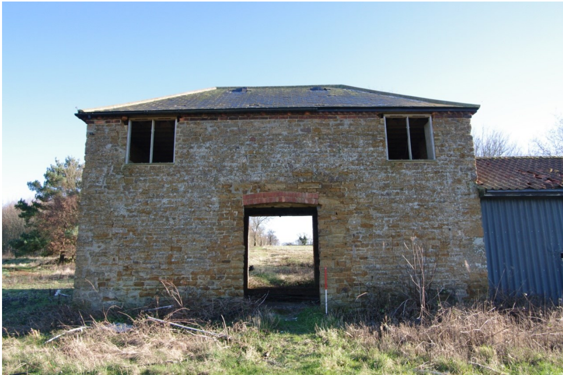
Figure 13 Old Barn, west facing elevation Looking east. 1m scale
