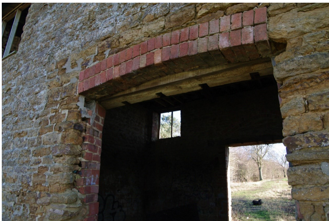
Figure 14 Old Barn, west facing elevation doorway detail Looking north-east
