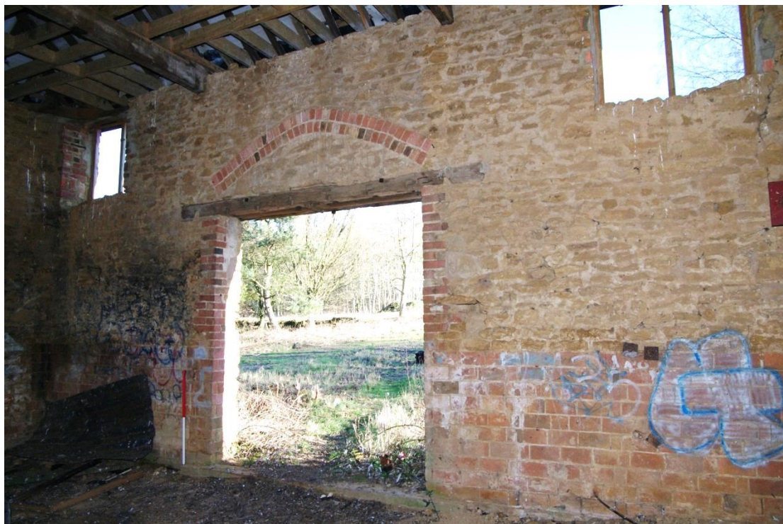
Figure 20 Old Barn, inside of east wall Looking north-east. 1m scale
