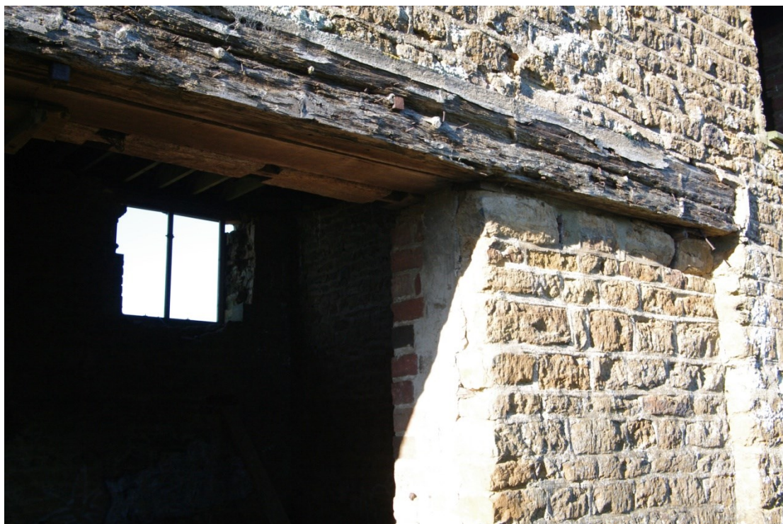
Figure 10 Old Barn, east facing elevation door detail Looking north-west
