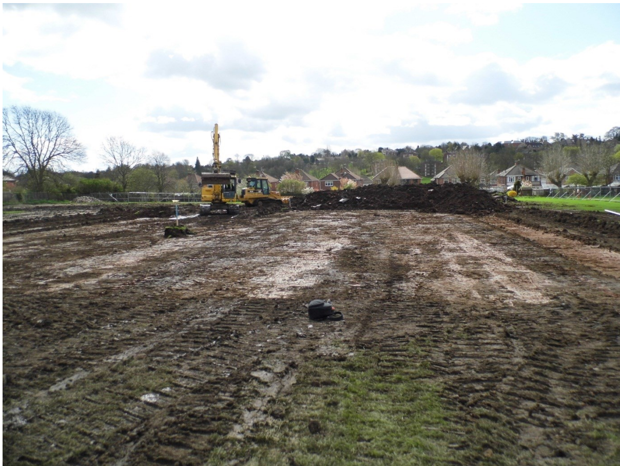
Figure 3 Removal of sub-soil, showing ridge and furrow. Looking South
