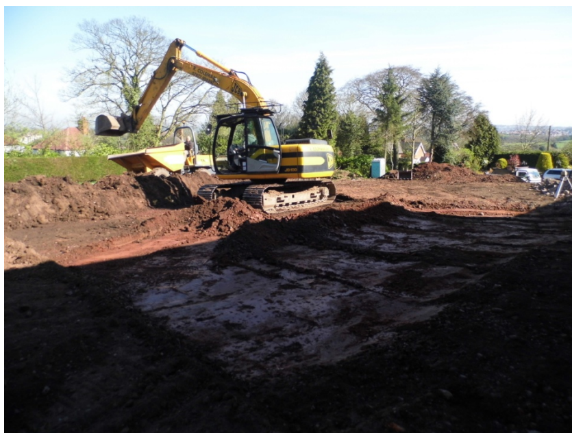
Figure 4: Top-soil stripping. Looking North
