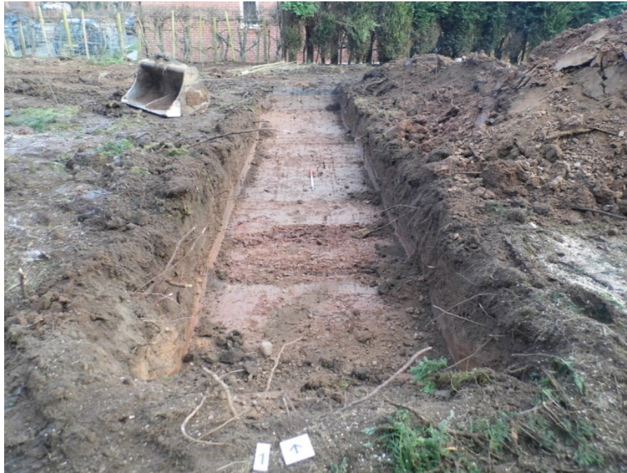
Figure 5: Trench 1 looking north
