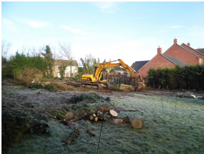
Figure 4: Site area, looking north.
