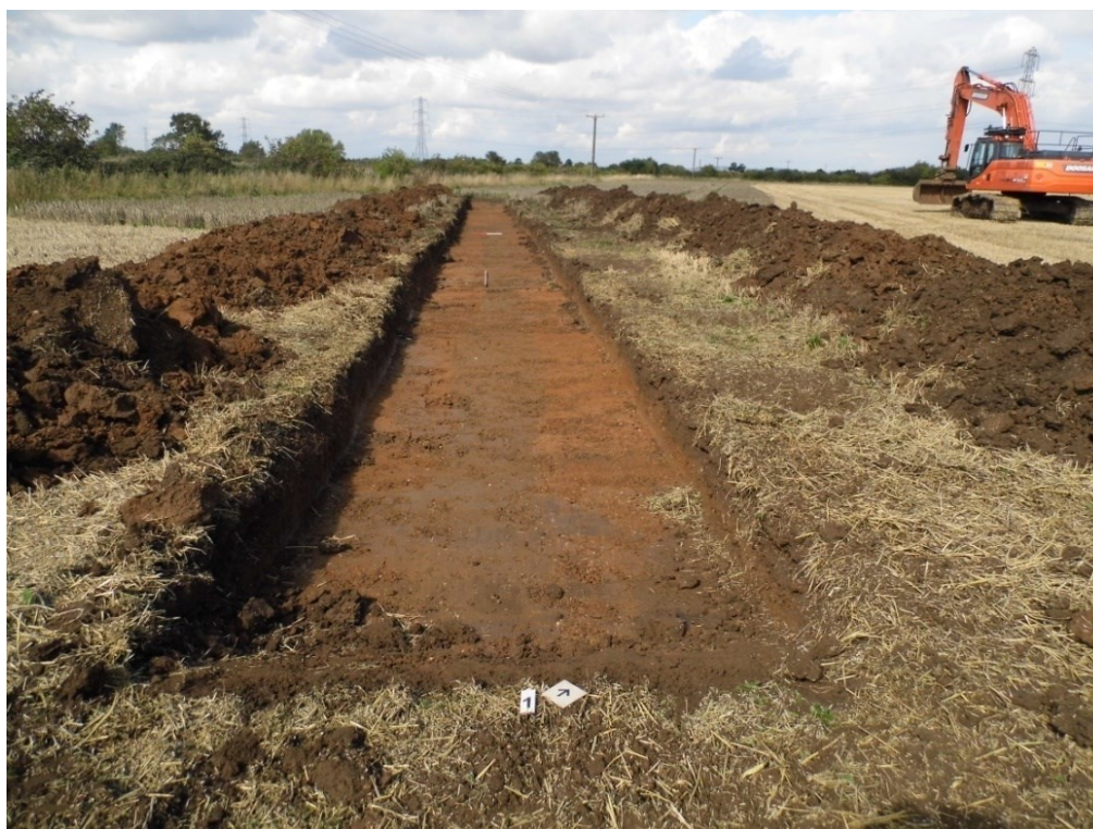
Figure 9: Trench 1 looking North
