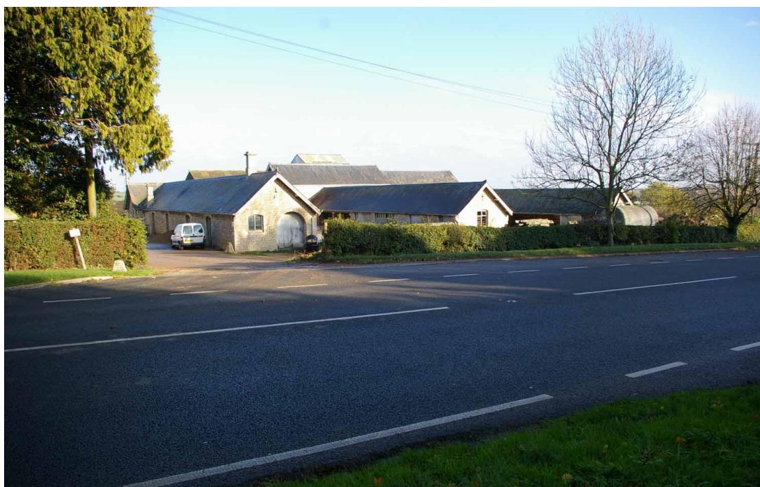
Figure 8 General view of farm buildings from A606 Looking north east
