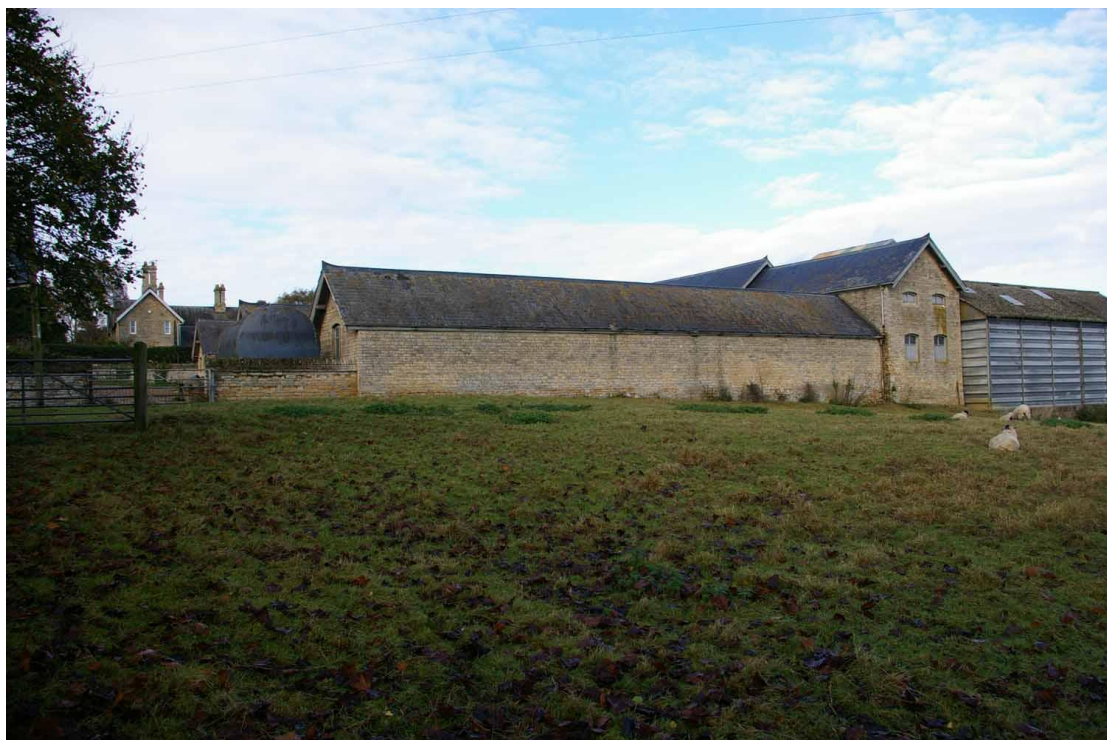
Figure 15 East facing elevation Looking west north-west
