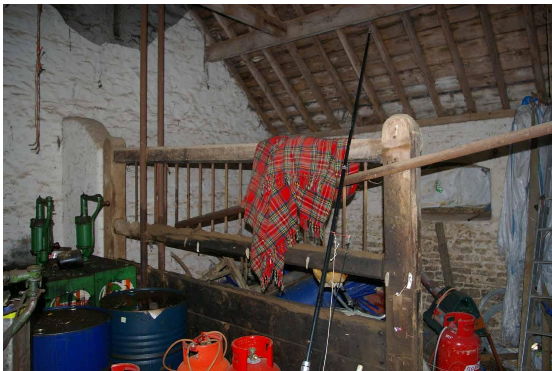
Figure 19 West wing, loose box Looking north east
