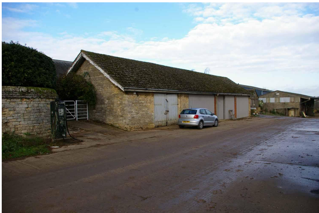
Figure 25 Cart shed Looking north-west
