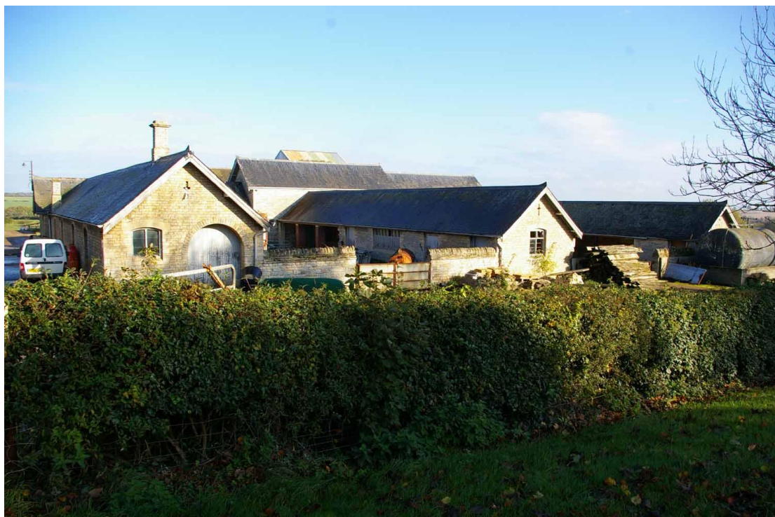
Figure 11 South facing elevation Looking north-east
