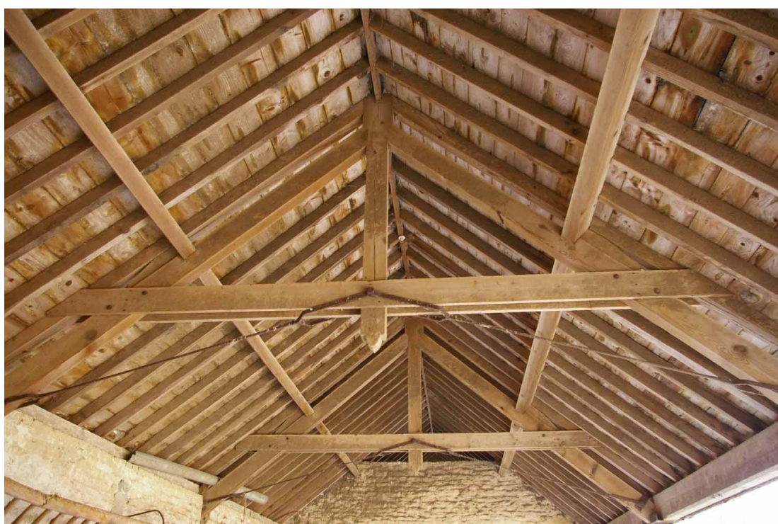
Figure 14 Roof structure detail Eastern cattle shed. Looking south
