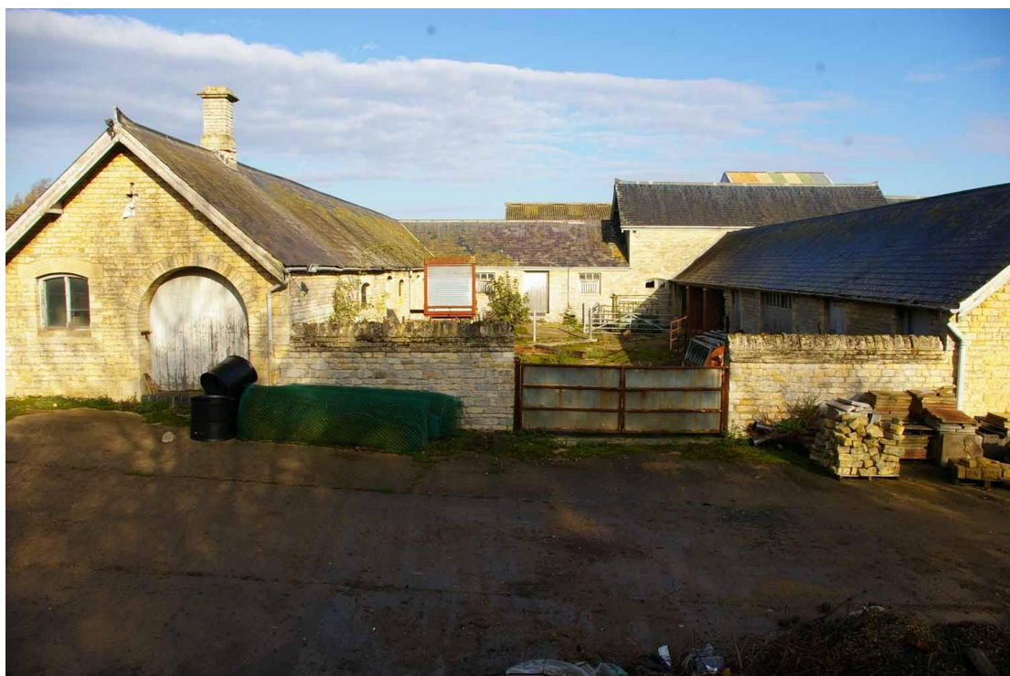
Figure 12 Western courtyard, south facing elevation Looking north. Note decorative ridge details at gable ends
