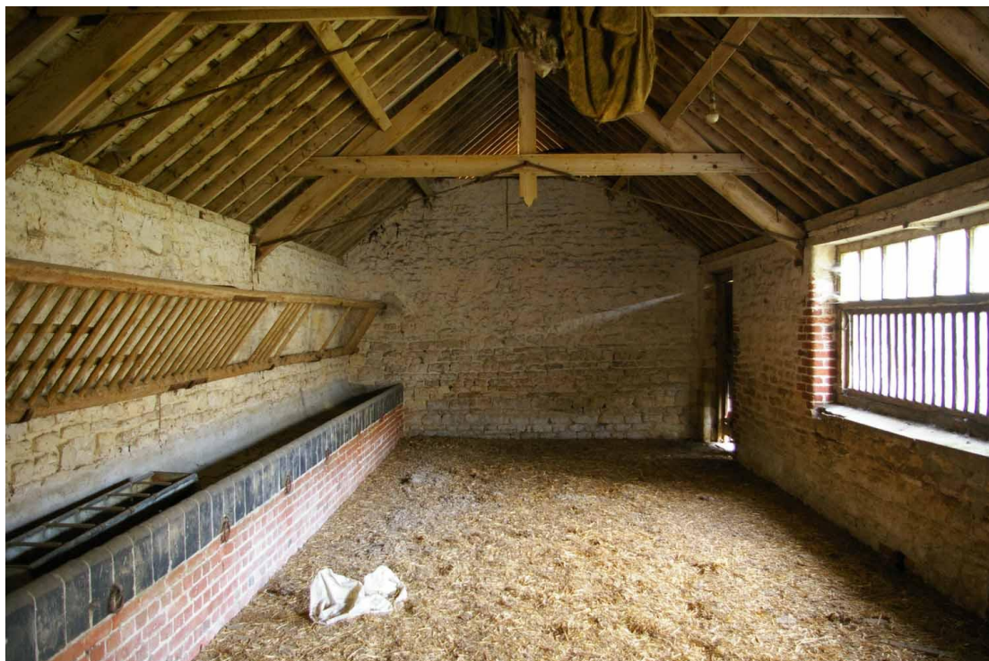
Figure 21 Centre wing stable Looking south
