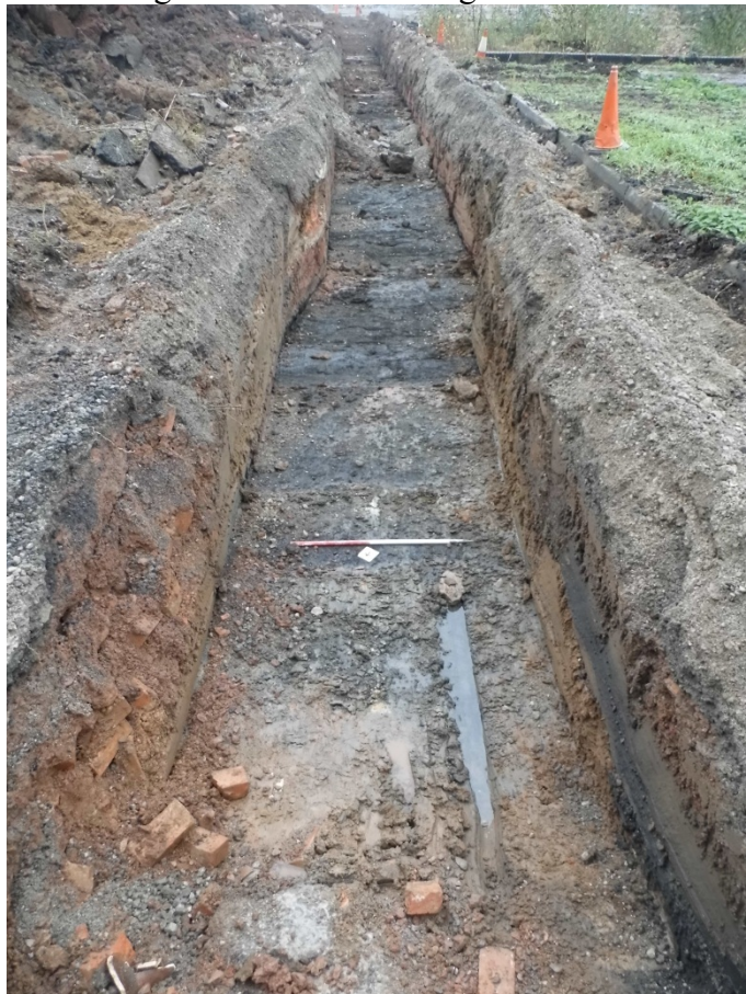
Figure 6: Trench looking south-east
