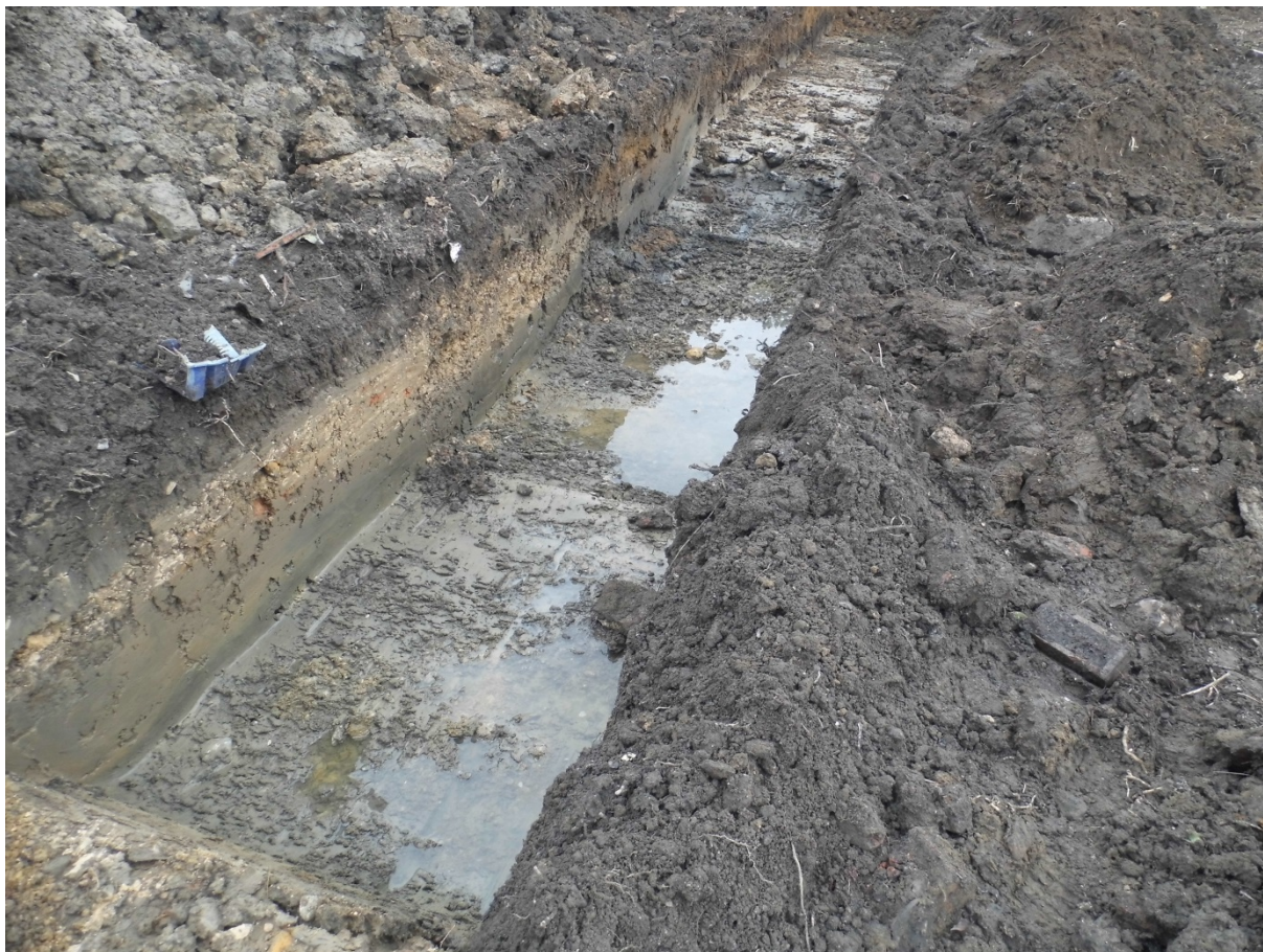
Figure 5: Trench 1 looking north
