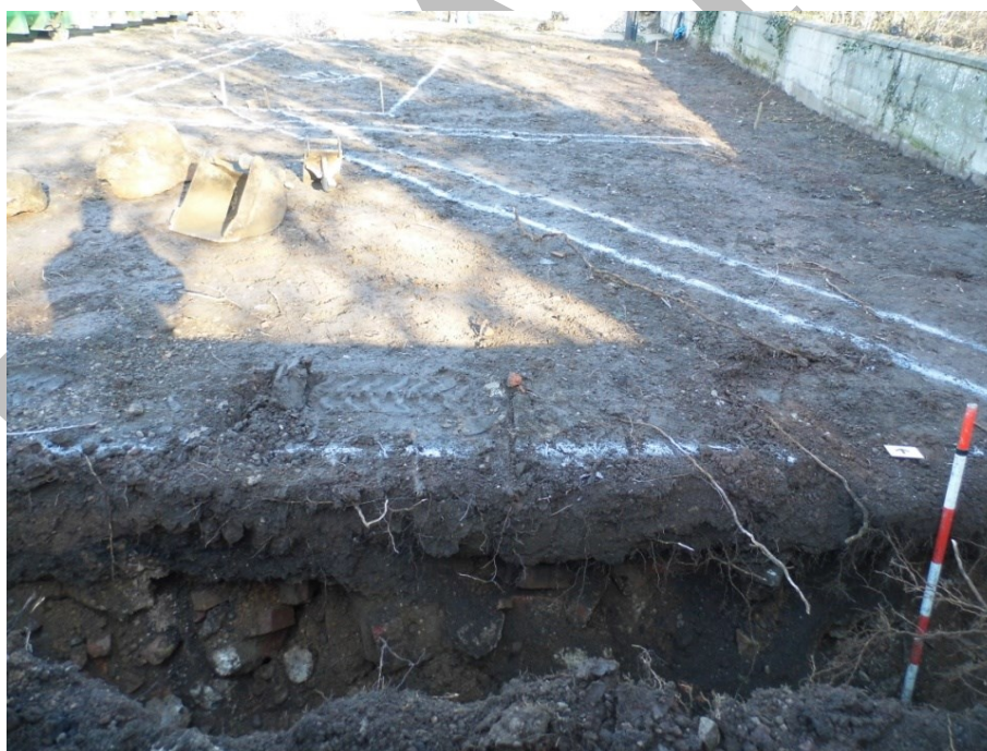
Figure 7: Excavation of pipe trench showing brick and concrete rubble. Looking North.
