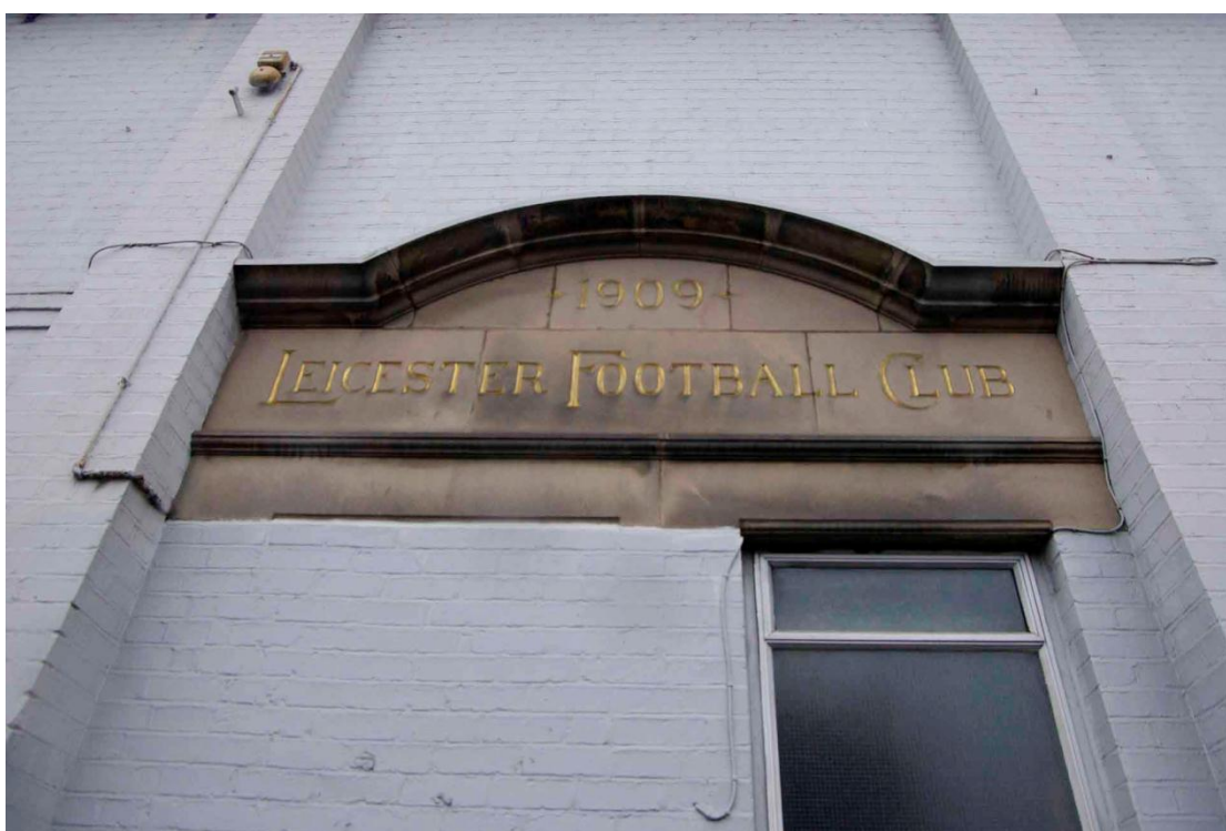
Figure 8 Former Clubhouse entrance Note blocked doorway on left of picture
