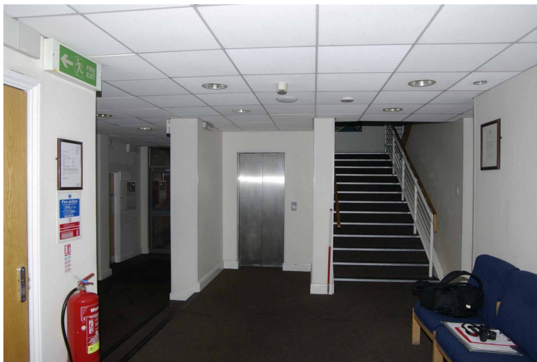
Figure 23 Entrance hallway into northern building Looking west. Shop doorway is to right of photograph at the bottom of the stairs
