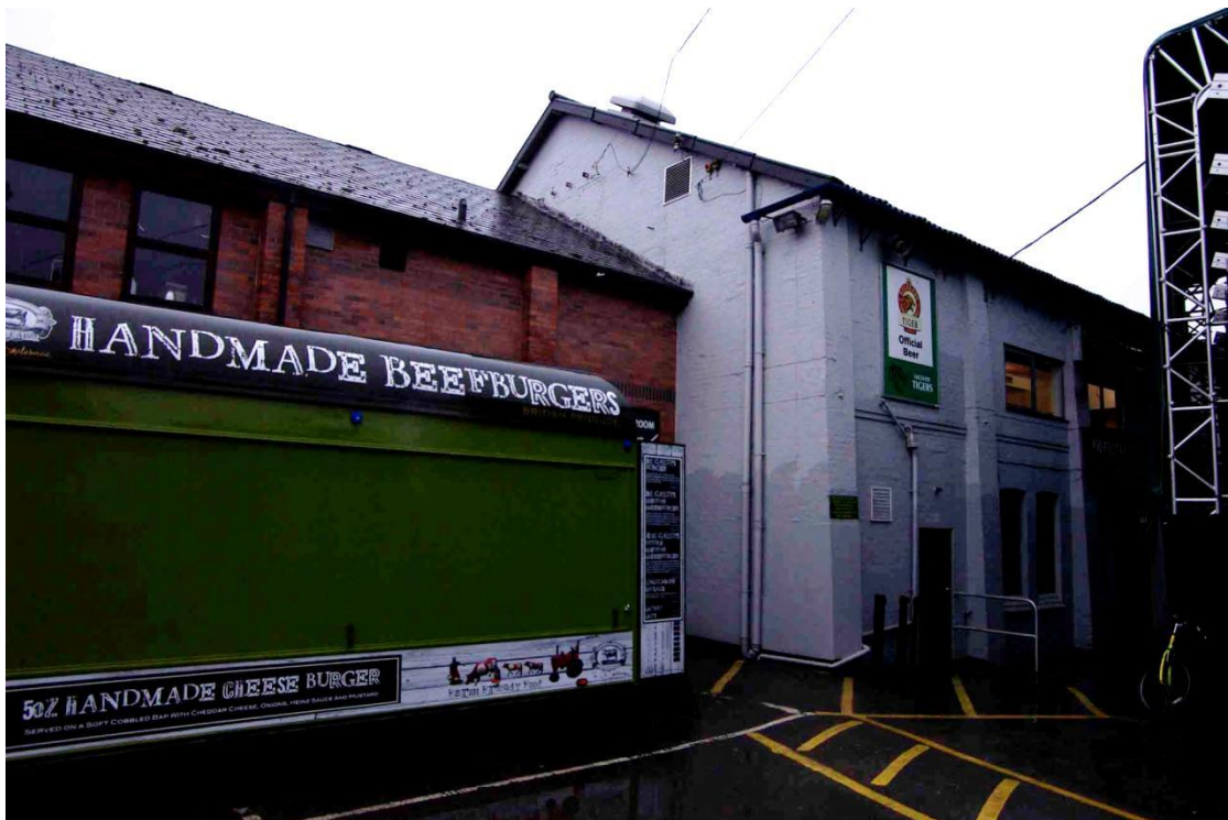
Figure 12 Junction of 1909 Clubhouse and southern building Looking north-west
