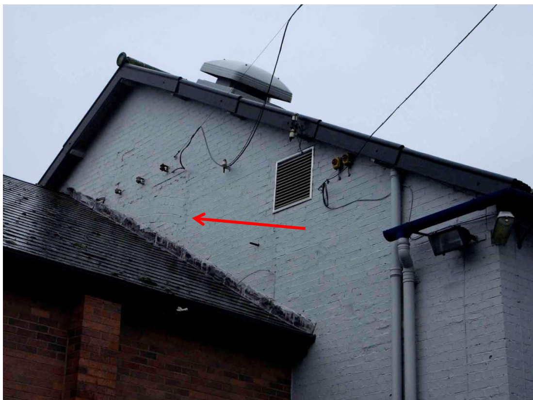
Figure 13 South gable end of 1909 Clubhouse Looking north-west. Blocked window arrowed
