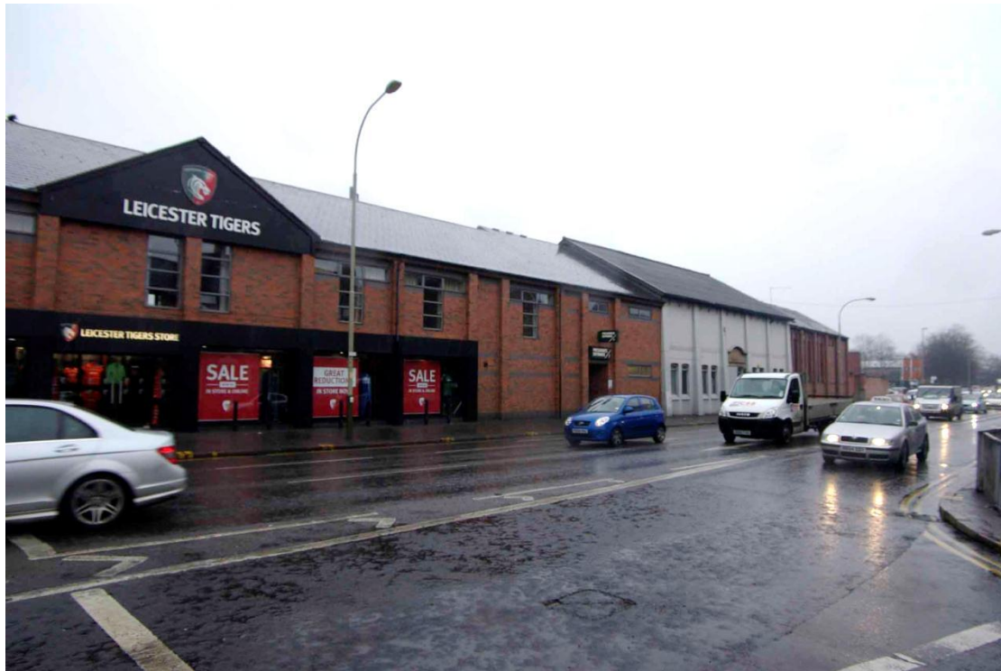
Figure 3 Clubhouse from Aylestone Road Looking south-east
