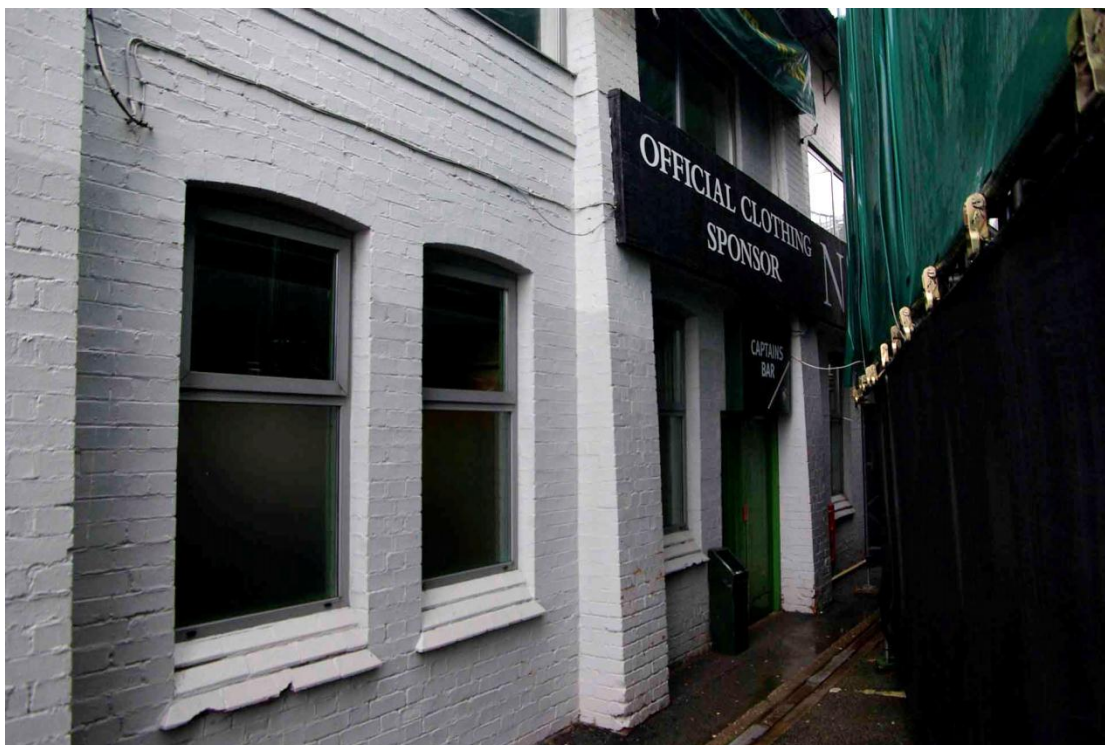
Figure 15 1909 Clubhouse, east facing elevation ground floor windows Looking north
