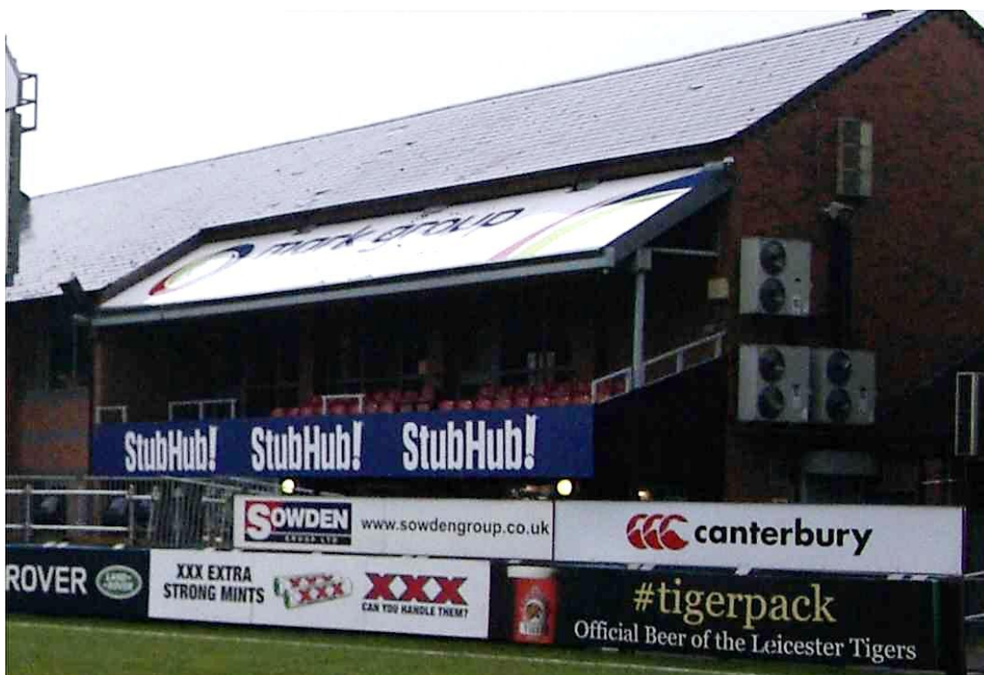
Figure 16 Northern building, east facing elevation Looking south-west
