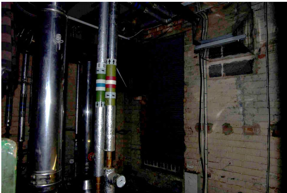
Figure 21 Boiler room Looking north-east. Note blocked window
