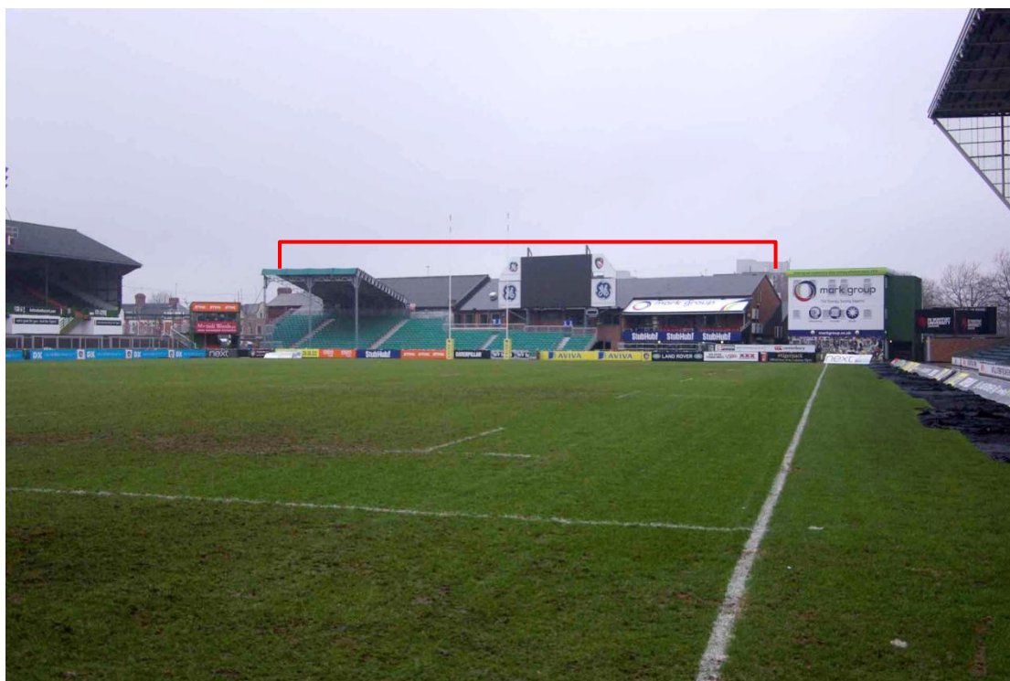
Figure 5 Clubhouse seen from east stand Looking west. Clubhouse buildings are highlighted
