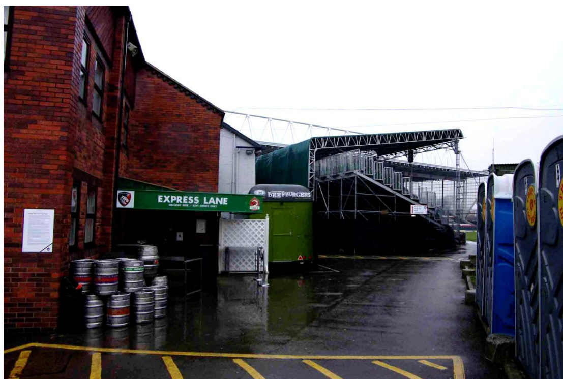
Figure 14 Southern building Looking north. Note step in wall line
