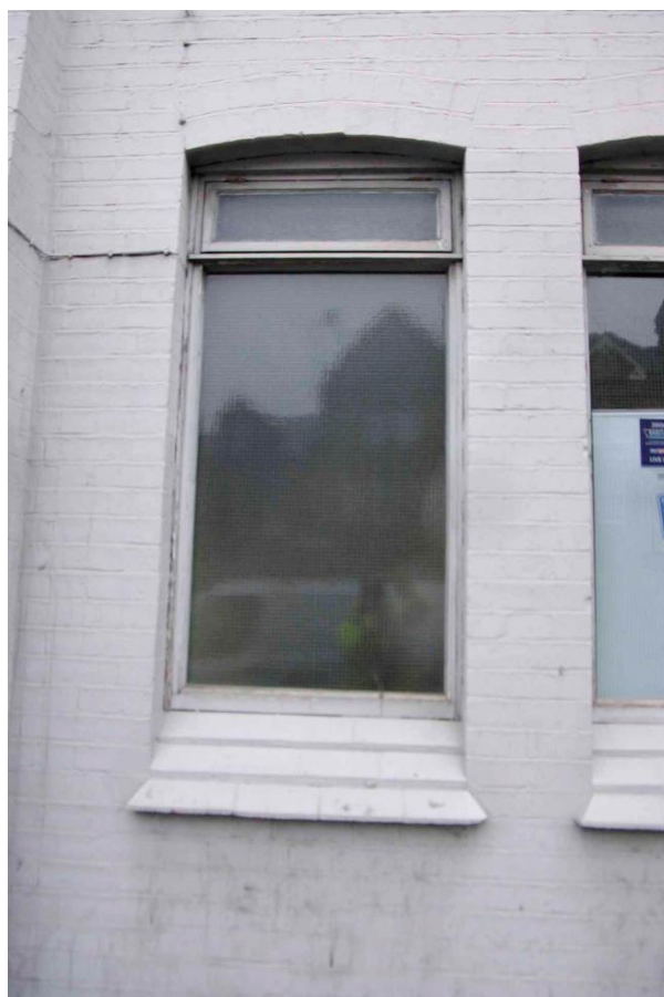
Figure 9 West facing elevation window detail Clubhouse building
