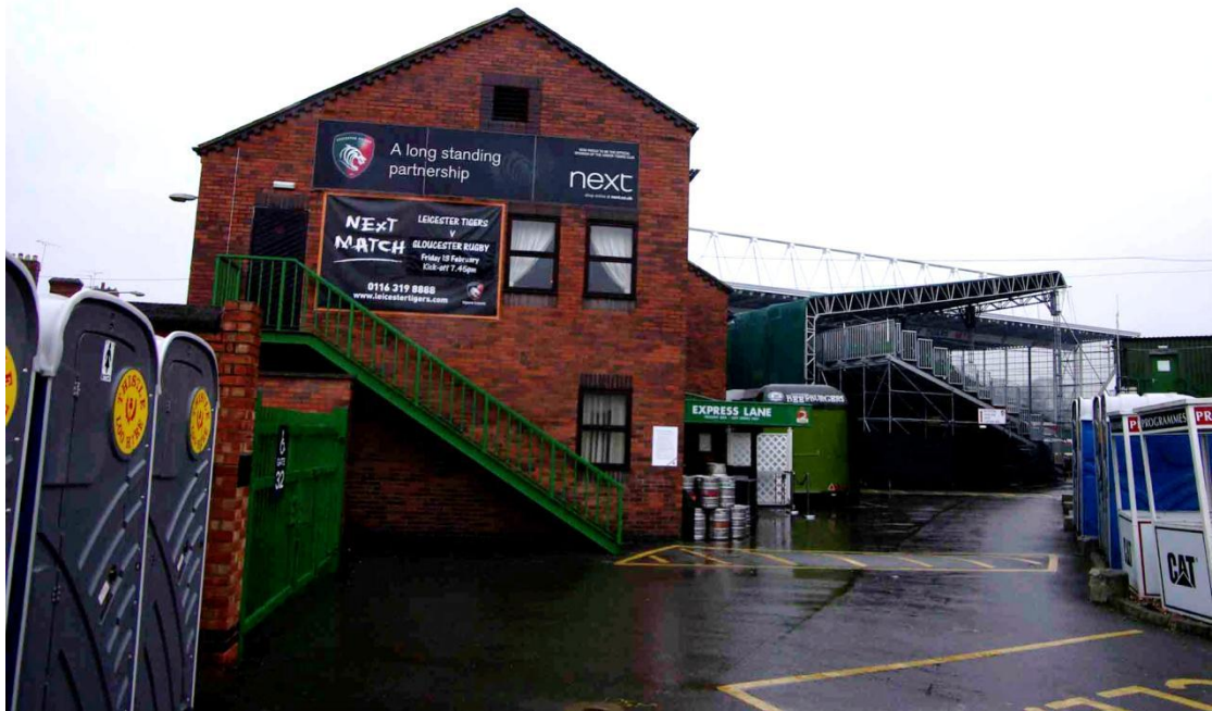
Figure 11 South facing elevation Looking north-east. Temporary stand between the Clubhouse and the pitch is on the right of the picture
