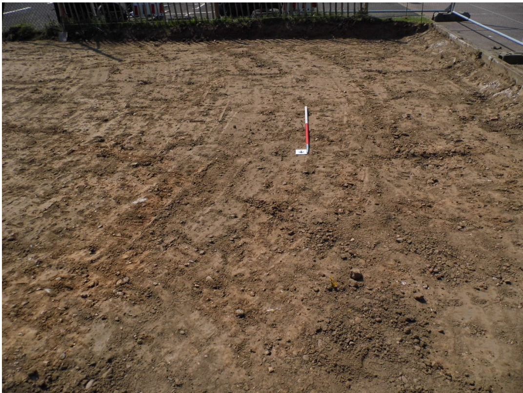
Figure 4 Stripped surface of west side of the area looking south
