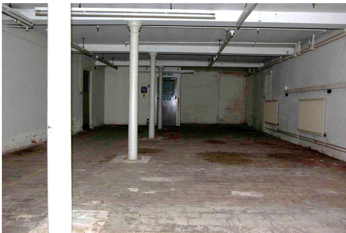
Figure 22 South range basement Looking south east. 1m scale
