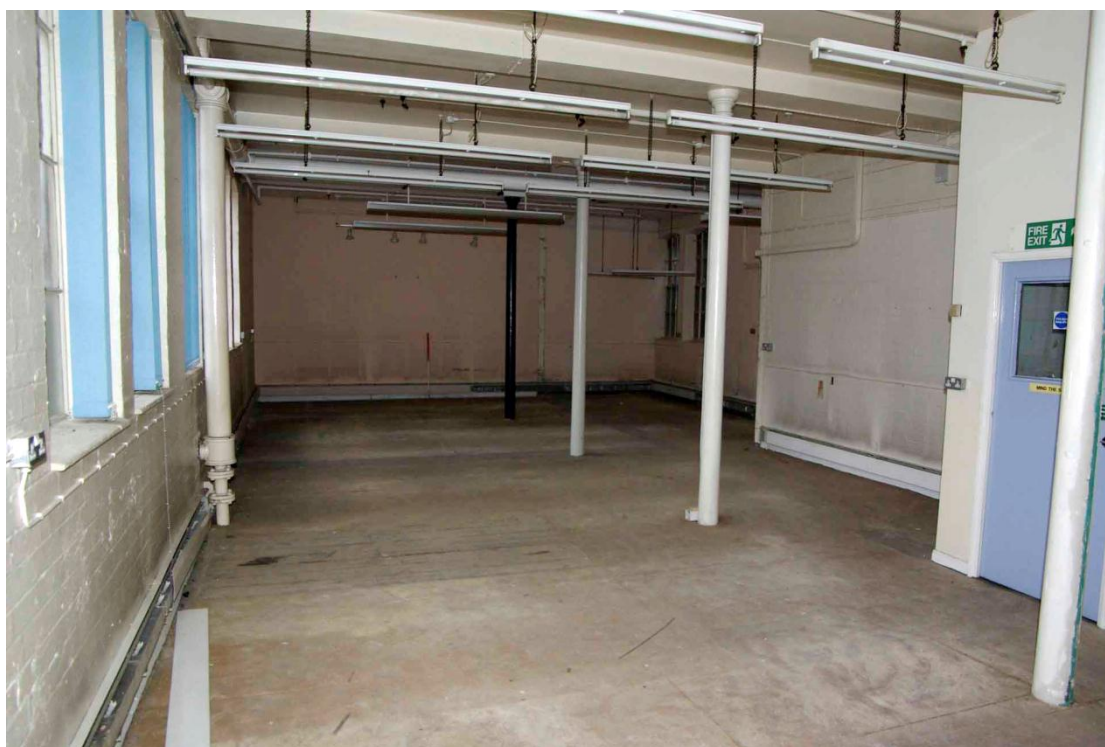
Figure 33 Ground floor south range Looking north west. 1m scale
