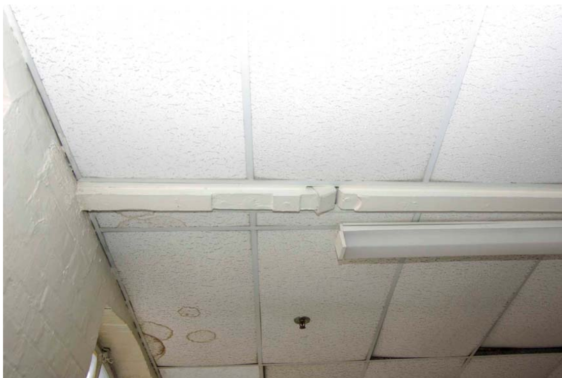
Figure 44 Front range roof detail, easternmost office
