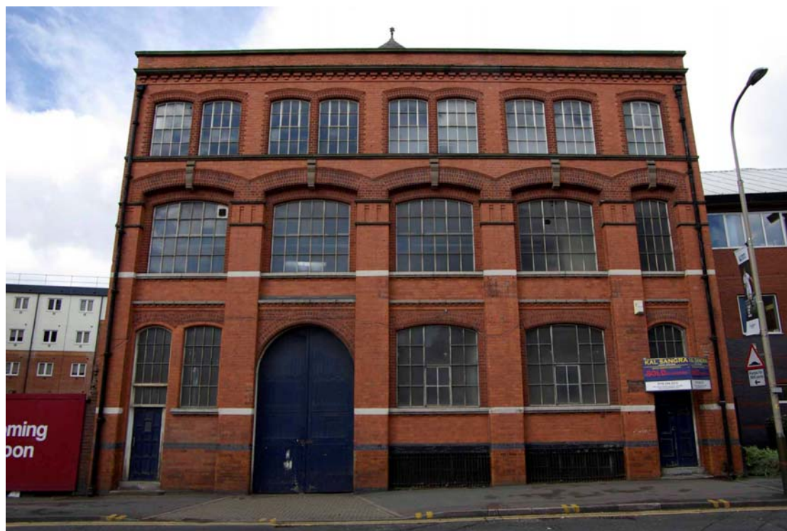
Figure 3 North-east facing elevation onto Oxford Street Looking south-west
