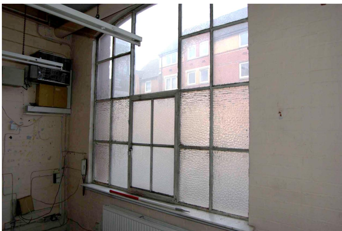
Figure 29 Front range window detail Looking north. 1m scale
