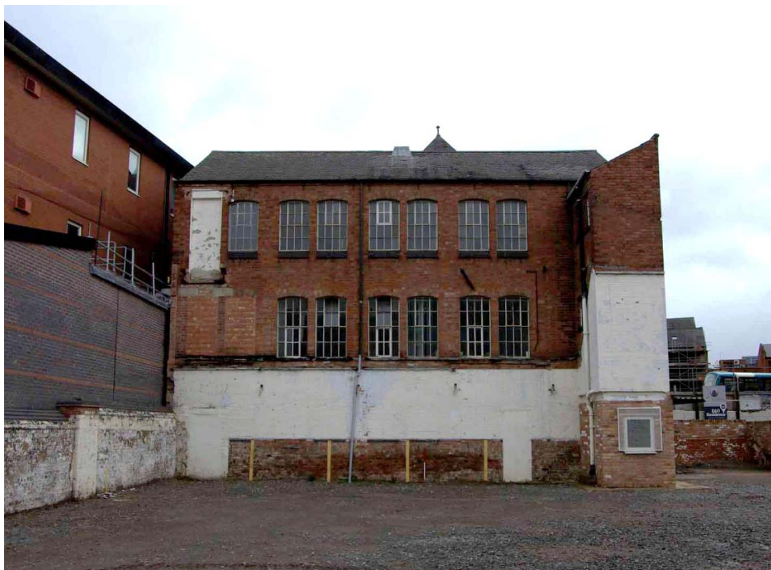
Figure 14 South-west facing elevation Looking north-east
