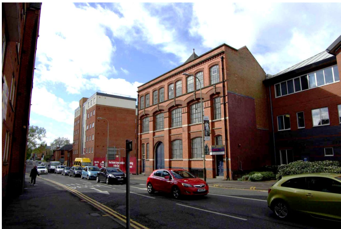
Figure 5 North east and north-west facing elevations Looking south east
