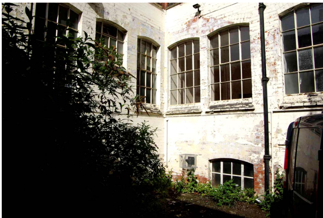
Figure 50 Courtyard, junction of cross and south ranges Looking west
