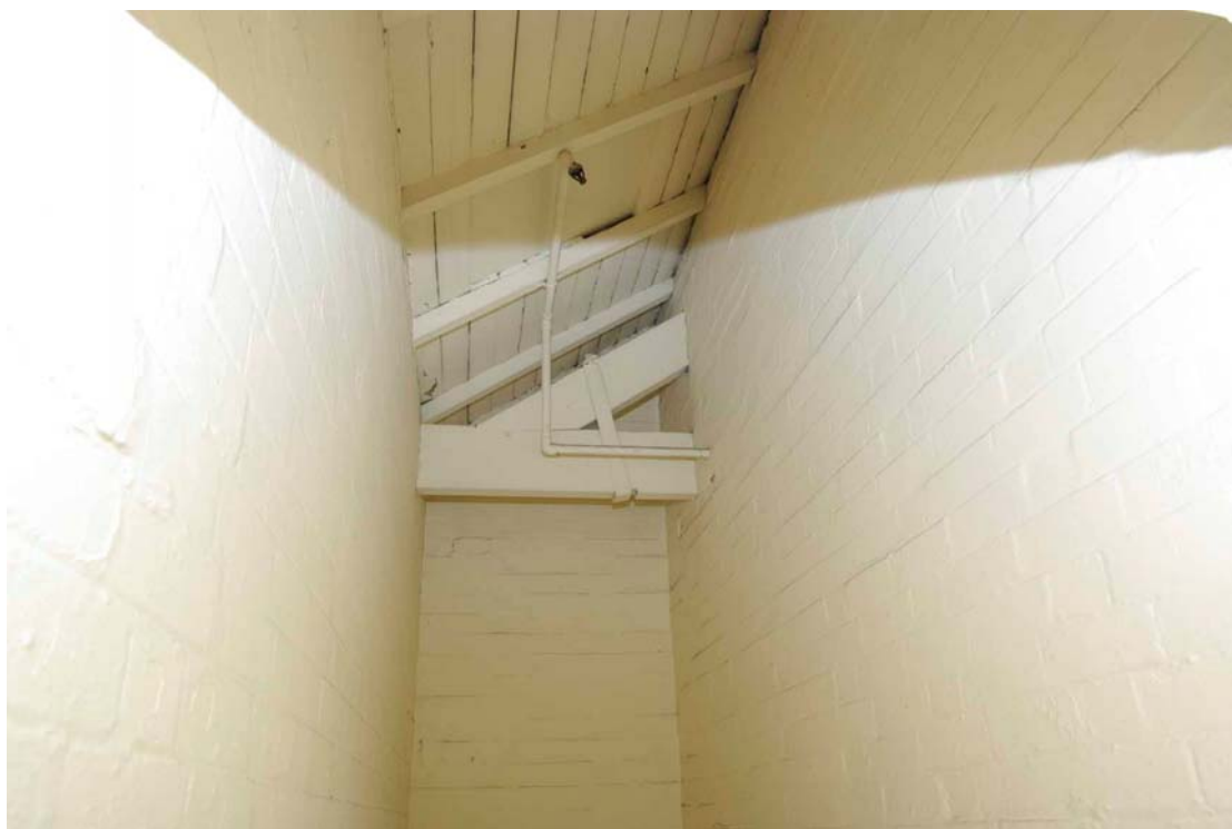
Figure 41 South range roof detail Looking south east over stairwell
