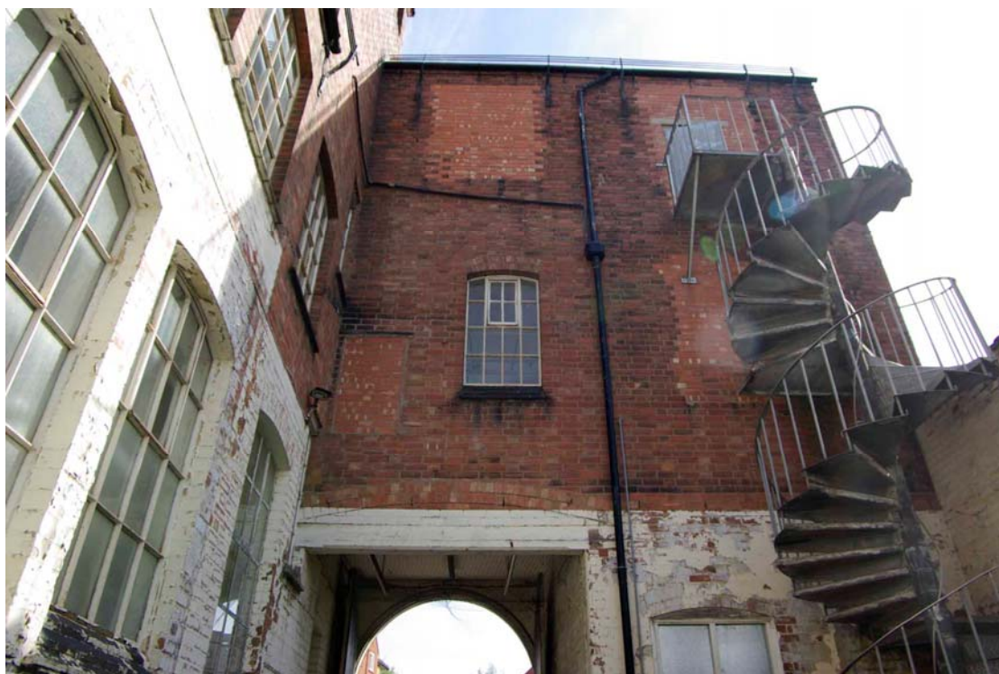
Figure 52 Courtyard, rear of front range Looking north east
