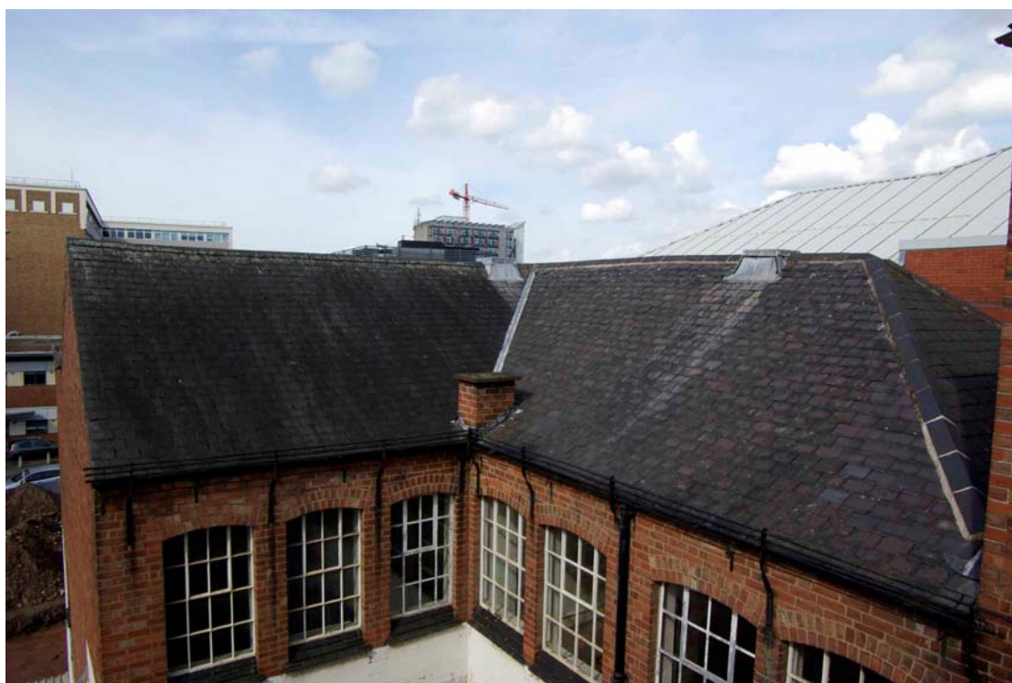
Figure 47 External roof detail of cross and south ranges Looking south-west
