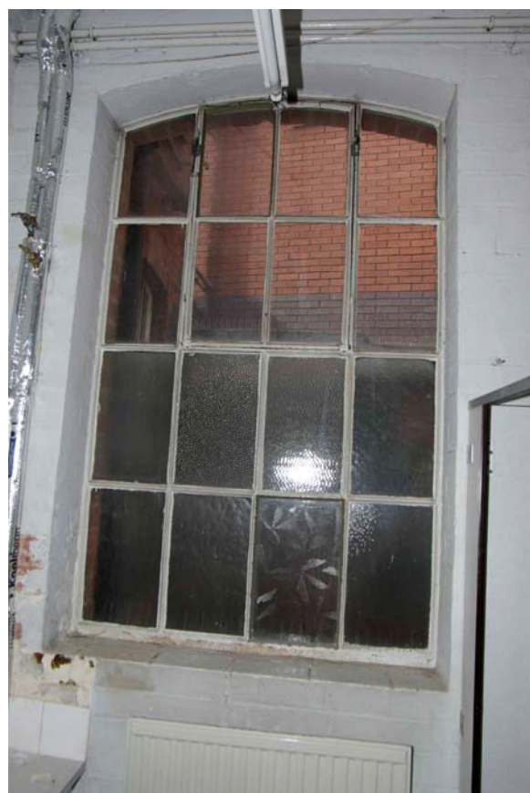
Figure 31 Cross range window detail Looking west
