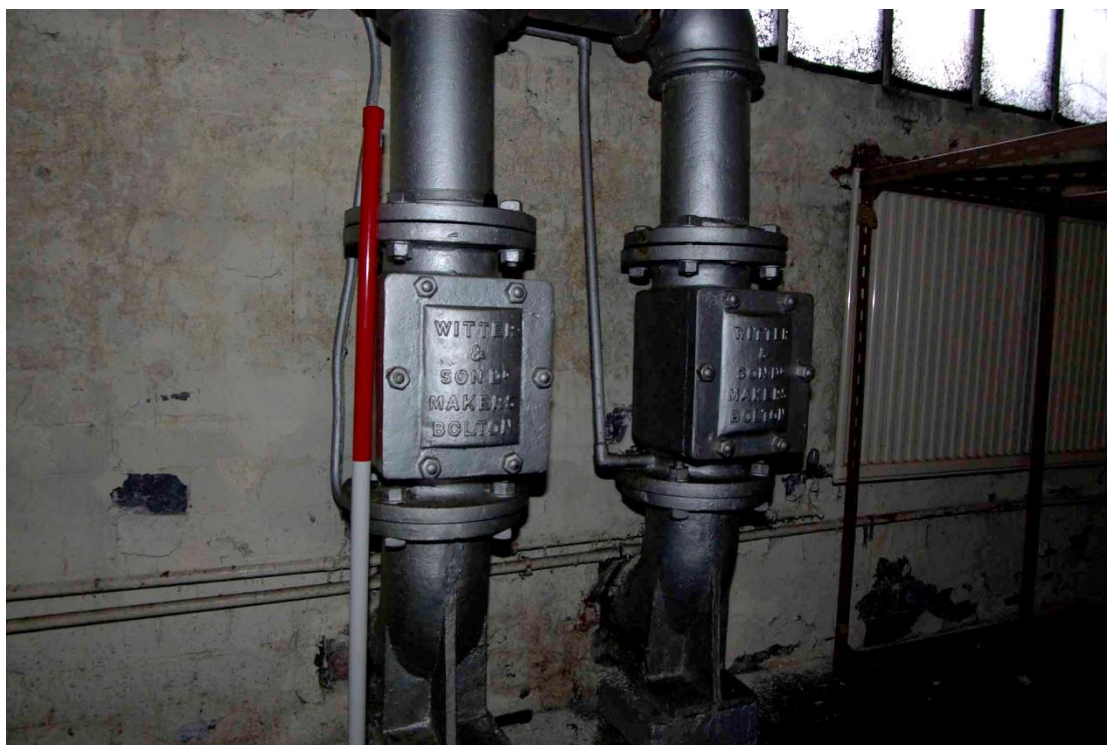
Figure 19 Heating apparatus, front range basement Looking north east. 1m scale
