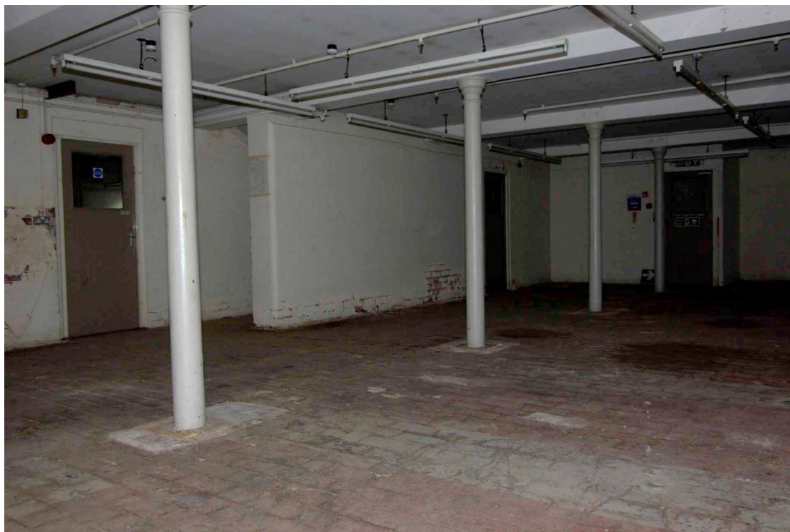
Figure 21 South range basement Looking east
