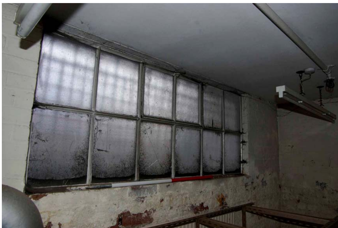
Figure 18 Front basement window Looking north-east. 1m scale
