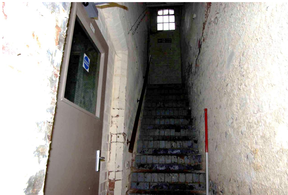
Figure 16 Main stairs to basement Looking south west. 1m scale
