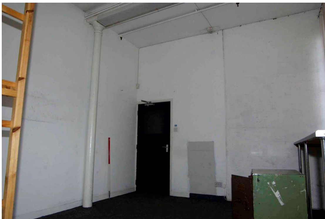
Figure 30 Office in cross range with column Looking north. 1m scale
