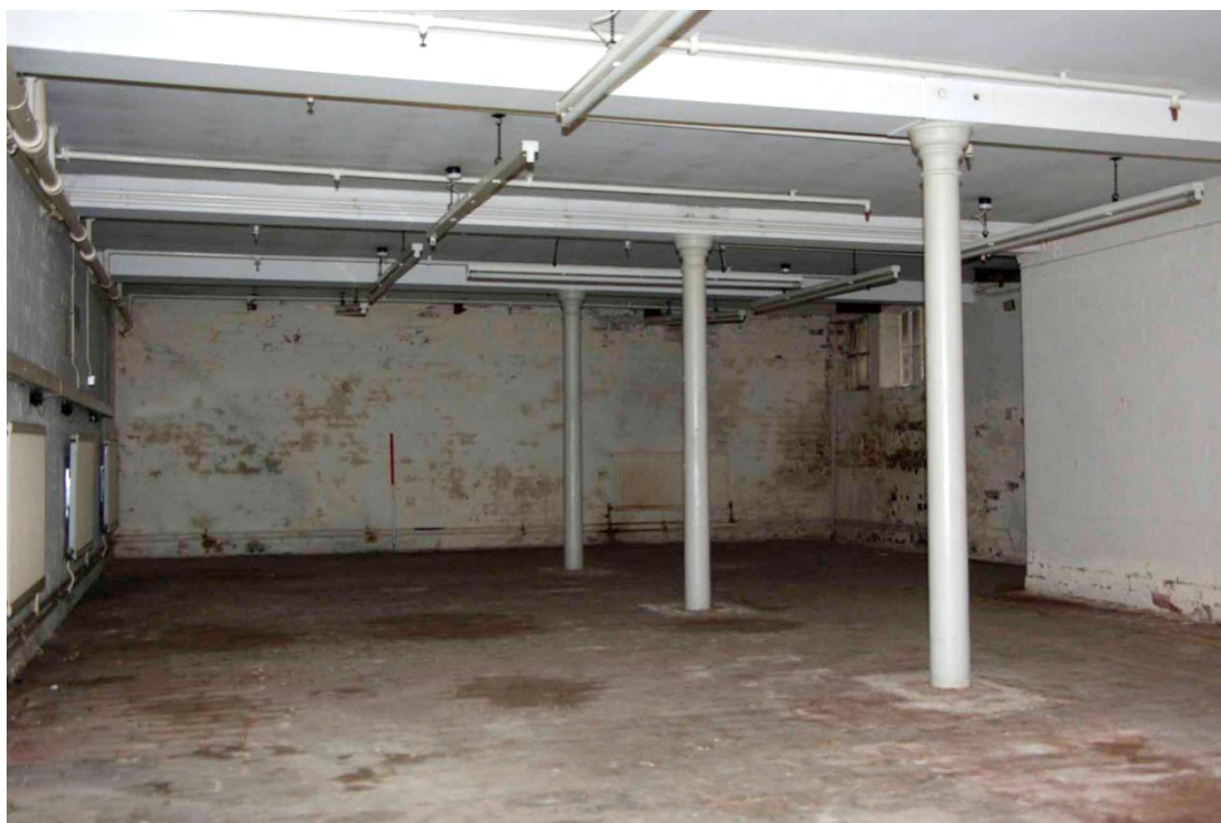
Figure 23 South range basement Looking north west. 1m scale
