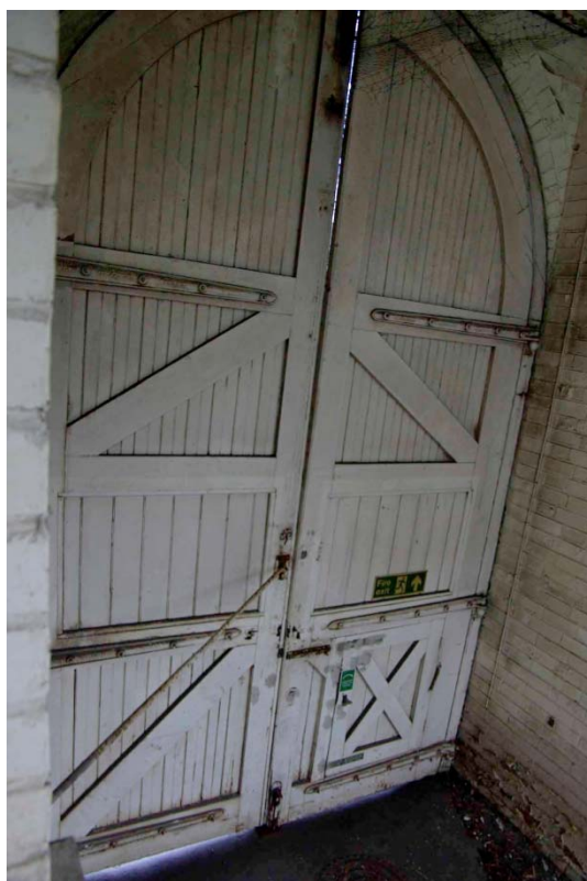
Figure 48 Inside view of courtyard doors Looking north-east
