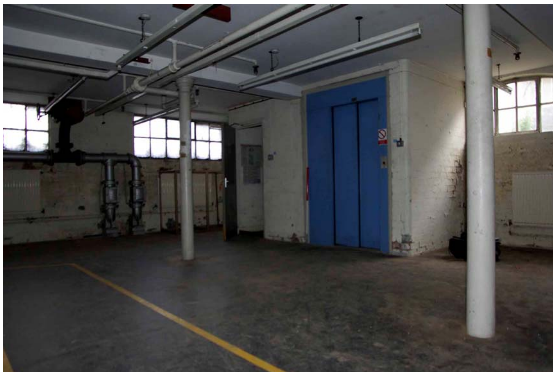
Figure 17 Front range basement Looking north east
