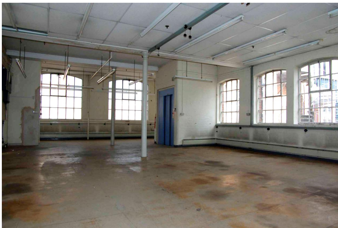
Figure 37 First floor front and cross range Looking north east
