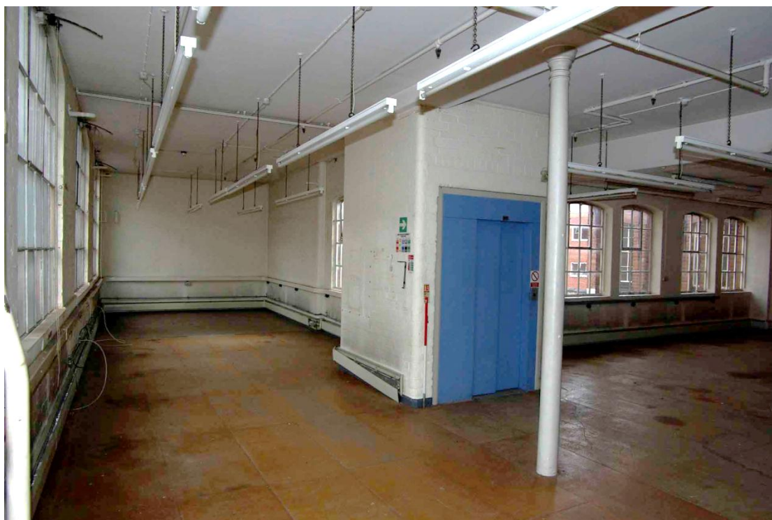
Figure 35 First floor front range Looking south east. 1m scale
