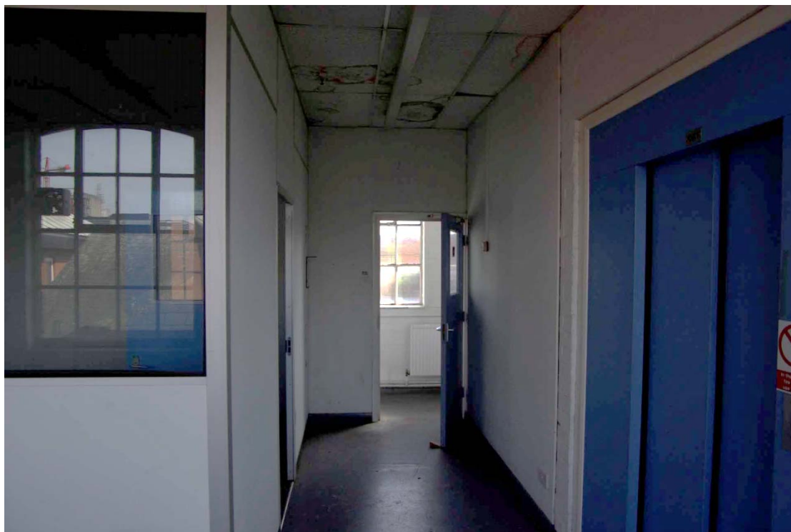
Figure 46 Front range offices and lift Looking north-east
