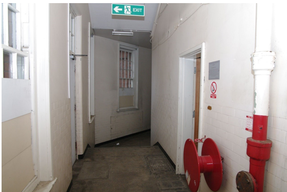
Figure 29 Zone 2 ground floor photo 26 corridor with glazed brick walling
