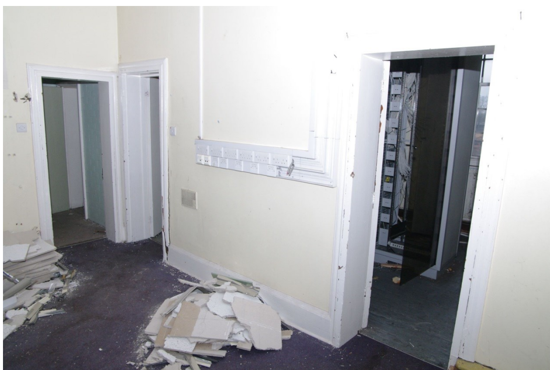
Figure 31 Zone 2 first floor photo 28 skirting boards and door surrounds
