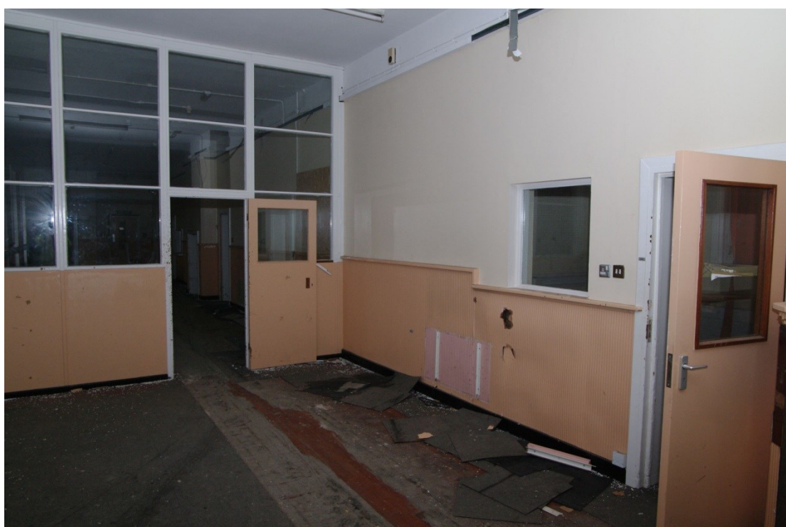
Figure 27 Zone 2 ground floor photo 24 day room possible panelling behind later sheeting
