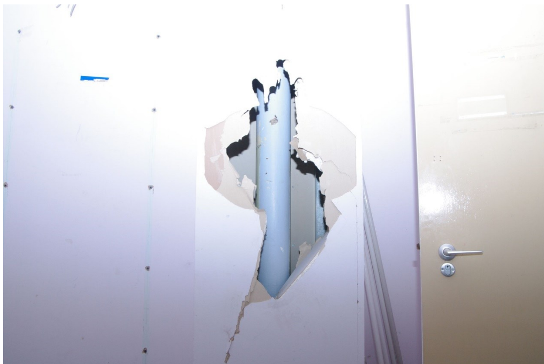
Figure 19 Zone 1 first floor photo 17 cast iron column
