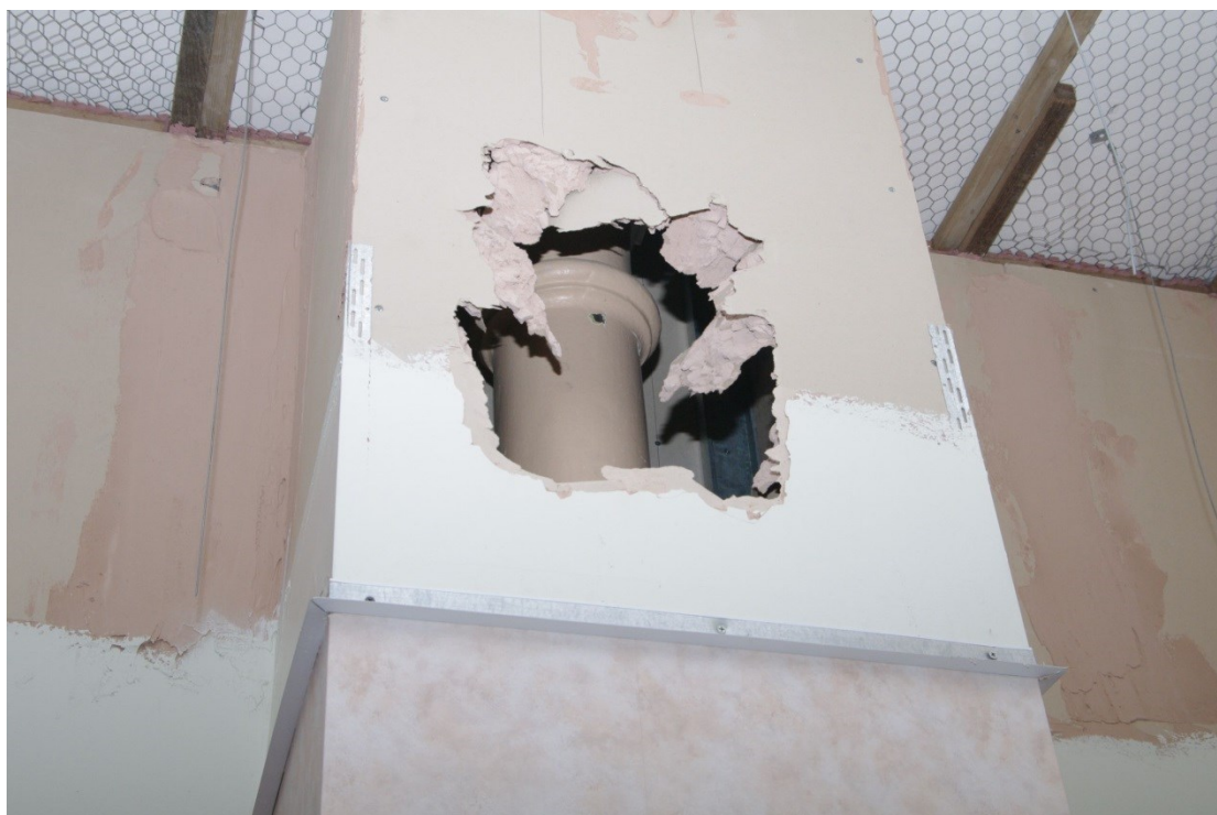
Figure 9 Zone 1 ground floor photo 7 head of cast iron column
