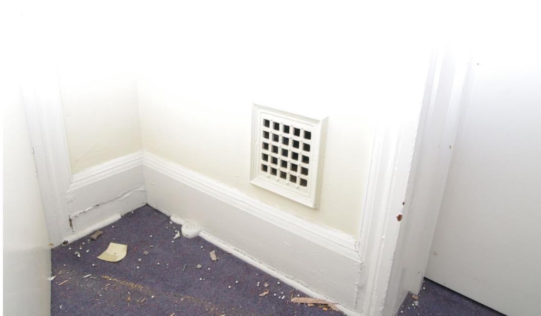
Figure 38 Zone 2 first floor photo 35 cell corridor vent
