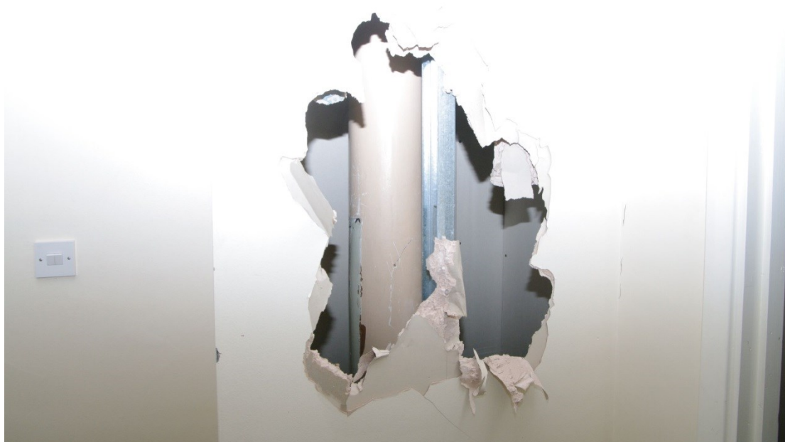
Figure 8 Zone 1 ground floor photo 6 cast iron column
