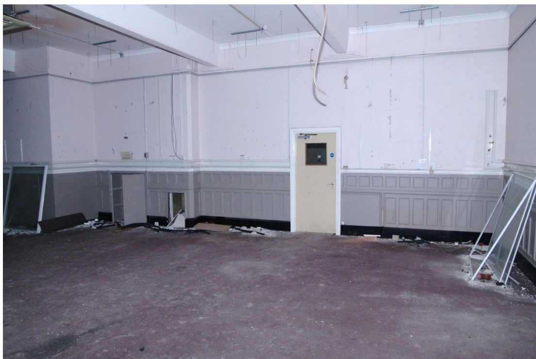
Figure 21 Zone 1 first floor photo 19 day room panelling
