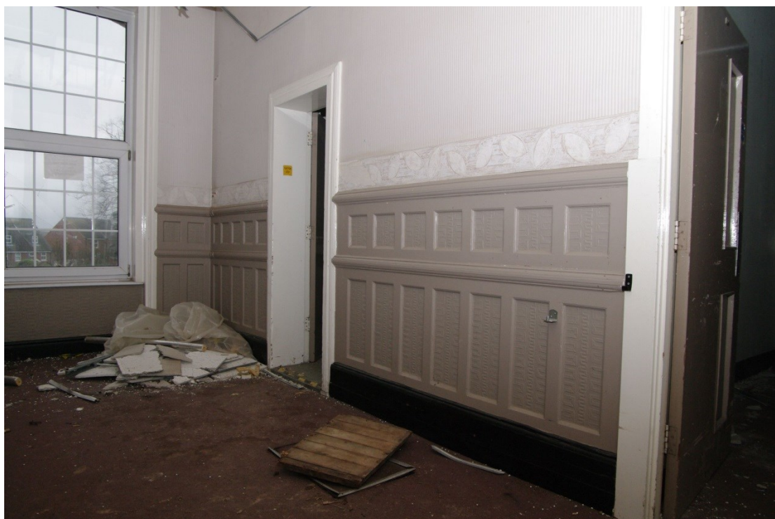
Figure 13 Zone 1 ground floor photo 11 day room panelling
