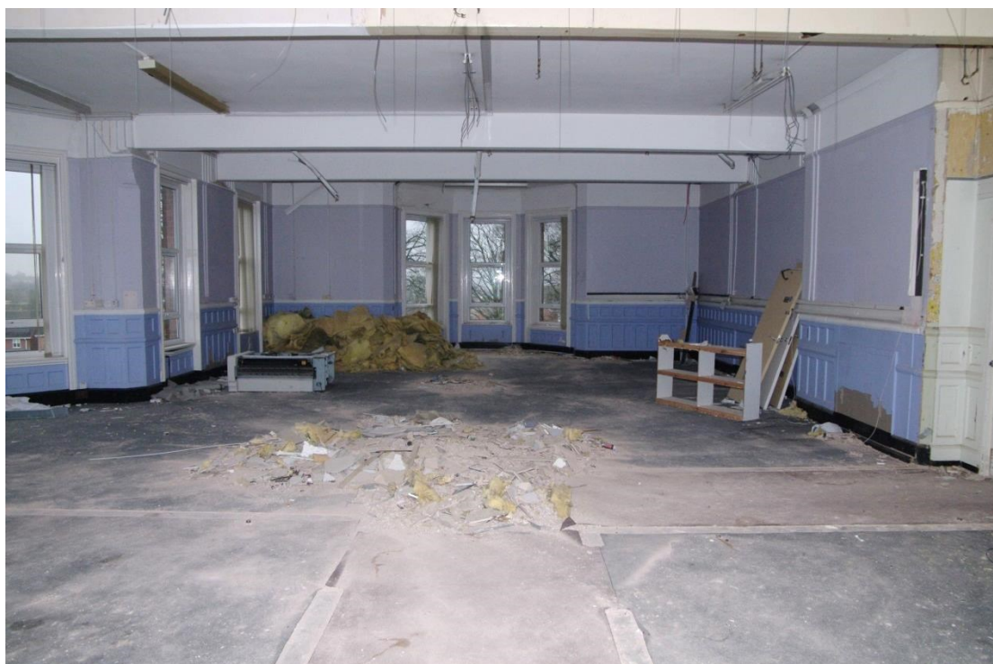
Figure 16 Zone 1 first floor photo 14 day room panelling
