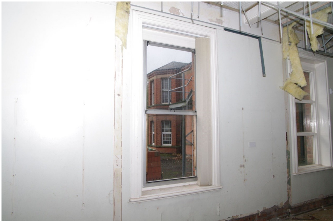
Figure 6 Zone 1 ground floor photo 4 moulded window surrounds
