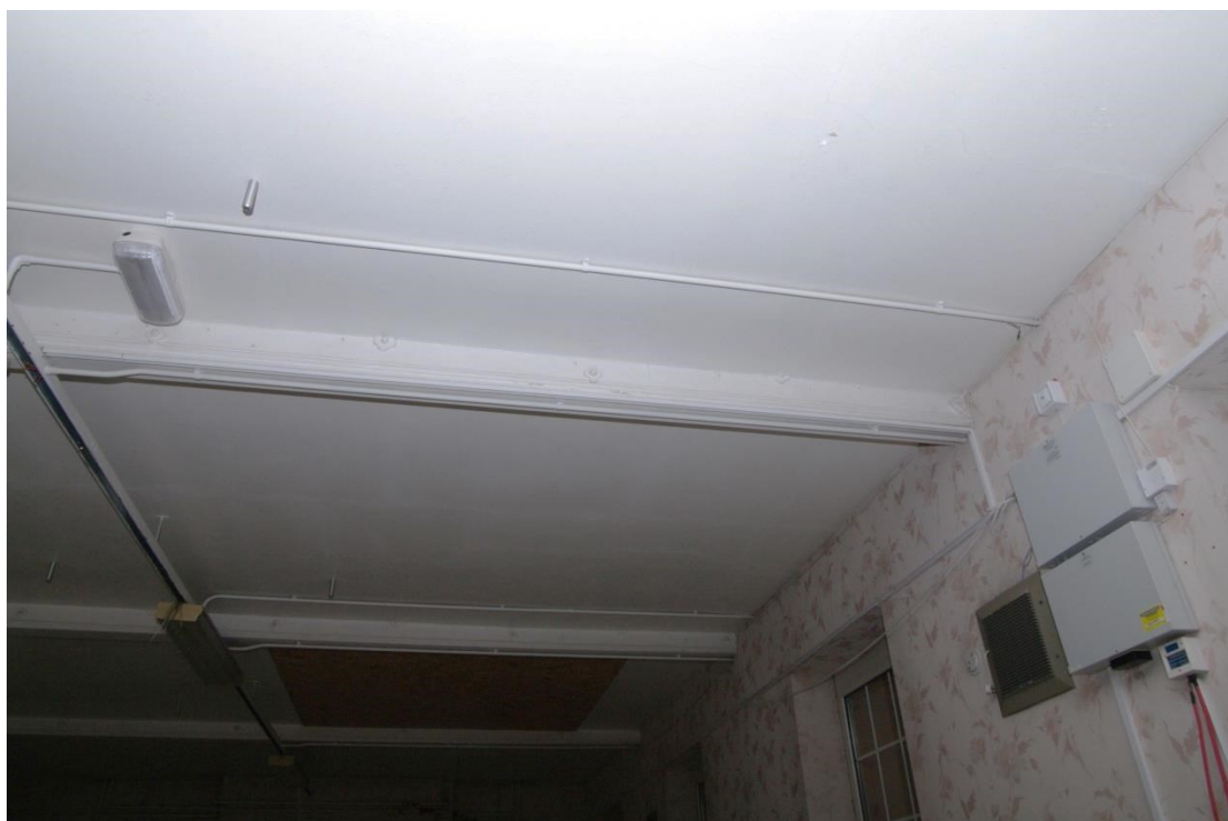
Figure 41 Zone 3 ground floor photo 37 ceiling joists
