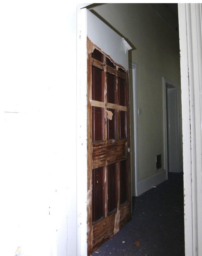
Figure 36 Zone 2 first floor photo 33 panelled door with modern covering removed
