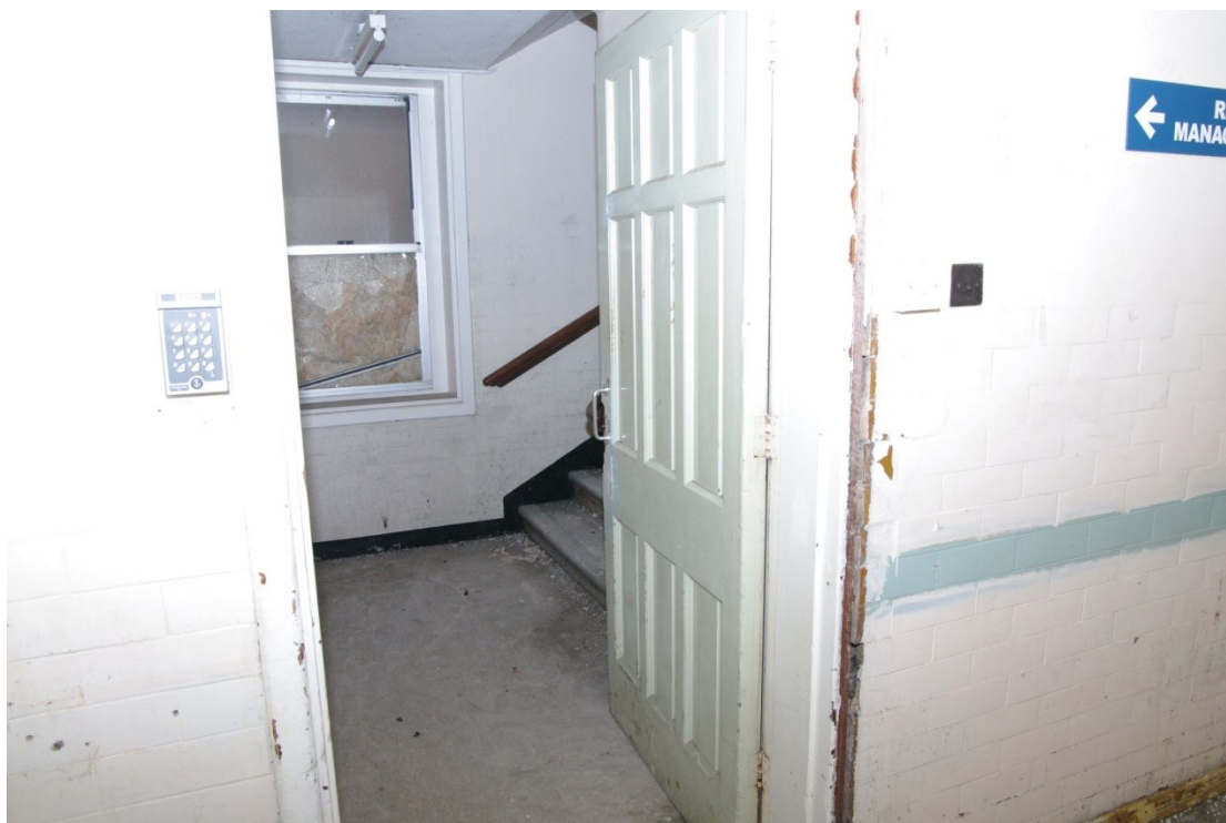
Figure 3 Zone 1 ground floor photo 1. Panelled door
