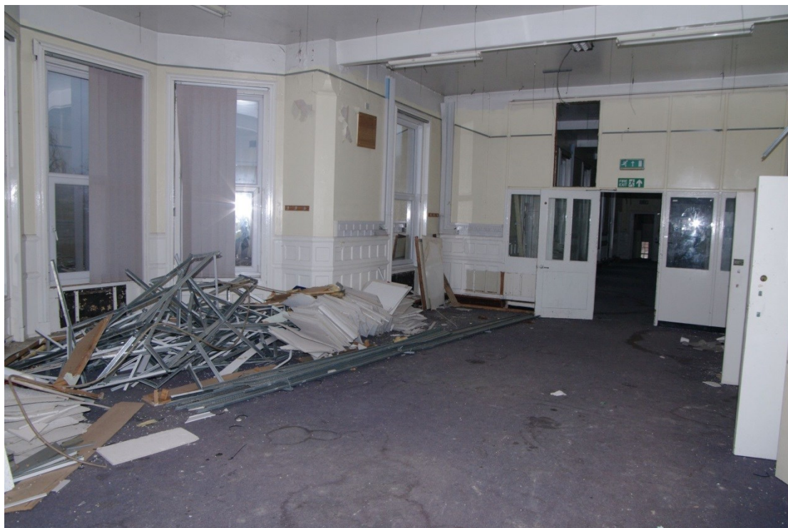
Figure 32 Zone 2 first floor photo 29 day room panelling
