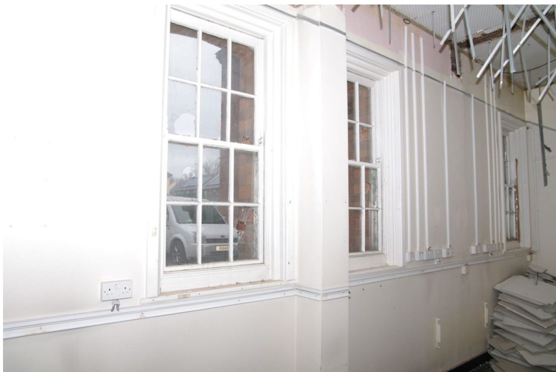
Figure 7 Zone 1 ground floor photo 5 sash windows
