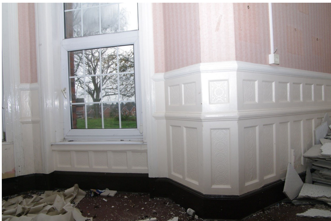
Figure 11 Zone 1 ground floor photo 9 day room panelling
