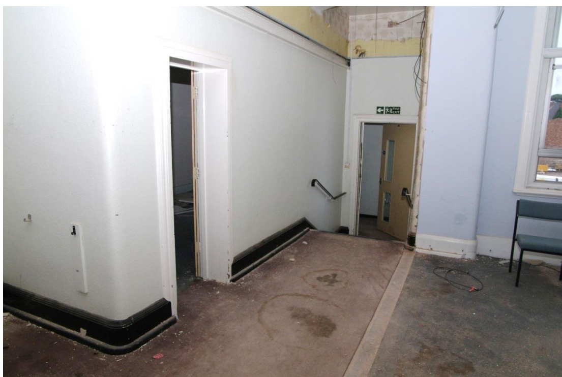
Figure 18 Zone 1 first floor photo 16 moulded door jambs and skirting
