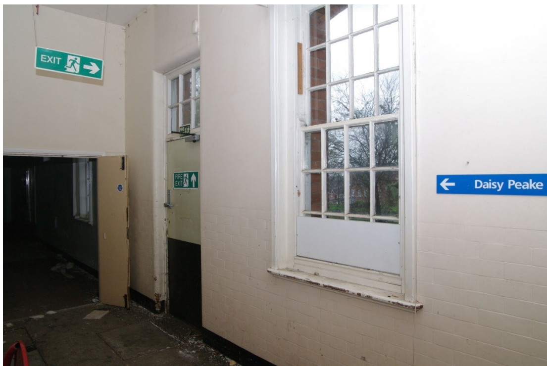
Figure 15 Zone 1 ground floor photo 13 boarded panelled door and sash window
