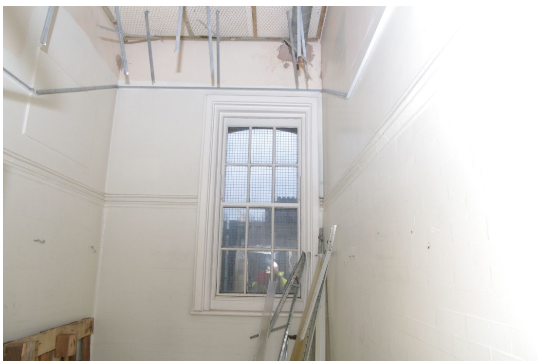
Figure 14 Zone 1 ground floor photo 12 sash window and glazed bricks of an individual cell
