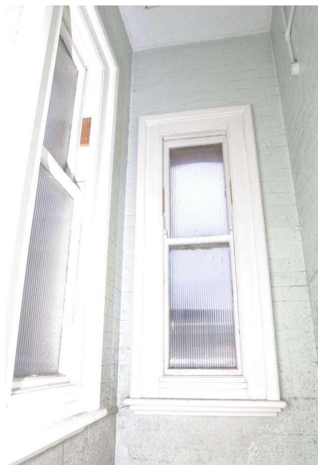
Figure 25 Zone 2 ground floor photo 22 toilet block windows
