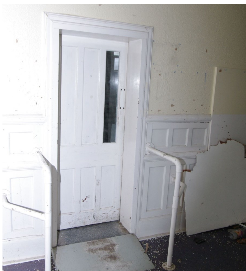
Figure 35 Zone 2 first floor photo 32 panelled cell door
