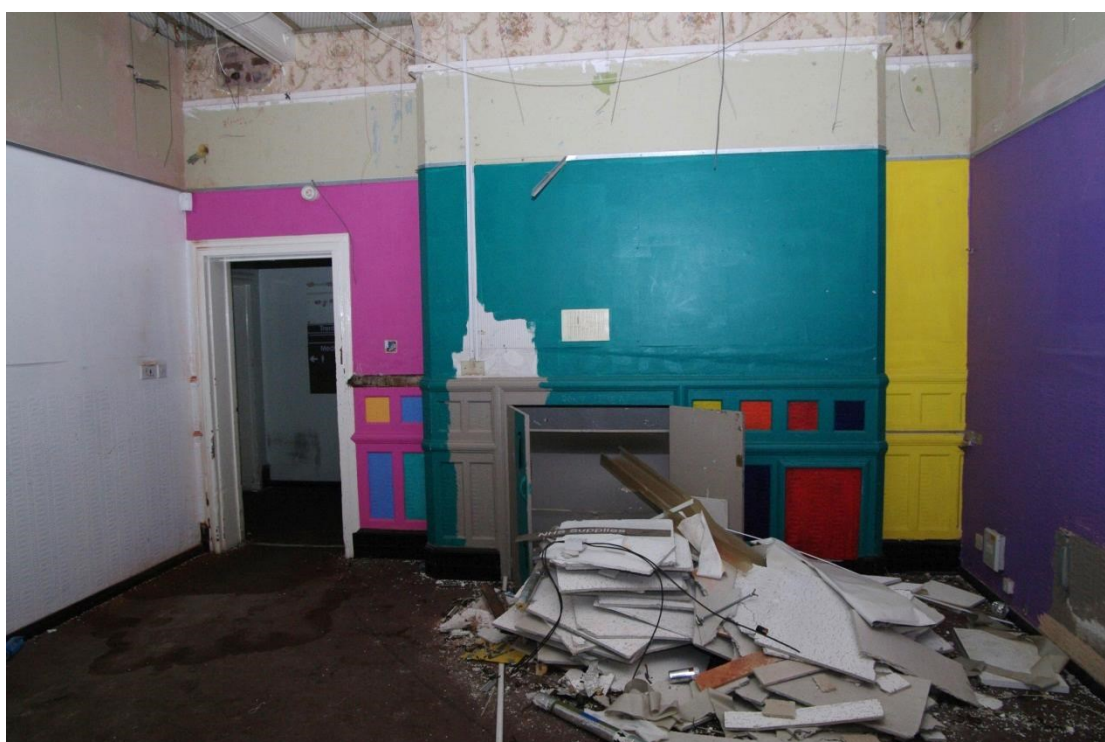
Figure 12 Zone 1 ground floor photo 10 day room panelling
