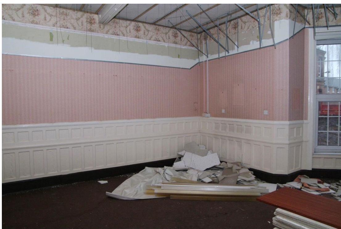
Figure 10 Zone 1 ground floor photo 8 day room panelling
