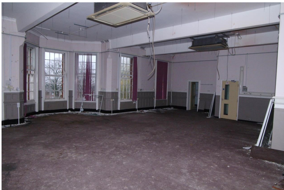
Figure 20 Zone 1 first floor photo 18 day room panelling
