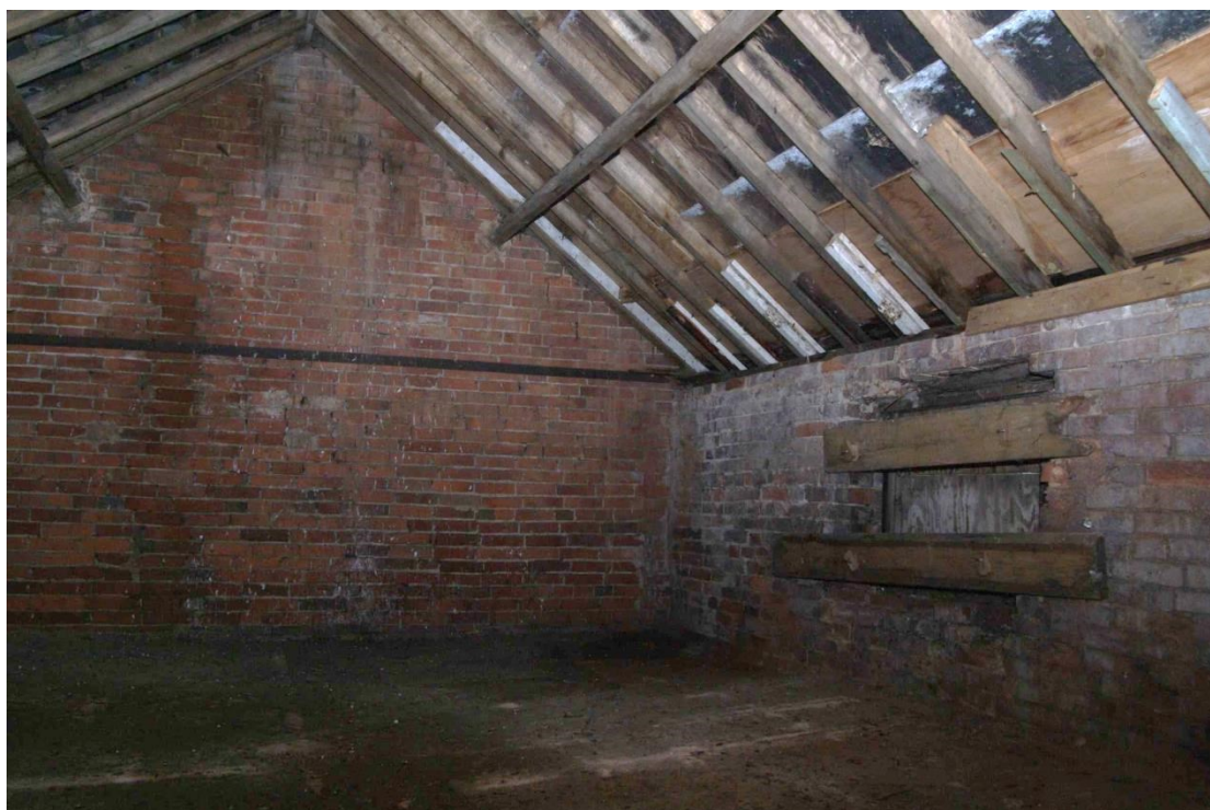
Figure 19 Barn, first floor Looking south-west
