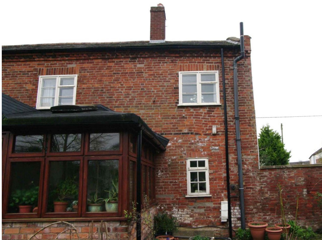
Figure 23 Farmhouse, west facing elevation Looking east towards southernmost bay
