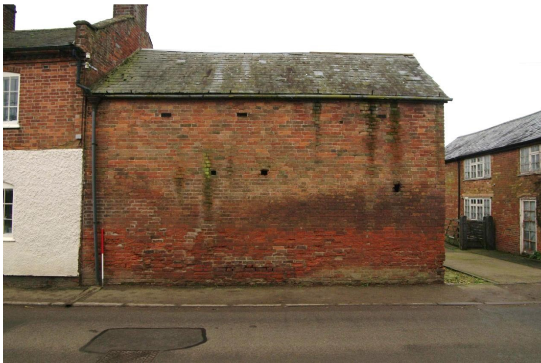
Figure 9 The barn, east facing elevation Looking west. 1m scale
