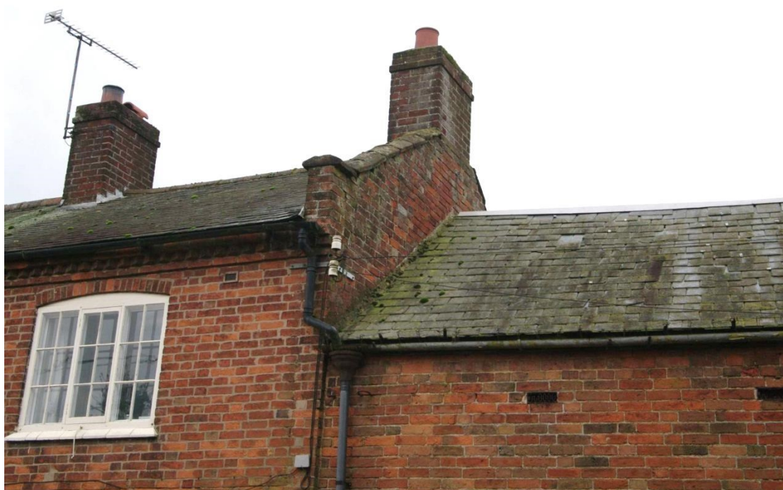
Figure 10 East facing elevation joint between barn and house Looking south-west
