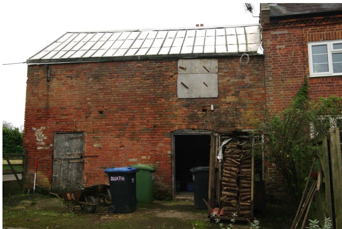
Figure 12 Barn, west facing elevation Looking east. 1m scale
