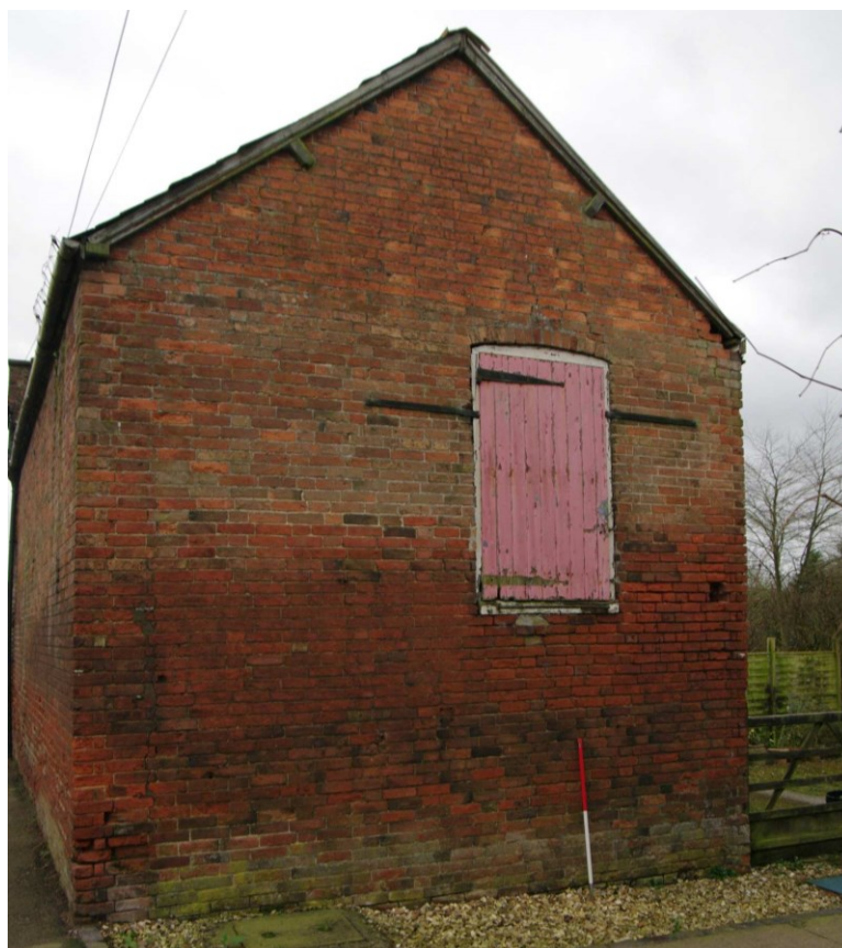
Figure 11 Barn, north facing elevation Looking south-west. 1m scale
