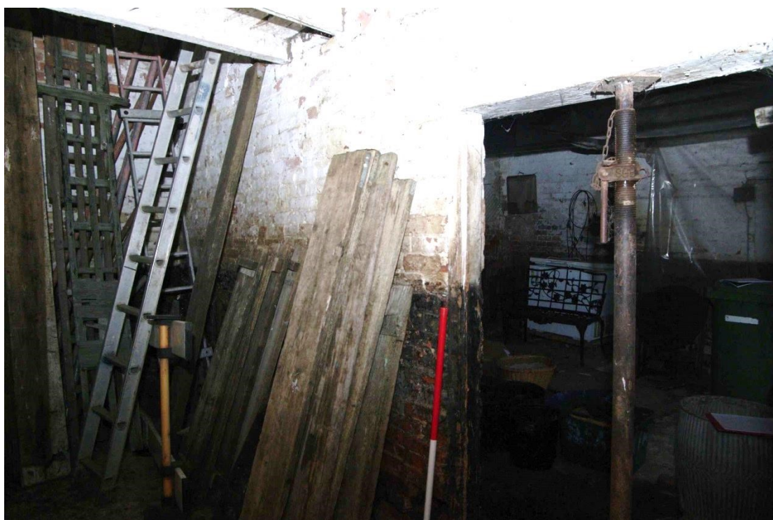
Figure 14 Barn, north room Looking south-east into southern room. 1m scale
