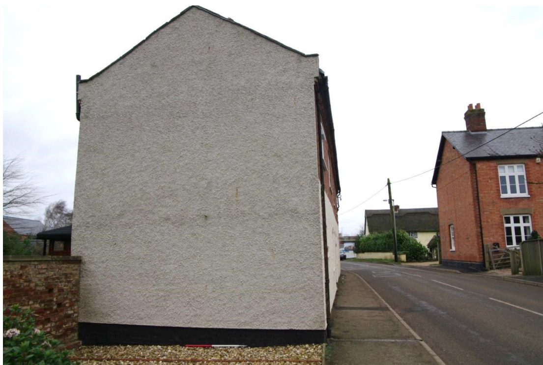
Figure 21 Farmhouse, south facing elevation Looking north. 1m scale
