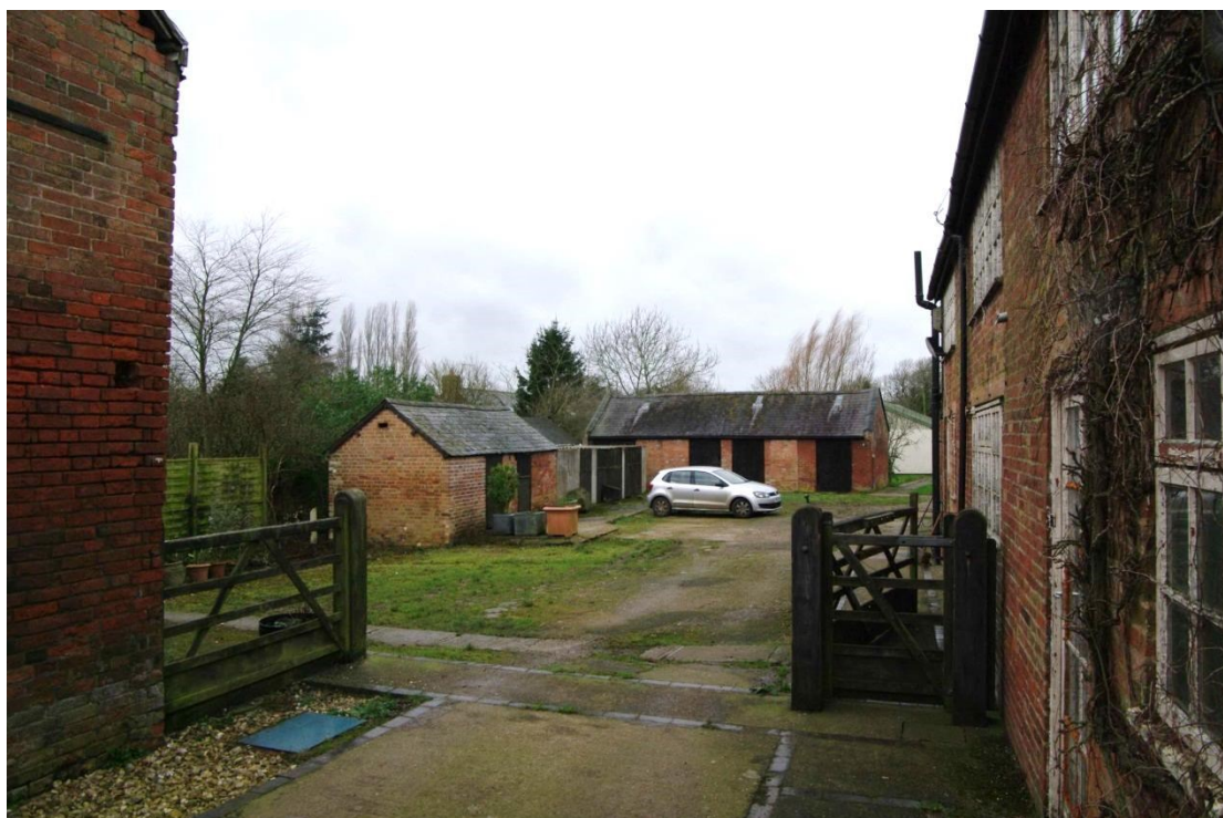
Figure 5 Sleath Farm, yard Looking west. Barn subject to this assessment is on left of photograph
