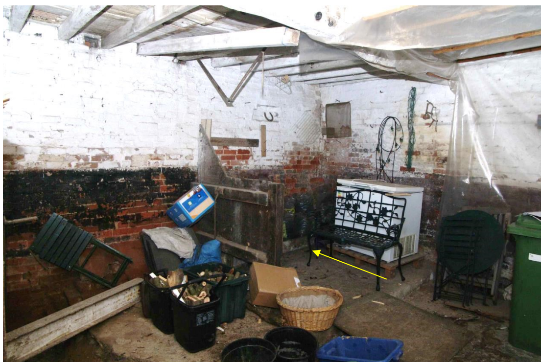
Figure 16 Barn, south room Looking south-east. Animal feed trough arrowed
