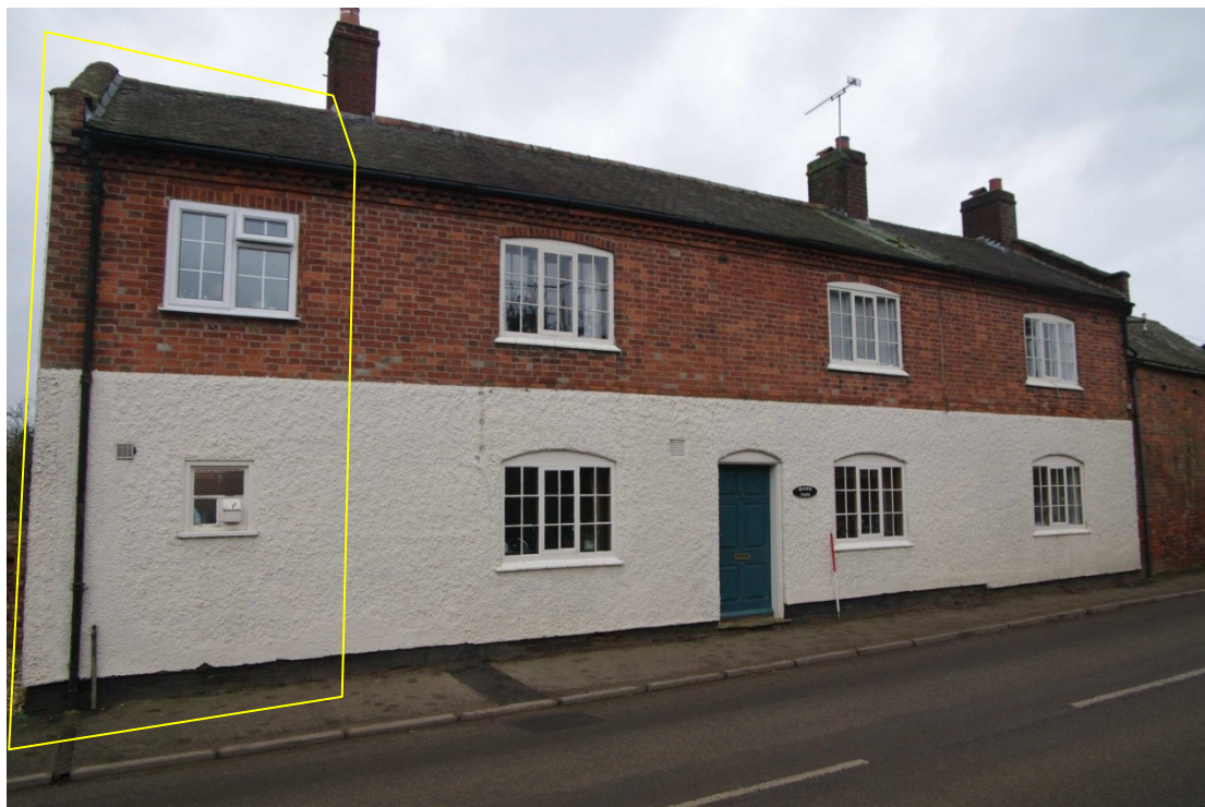
Figure 20 Farmhouse, east facing elevation Looking north-east. 1m scale. Yellow box indicates the portion of the building to be demolished
