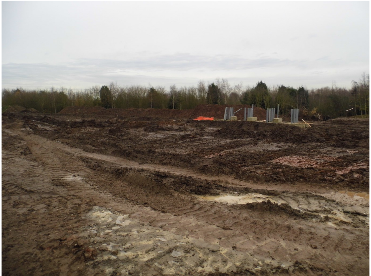
Figure 4 General view of site during groundworks (09.12.2014)
