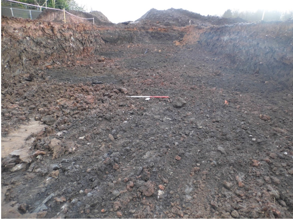
Figure 6 Central part of application area following machine stripping showing modern disturbance (09.12.2014)
