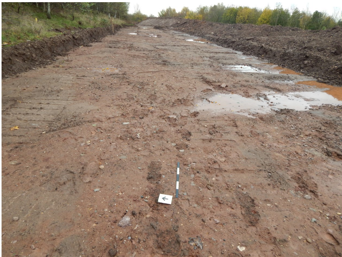
Figure 5. Stripped area to north of development area viewed from the west (19.11.2014)
