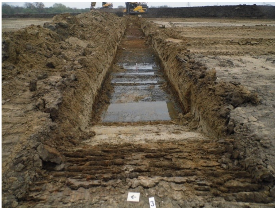
Figure 8: Trench 3 looking east.
