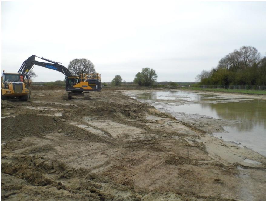
Figure 5: In process of removing glacial deposits, looking south.
