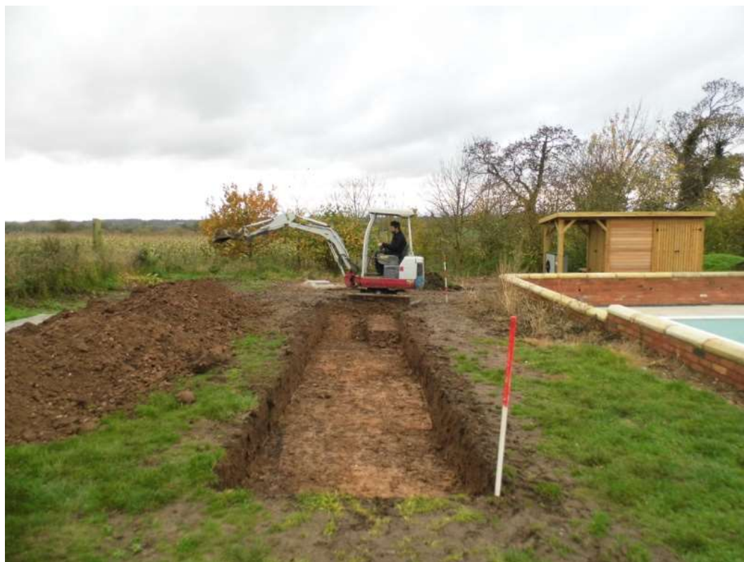
Figure 7: Trench being excavated
