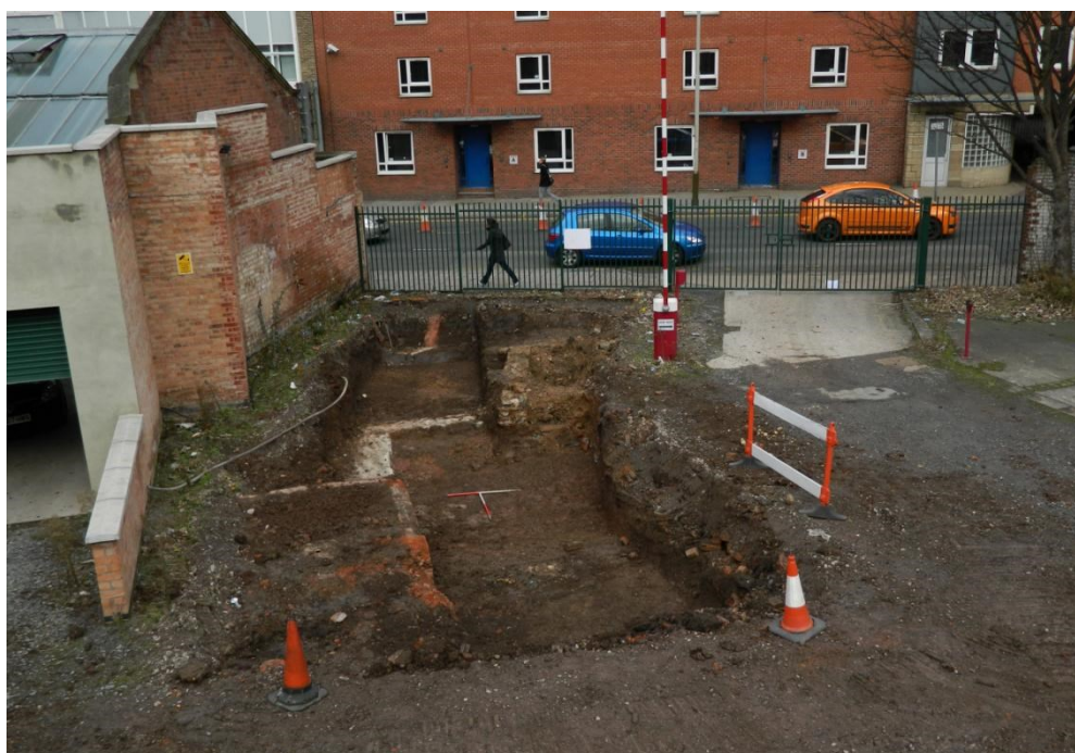
Figure 15: Trench 3 prior to excavation (Newarke Street in the background)
