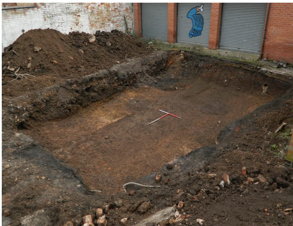
Figure 8: Trench 2 prior to excavation
