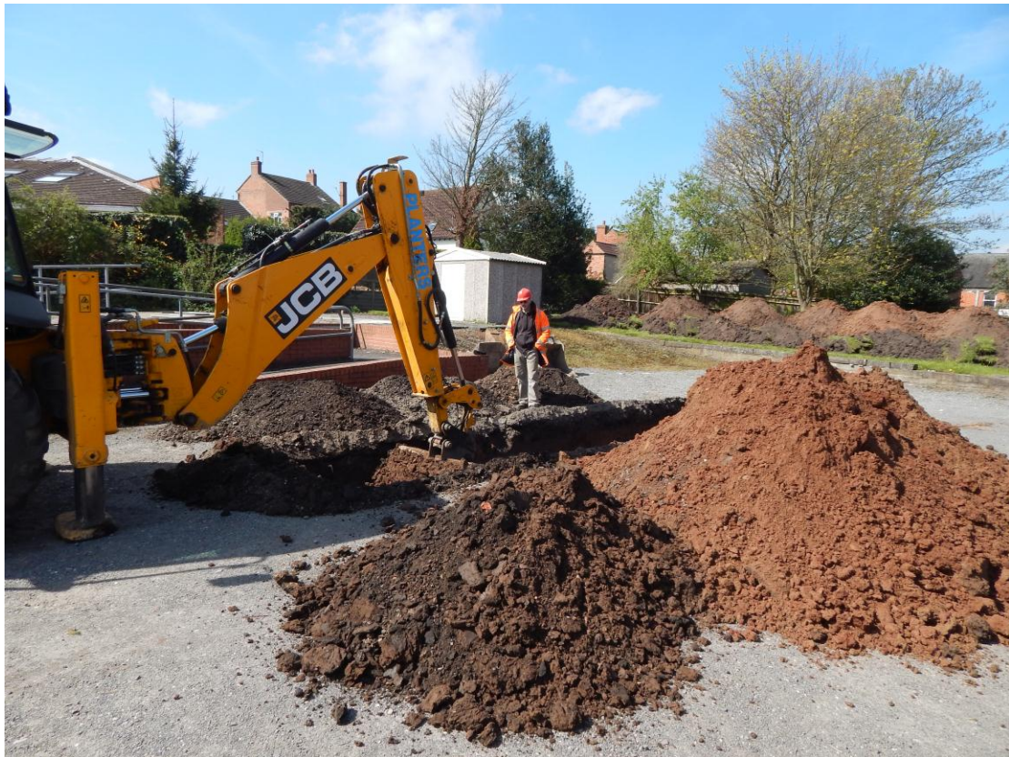
Plate 3: Work in progress on Trench 02, looking south
