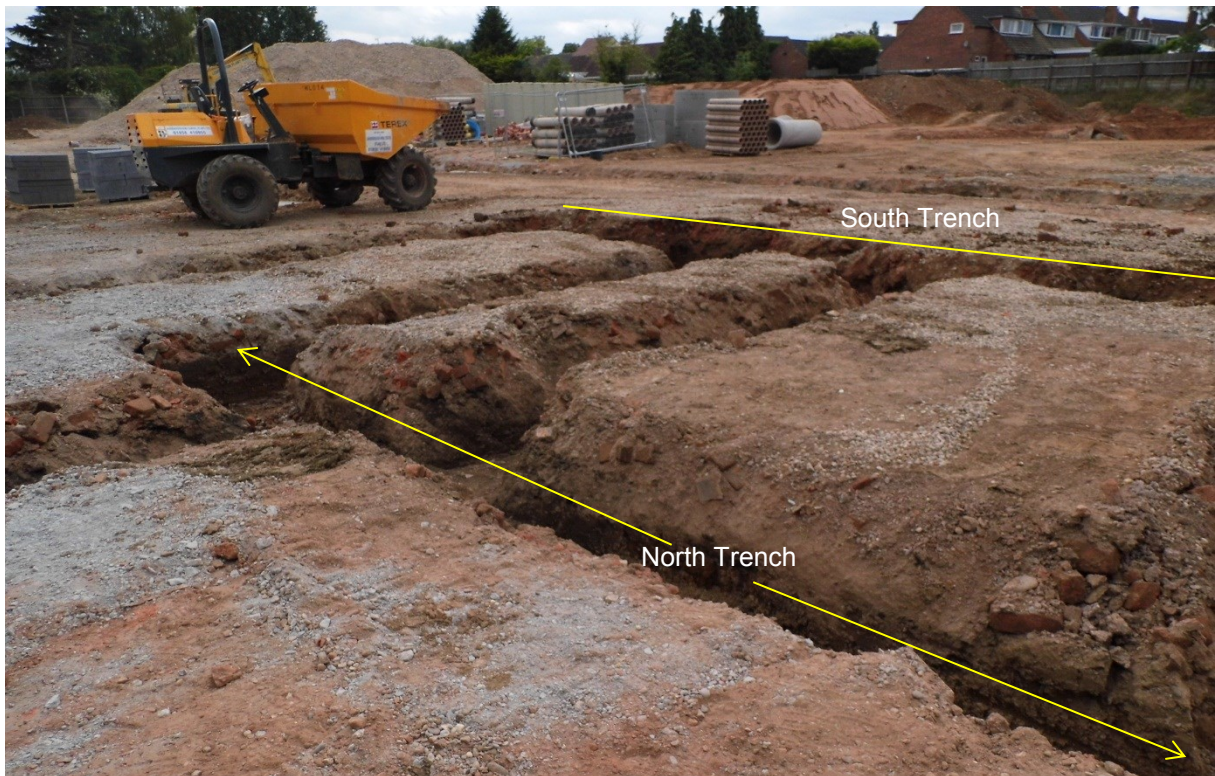
Figure 7. Plot 25 trenching after excavation (facing SE)
