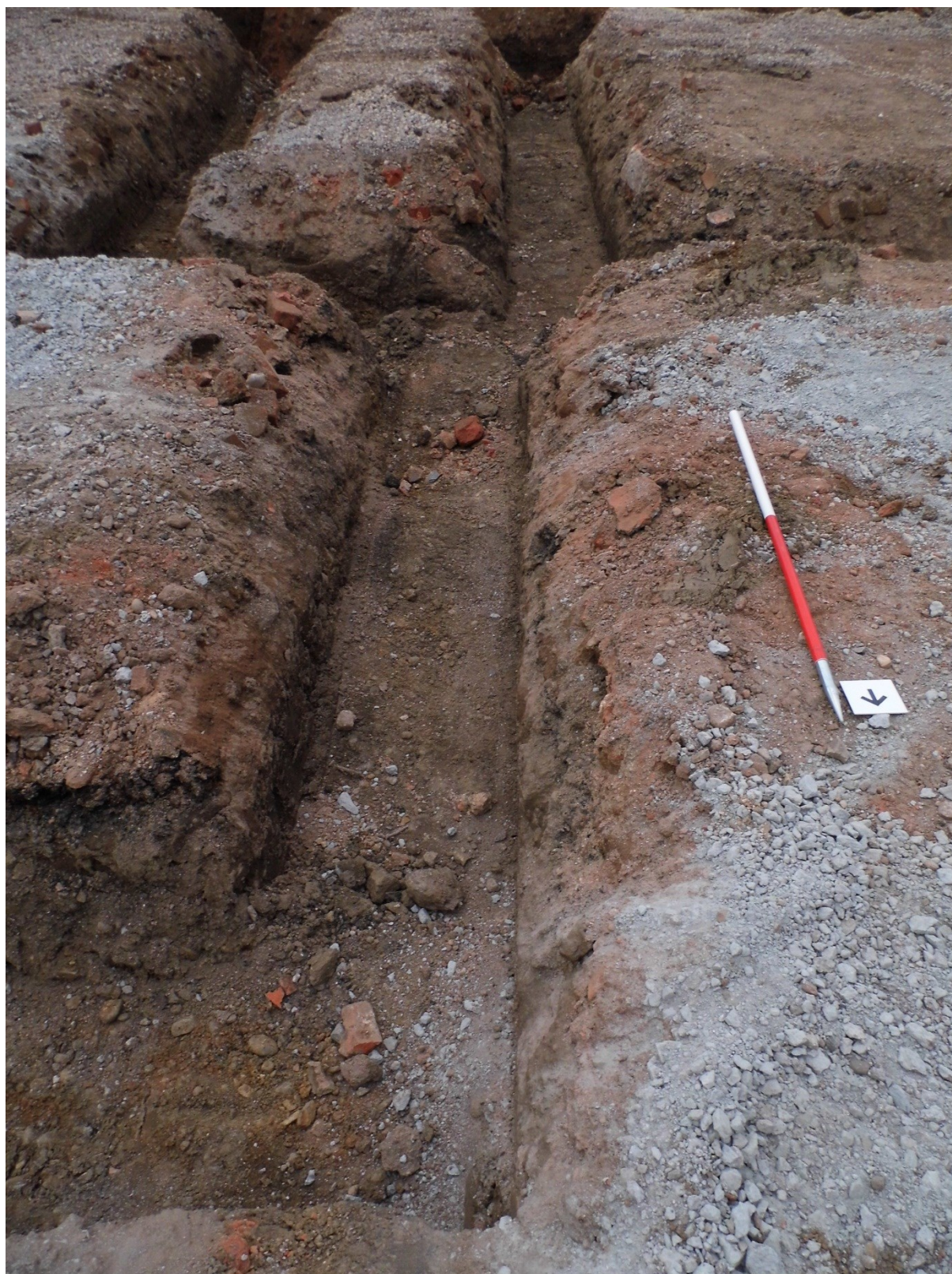
Figure 10. Central area of foundation trench in Plot 25
