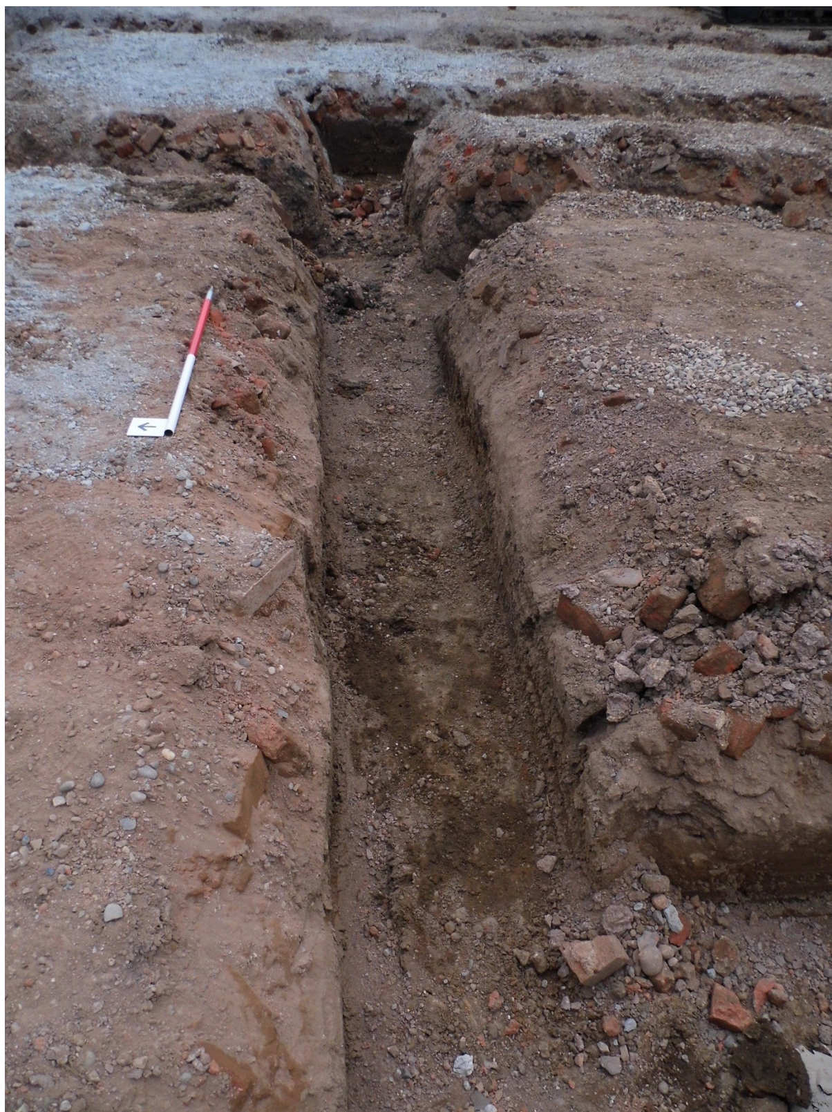
Figure 9. North area of foundation trench in Plot 25
