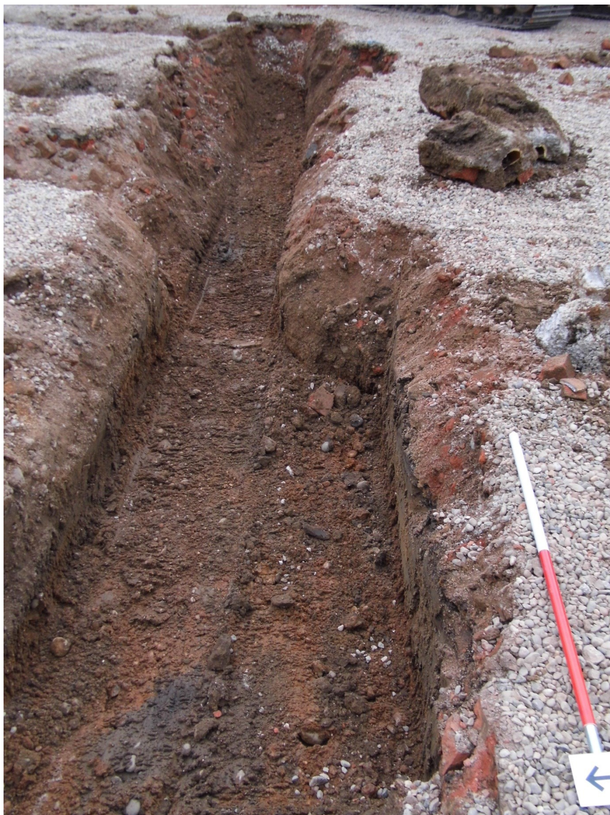
Figure 14 South side of foundation trench in Plot 25
