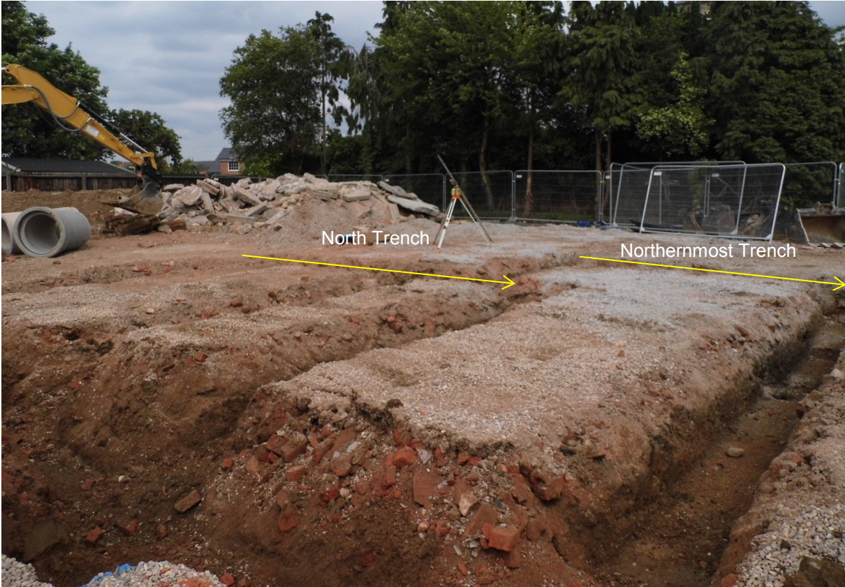
Figure 8. Plot 25 trenching after excavation (facing NW)
