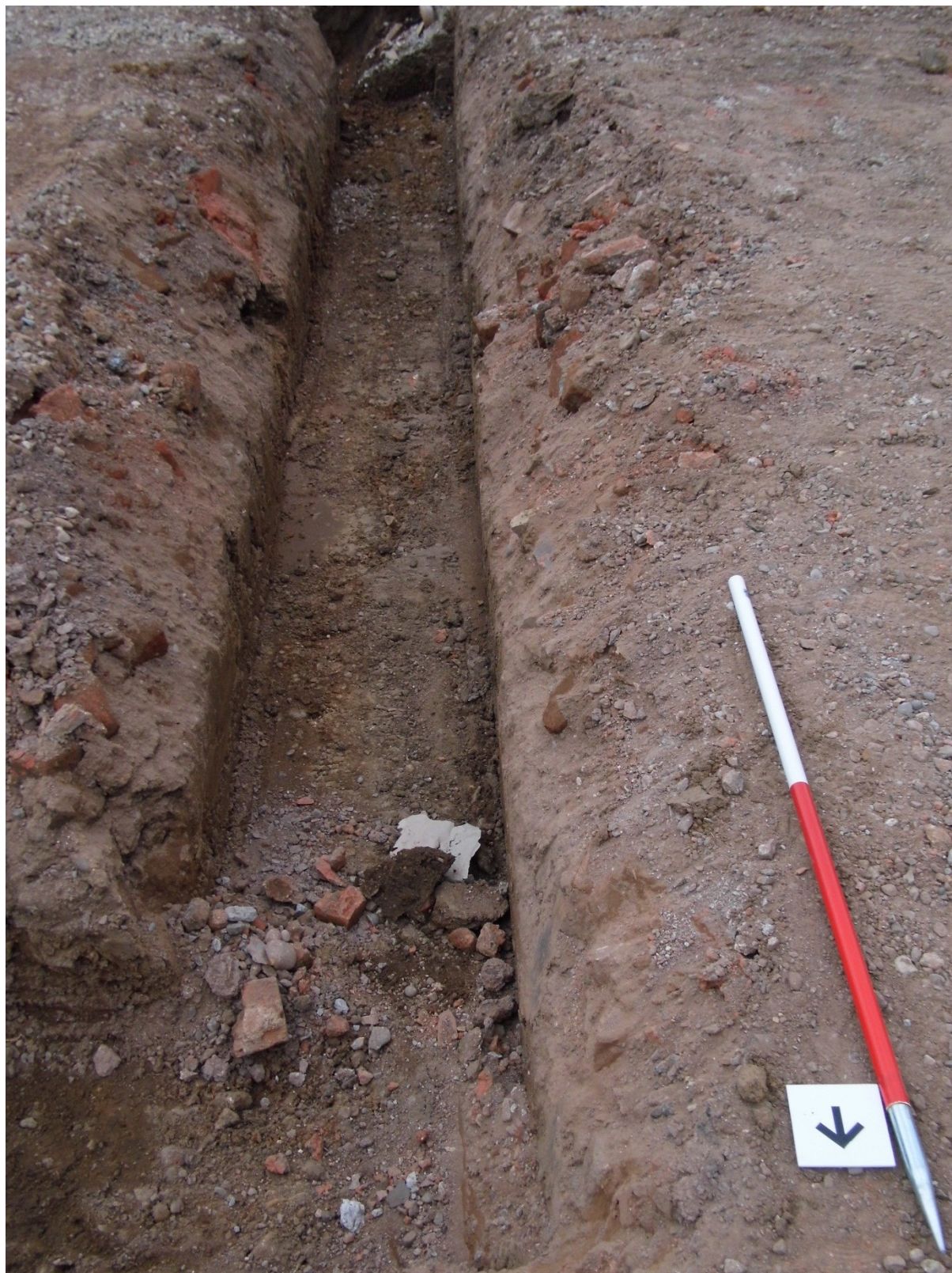
Figure 5. Western side of foundation trench in Plot 25.
