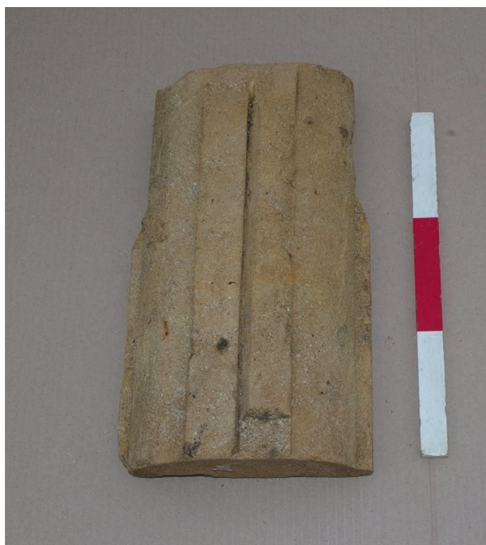
Figure 24. Window mullion B, ovolo-profile (incomplete). Scale 300mm.
