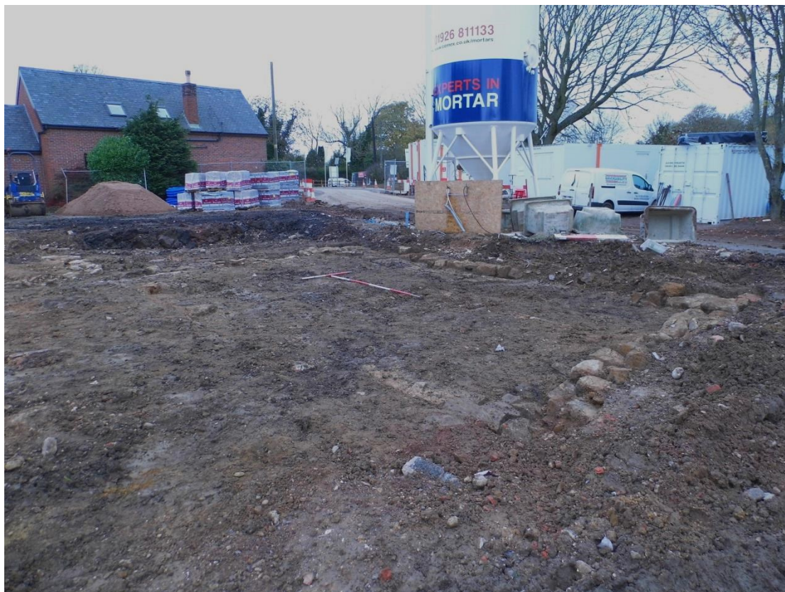
Figure 6: General view north across building (2m scales)
