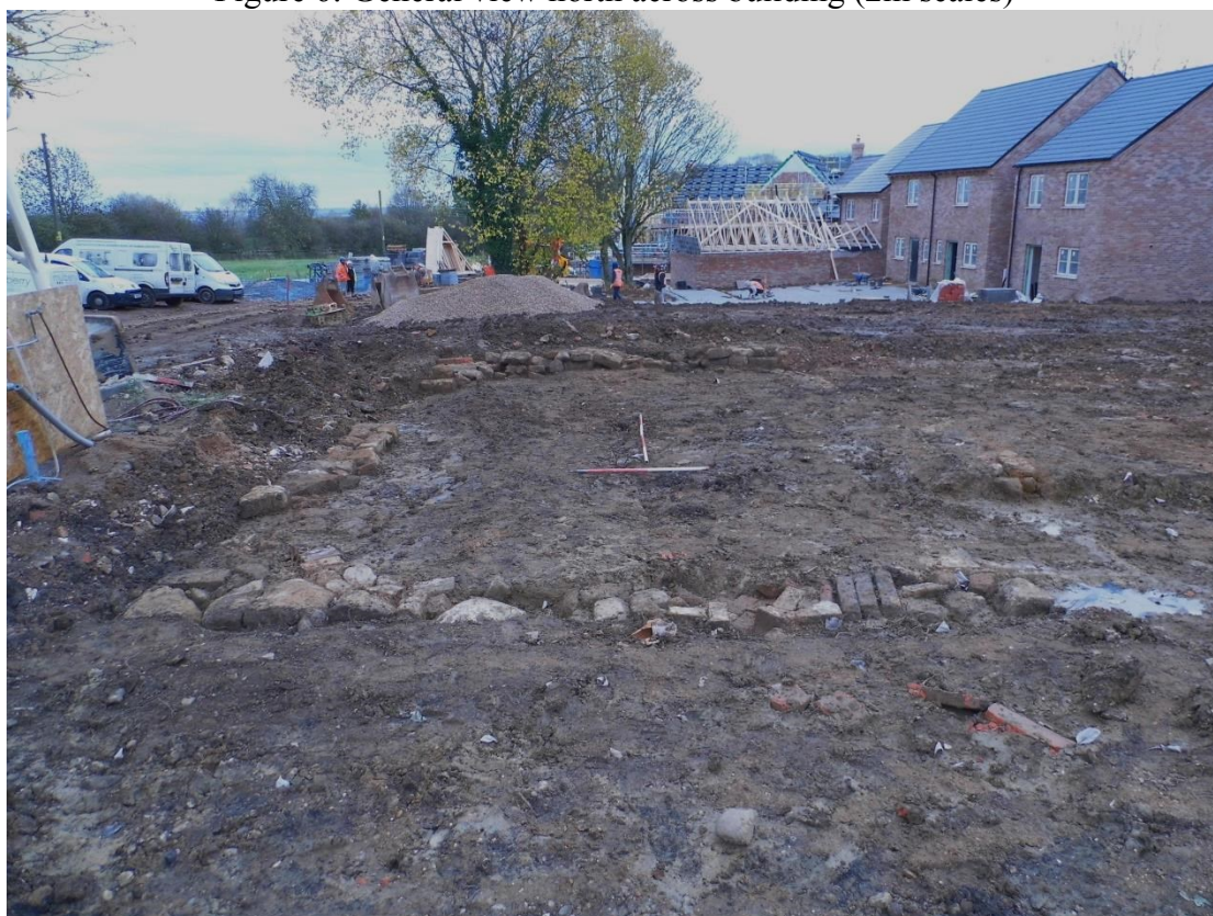
Figure 7: General view north-east across building (2m scales)
