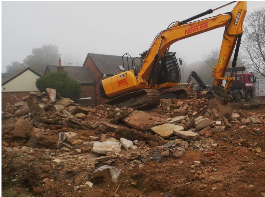
Figure 4: Demolition of the manor house in progress
