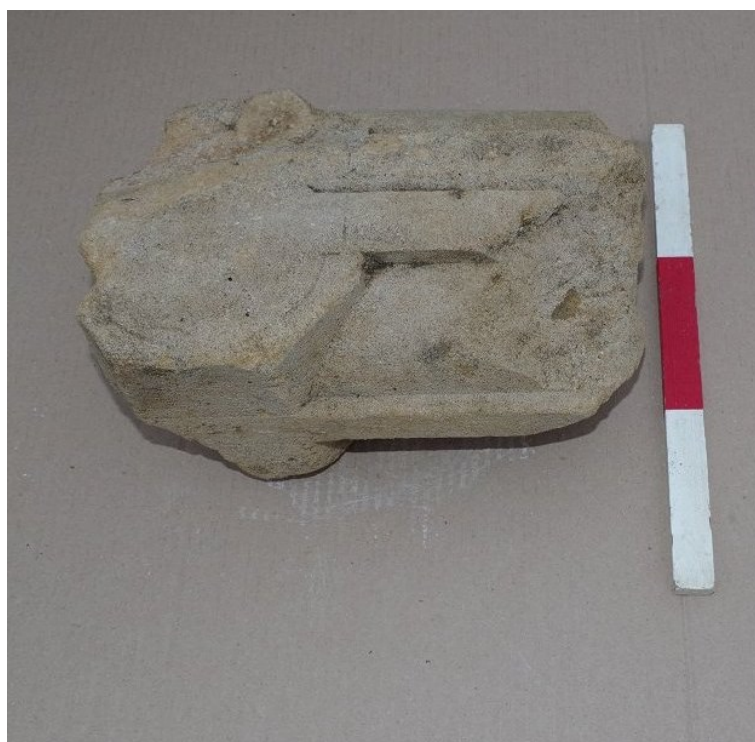
Figure 28. Window transom F. Note scribed mark on upper surface for ovolo mullion. Scale 300mm.
