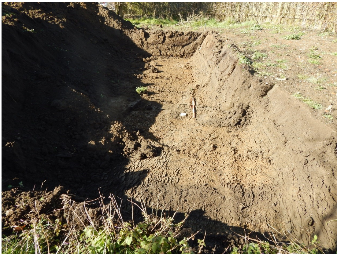
Plate 3: Trench 1 being excavated looking west with the water pipe trench in the foreground
