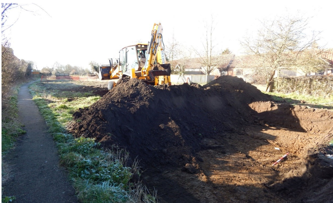
Plate 2: Work in progress on Trench 1, looking south-west
