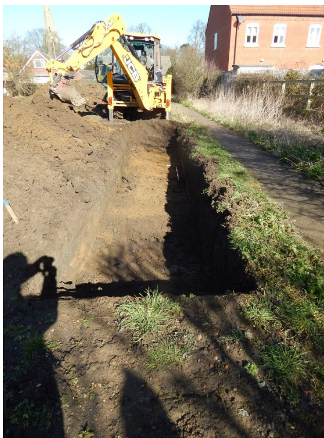
Plate 6: Post excavation shot of Trench 3, looking north
