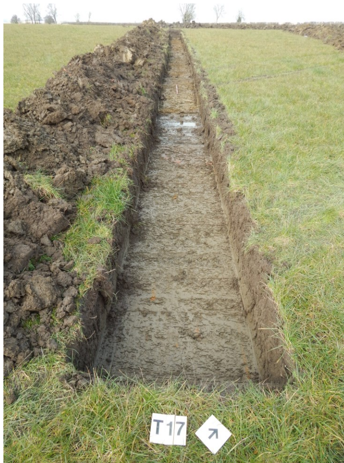
Plate 7: Trench 17, post excavation, looking north-west
