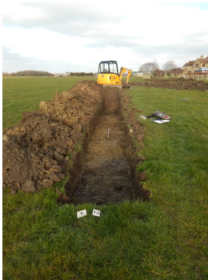
Plate 5: Trench 12, post-excavation and partially back-filled, looking north-east
