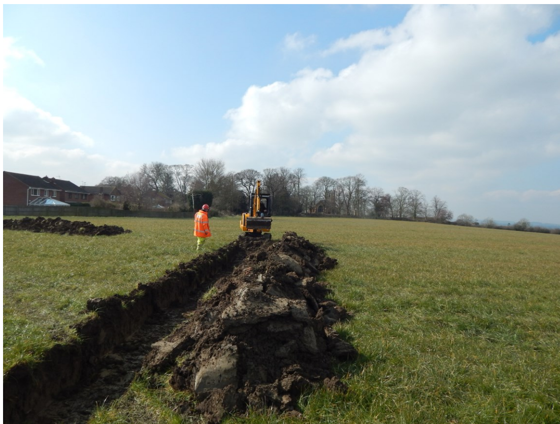
Plate 6: Work in progress, Field 3, Trench 16, looking west
