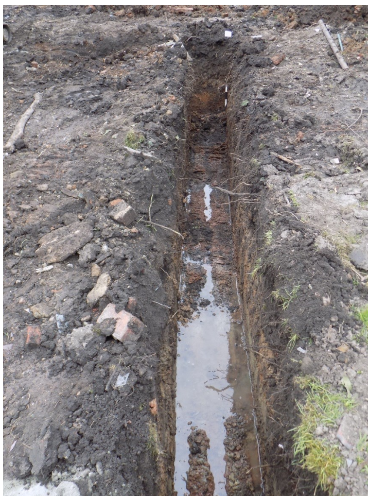
Figure 4 Western trench for garage looking north.
