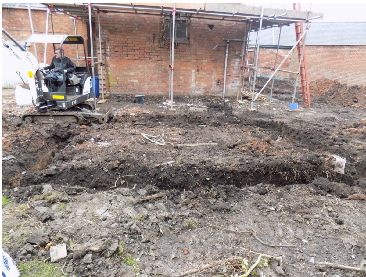
Figure 5 Completed footing trenches for garage.
