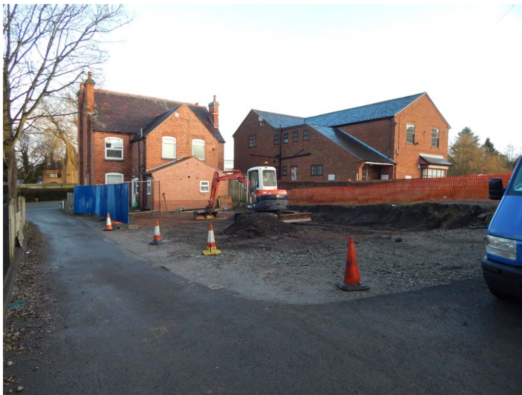
Figure 4: The site being stripped prior to excavation, looking north
