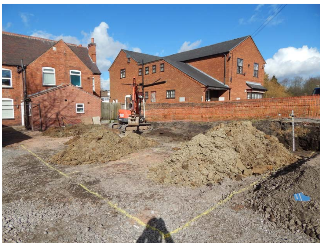
Figure 5: Work in progress on north-east trench, looking north
