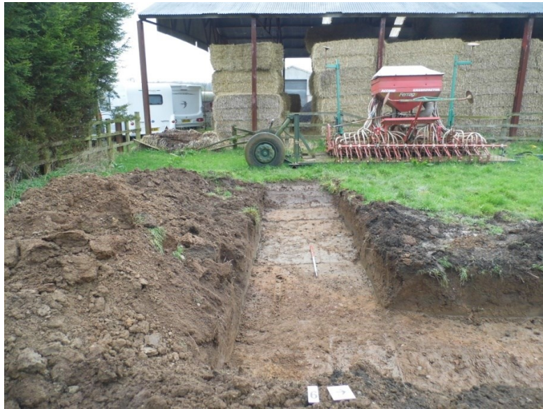
Figure 7: Trench 6, looking west
