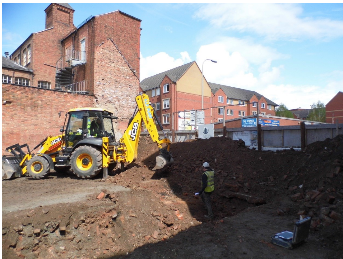
Figure 4: Machining in progress
