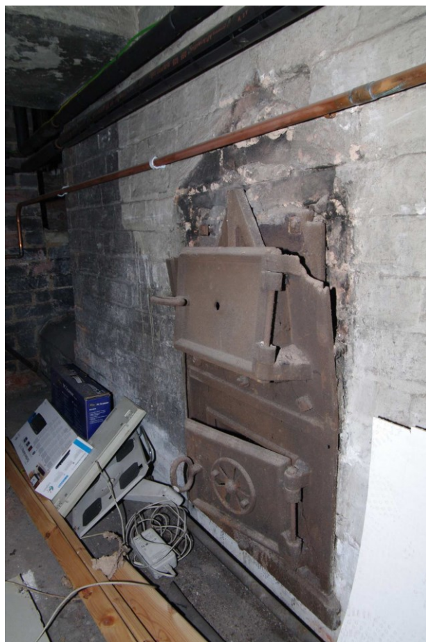
Figure 27 Cellar C1. Boiler door at southern end of room Looking west
