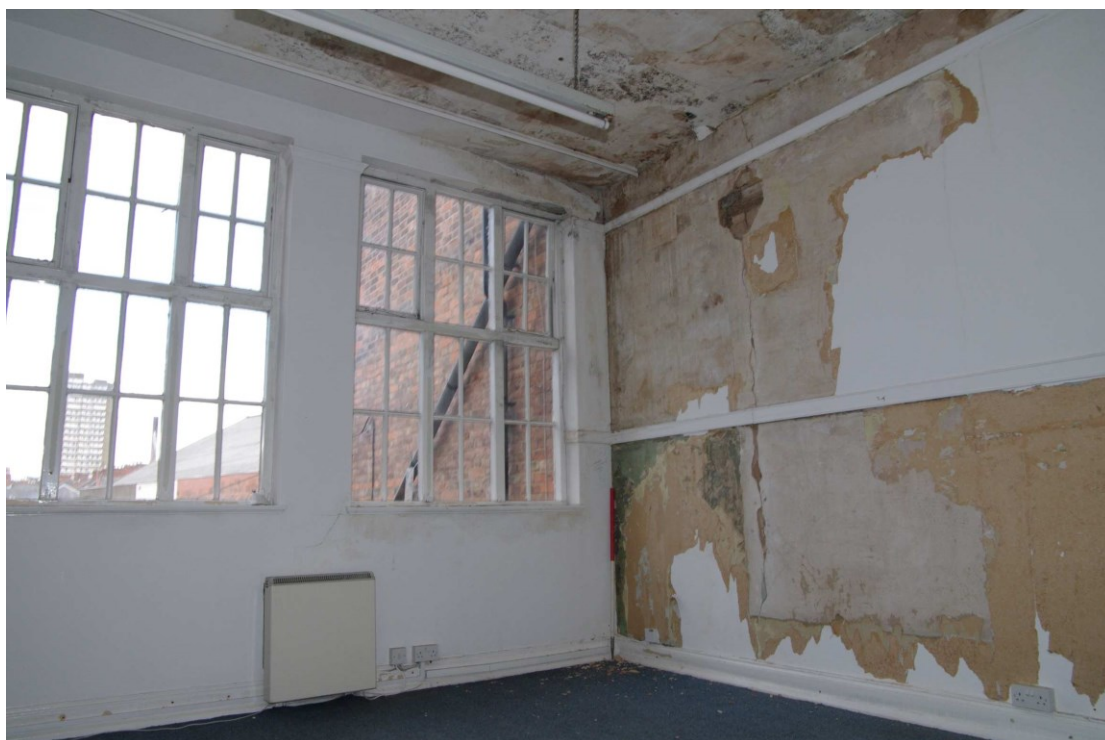
Figure 58 F7 Looking north-east. 1m scale
