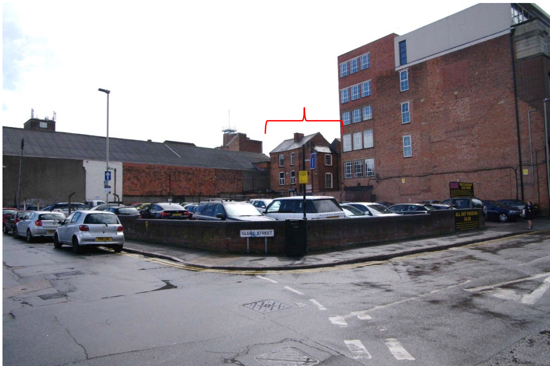
Figure 10 Rear of 54 to 58 Looking south-east from the corner of Conduit Street and Glebe Street (part of Number 54 obscured by building on right of picture)
