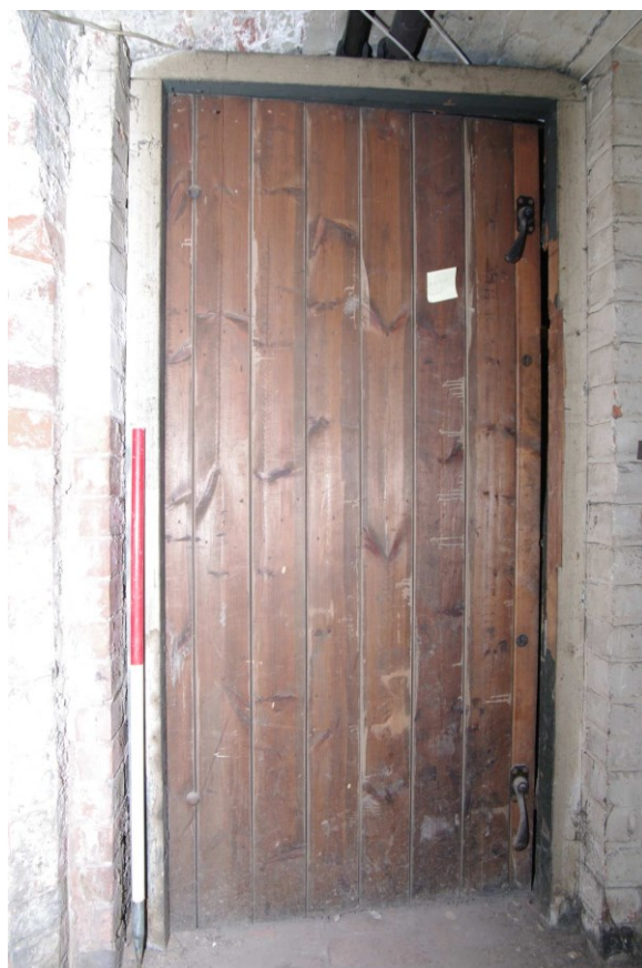
Figure 28 Door from C1 to C2 Looking south-east. 1m scale
