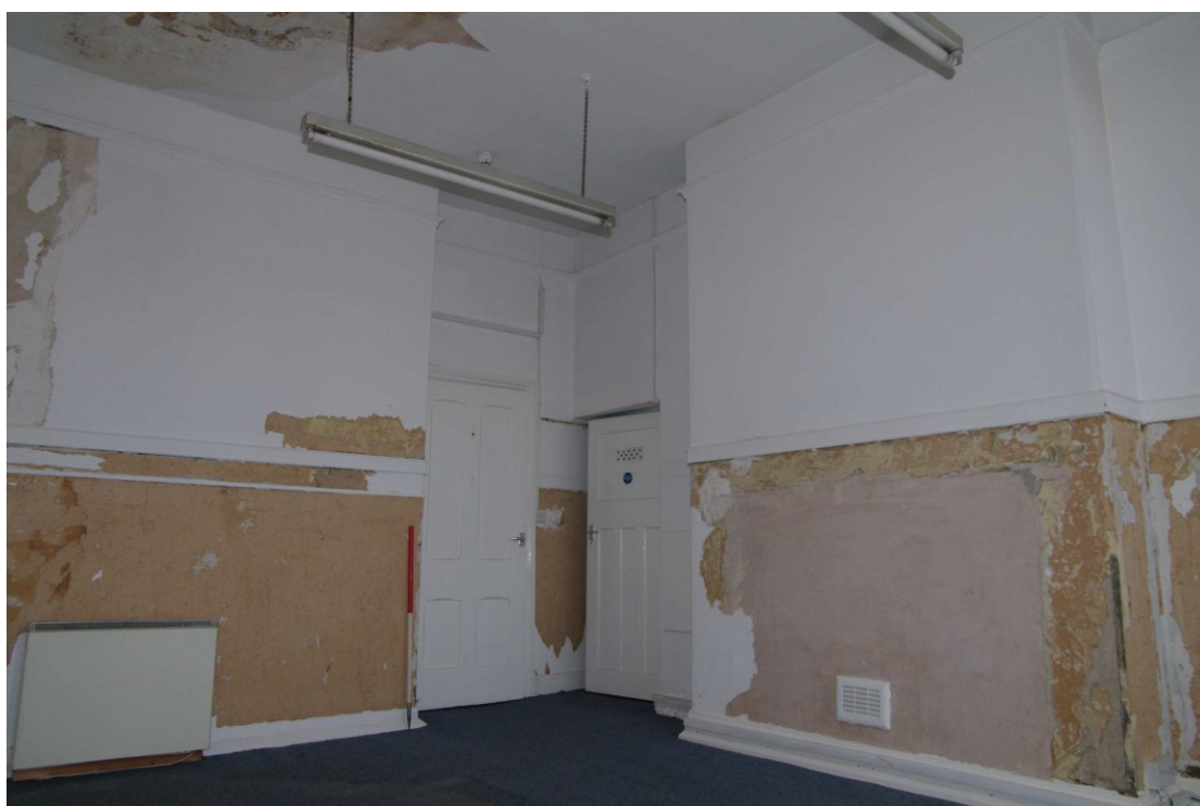
Figure 59 F7 Looking west. 1m scale
