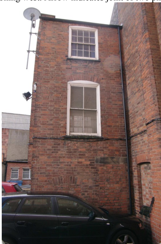
Figure 22 North-west facing elevation of second phase extension to rear of No 56 Looking south-east. Note blocked door and window at ground floor
