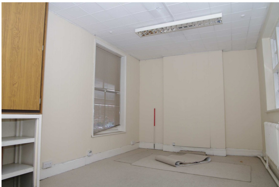
Figure 62 F11 Looking north-east. 1m scale
