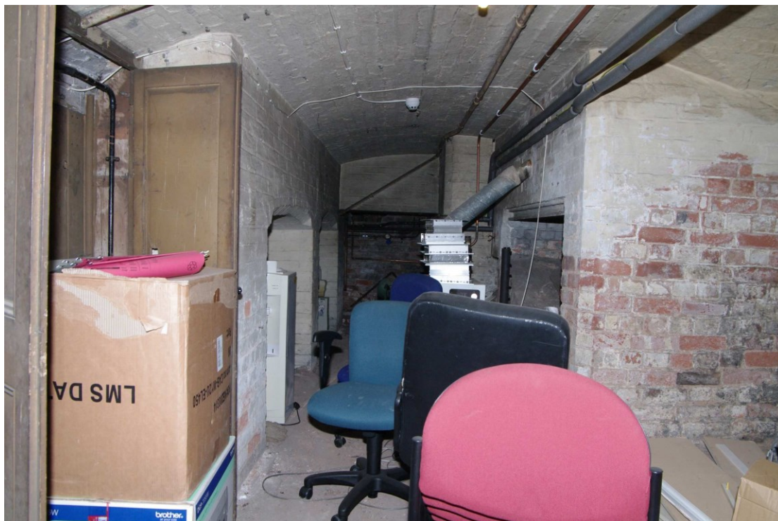
Figure 26 Cellar C1 Looking south-west
