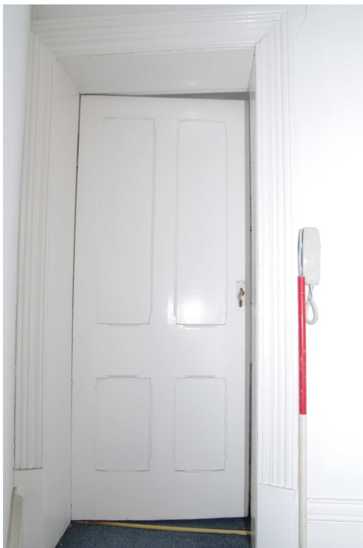
Figure 53 F2 doorway 1m scale
