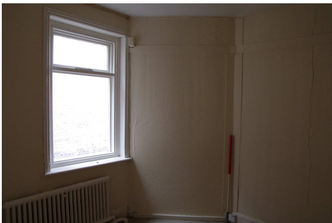
Figure 61 F10 Looking north. 1m scale
