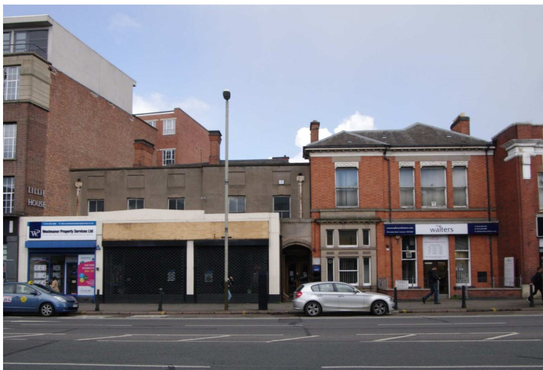
Figure 14 South-west facing elevation Looking north-east. 54 to 58 from left to right
