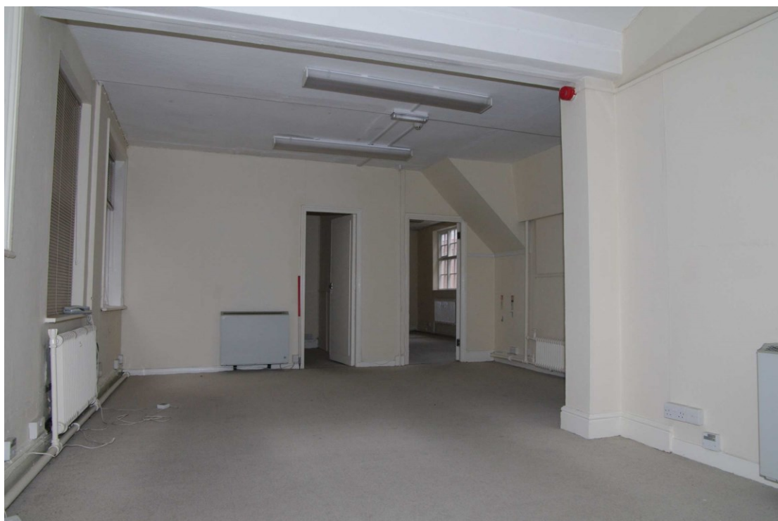
Figure 60 F9 Looking north-east. 1m scale
