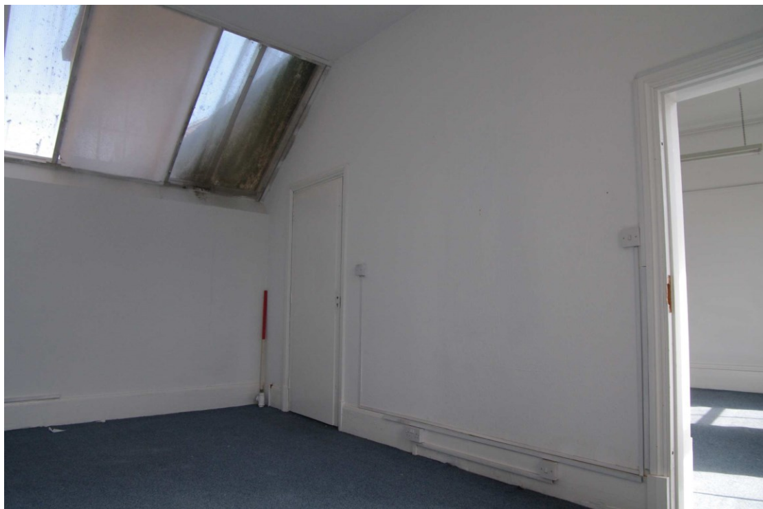
Figure 50 F1 Looking north-east. 1m scale
