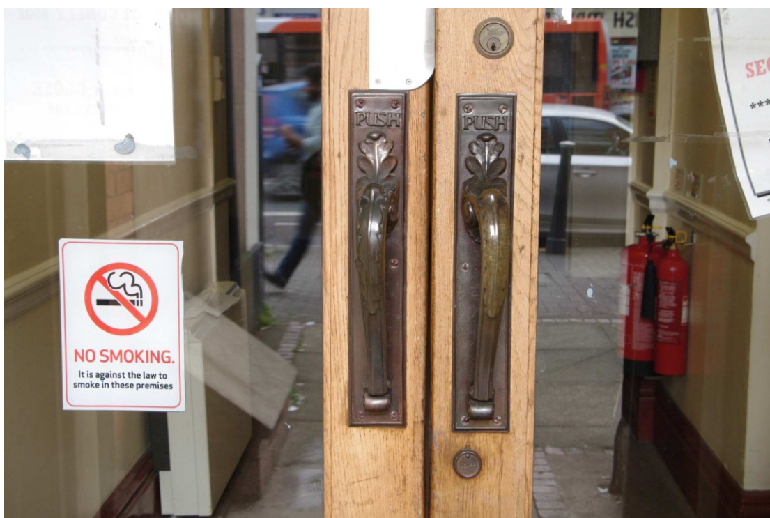
Figure 16 Door handles on main doorway, south-west facing elevation Looking north-east
