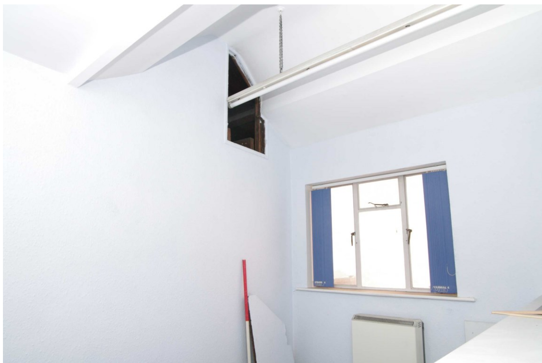
Figure 71 S1 Looking west. 1m scale. Note pitched ceiling
