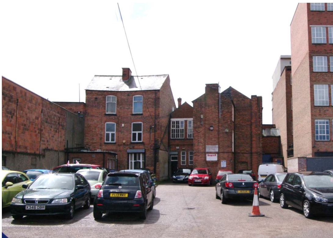
Figure 19 North-east facing elevation and extensions Number 58 on left of picture
