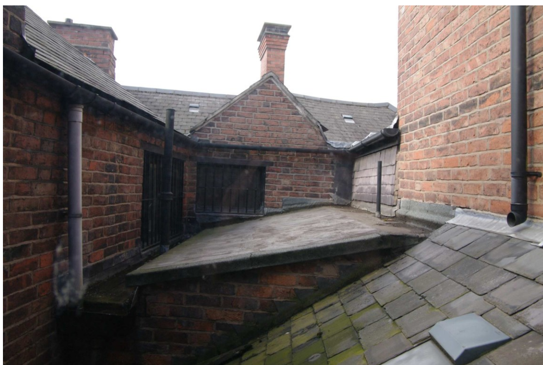
Figure 74 View of roof from S5 Looking west
