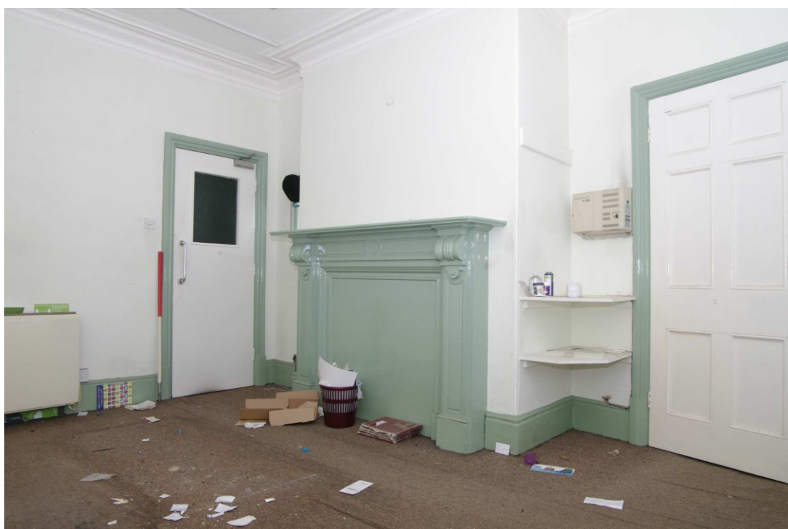
Figure 65 F14 Looking west. 1m scale
