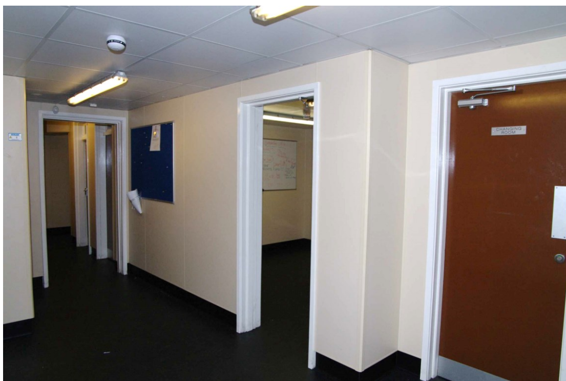
Figure 41 G8 and side rooms Looking south-west
