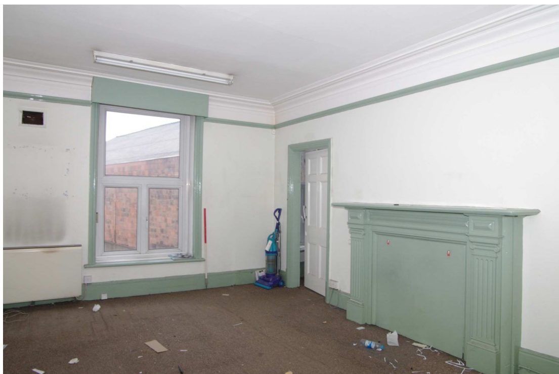
Figure 64 F13 Looking east. 1m scale. Doorway into F14 in centre of picture
