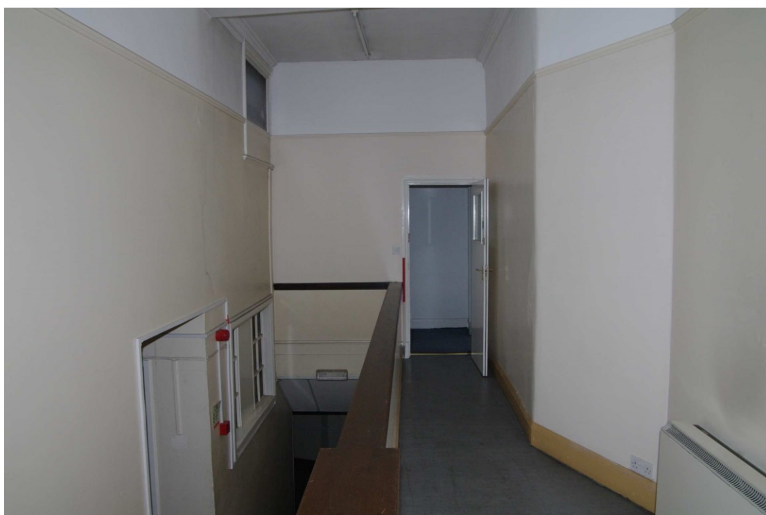
Figure 57 F4 landing and stairs Looking east. 1m scale
