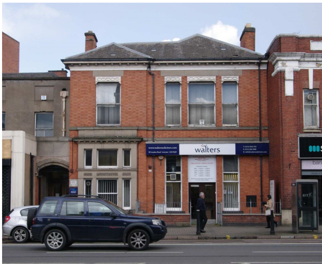
Figure 17 Number 58 south-west facing Looking north-east
