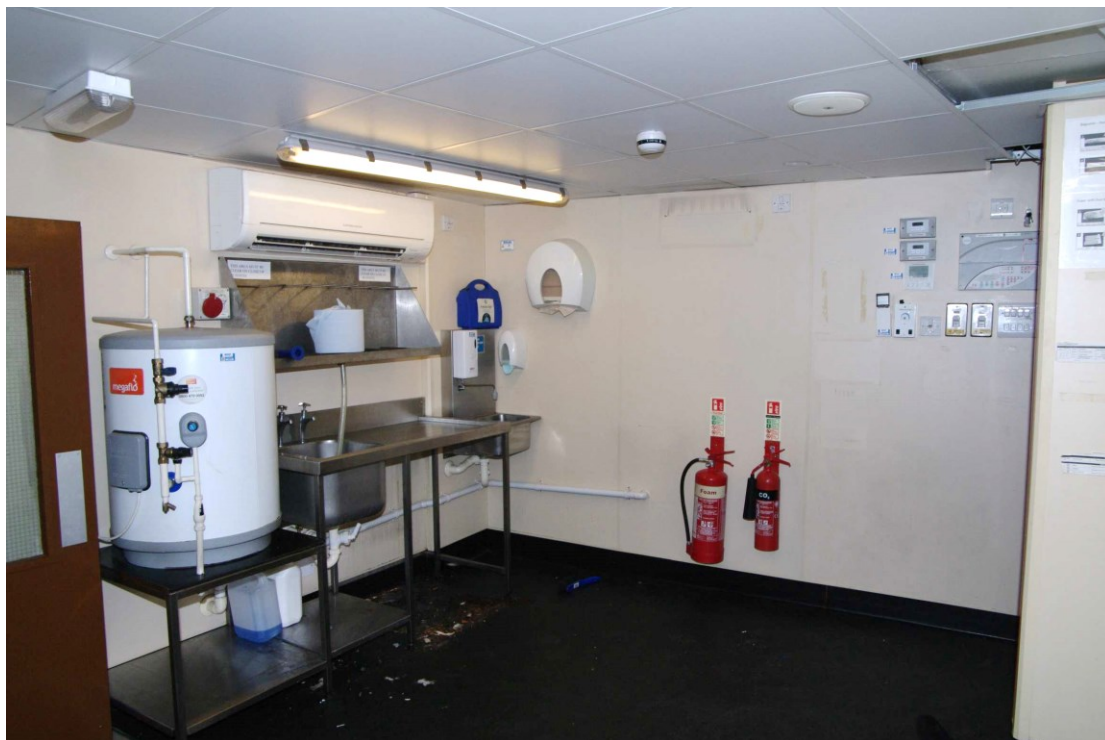
Figure 40 G7 food preparation area Looking south-east
