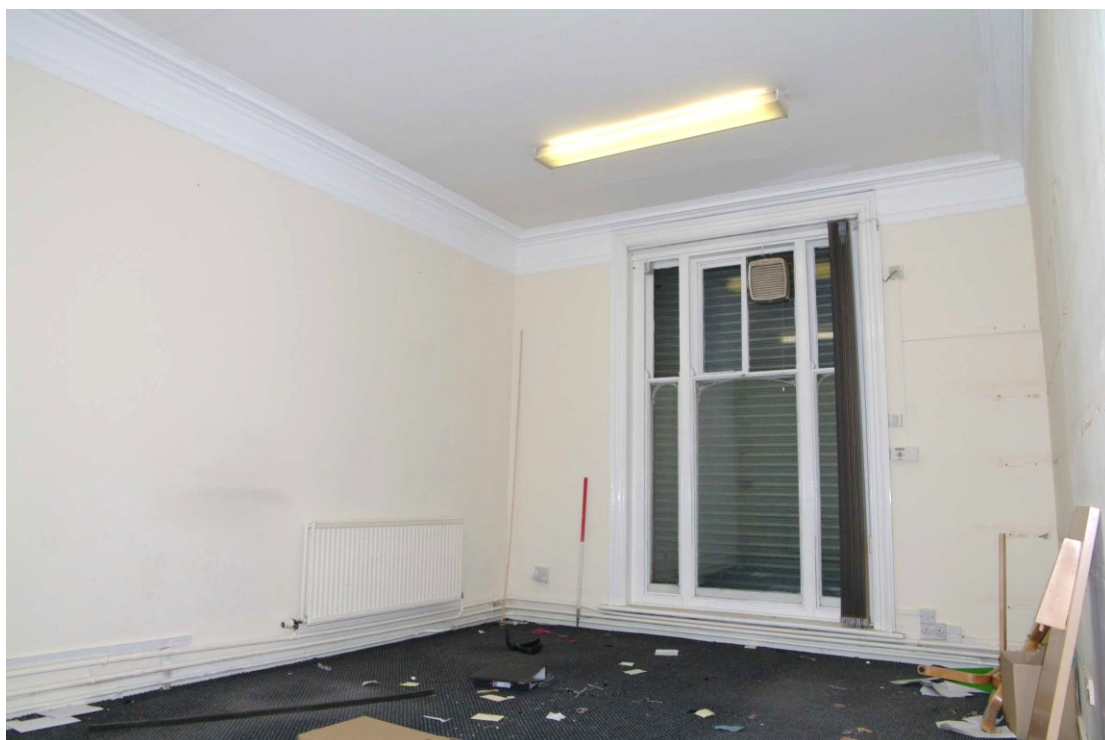
Figure 48 G18 Looking north. 1m scale
