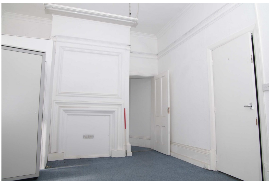
Figure 55 F3 Fireplace Looking north-west. 1m scale
