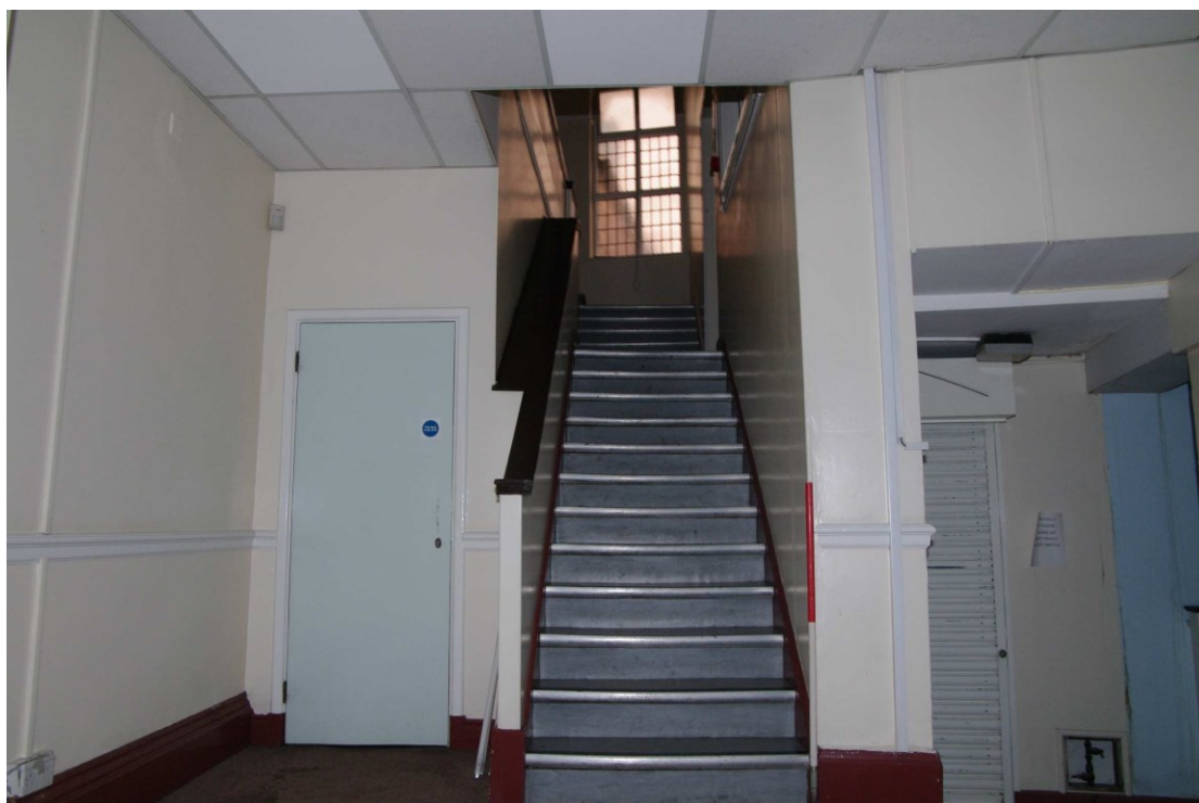
Figure 56 Stairs from G2 up to first floor Looking north-west. 1m scale
