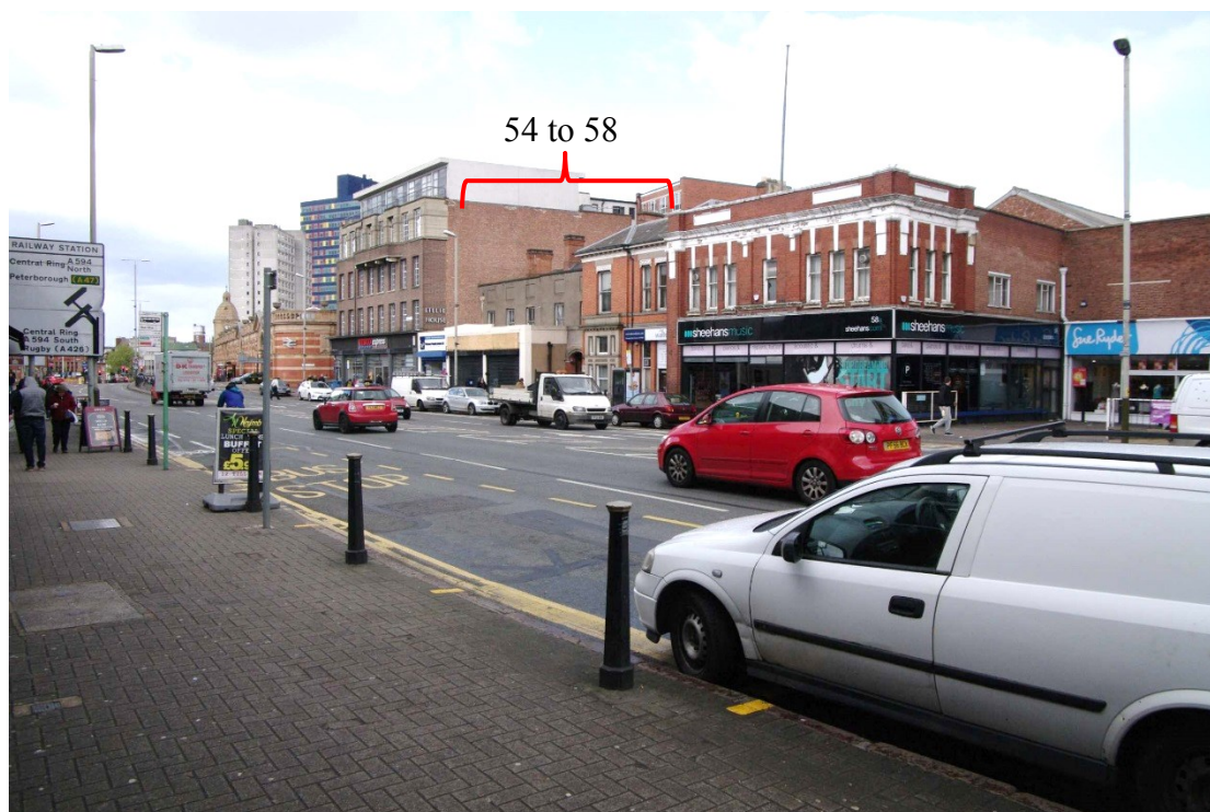
Figure 8 54 to 58 London Road Looking north across London Road. Buildings highlighted
