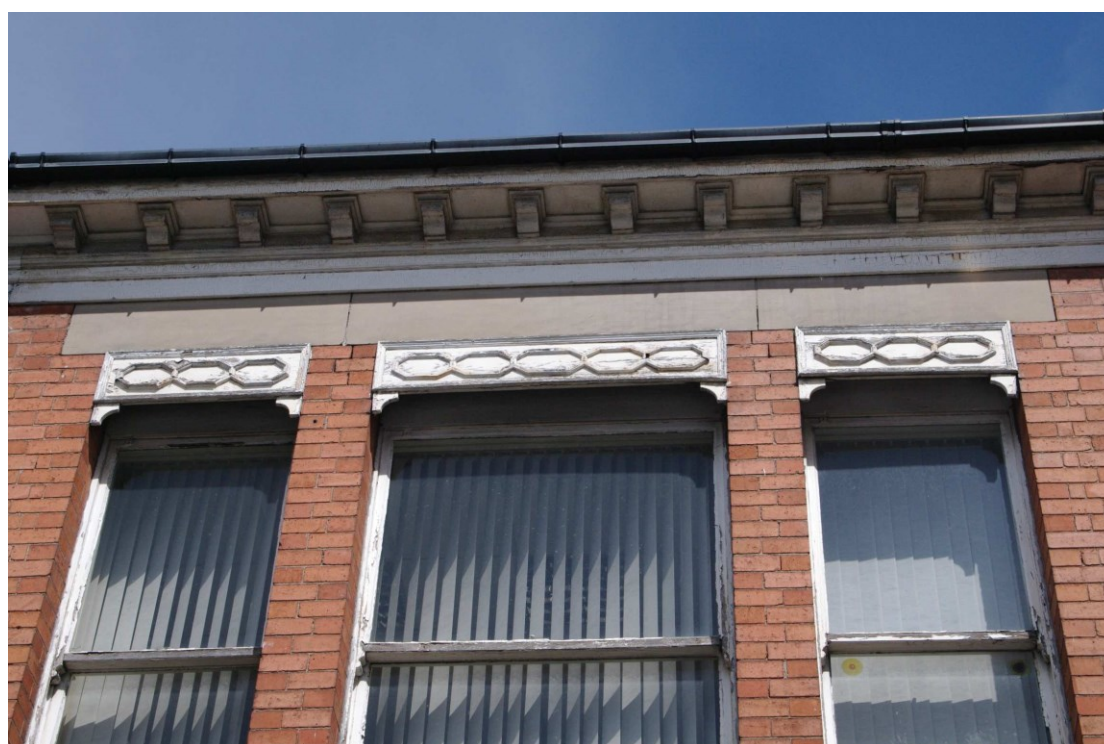
Figure 18 Number 58 south-west facing first floor window detail Looking north-east
