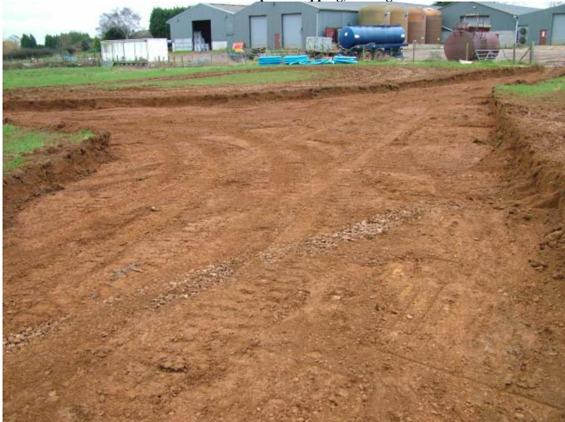
Plate 4: Area after topsoil stripping, looking south east
