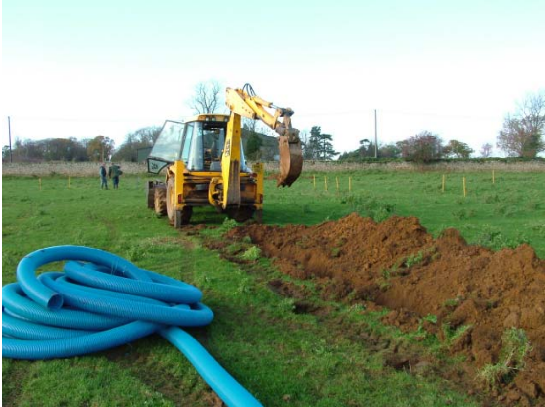
Plate 1: Work in progress on drains, looking west
