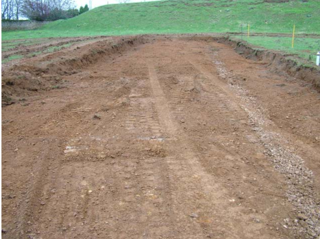
Plate 3: Area after topsoil stripping, looking north
