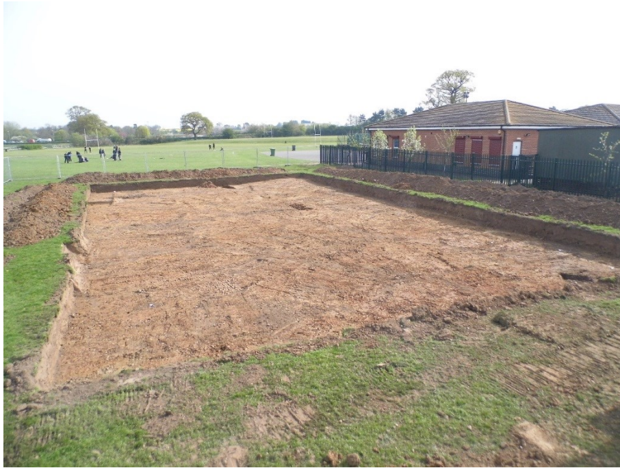
Figure 10: Excavation area, looking north-east
