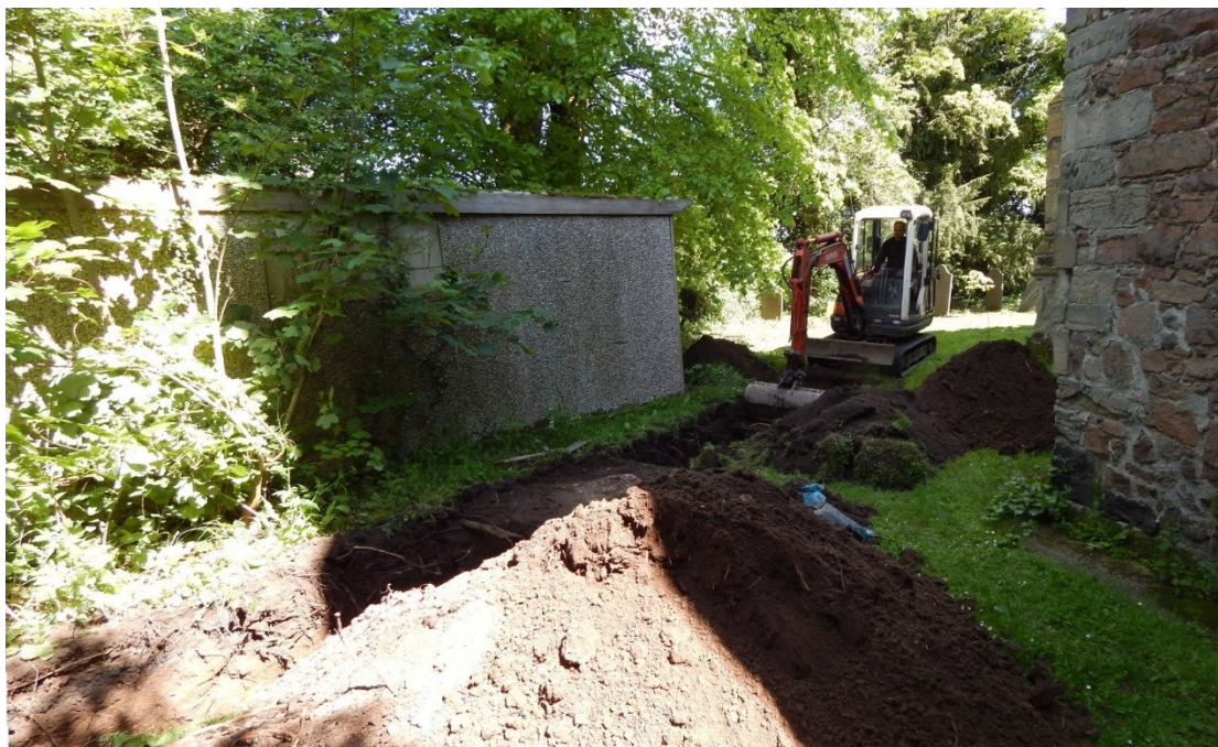
Plate 1: Work in progress on T P 07
