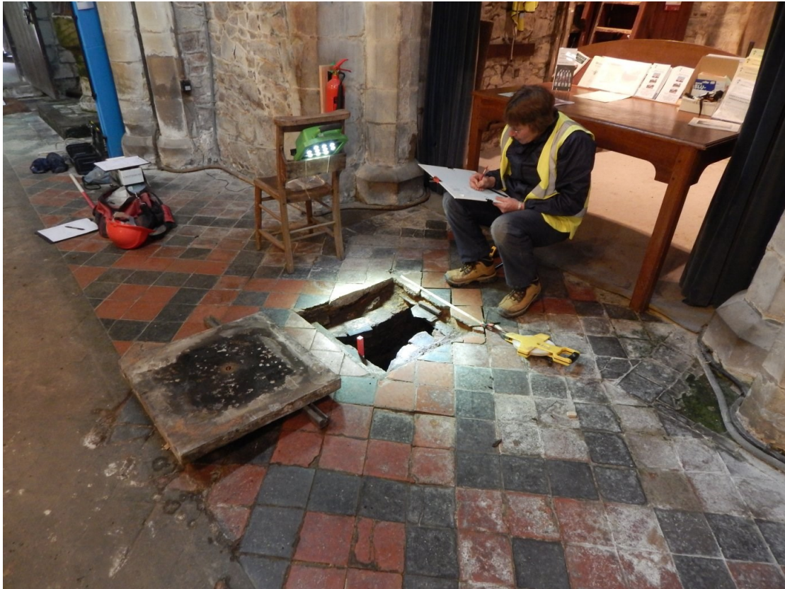
Plate 7: Work in progress recording T.P 05, looking south-west
