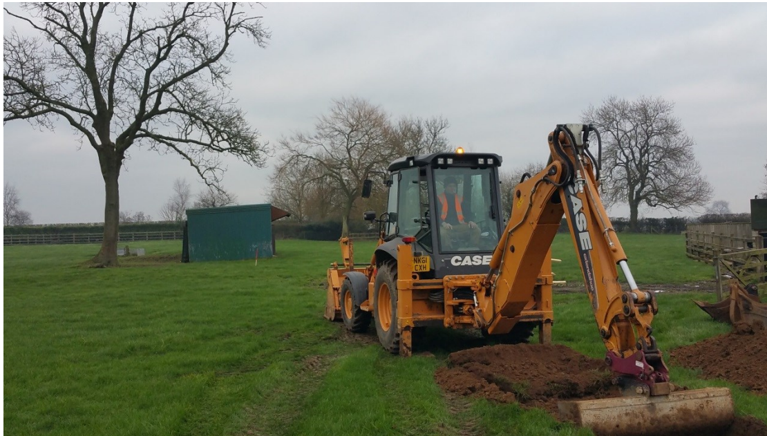
Figure 5: Excavation in progress
