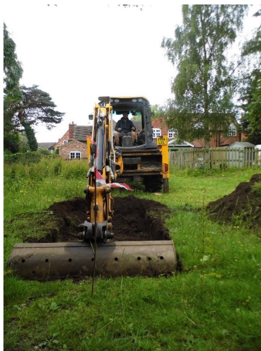
Figure 7: Excavating Trench along building footprint , looking south.
