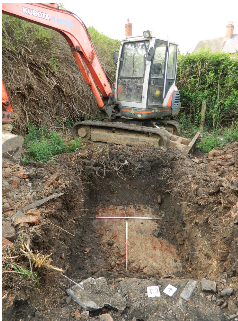
Figure 8 Trench 3 extension viewed from the south.
