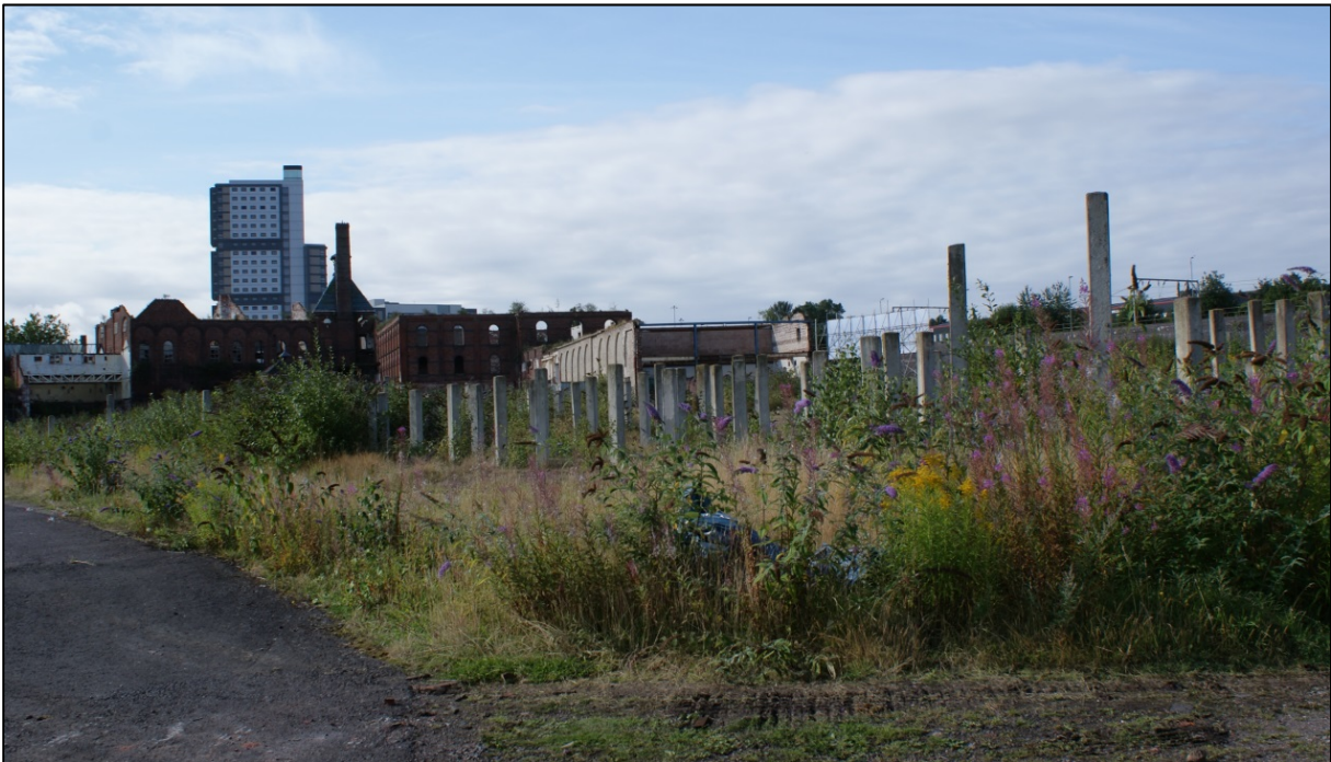
Figure 8: Photograph of the north east corner of the site looking south, with the concrete plinth and piling in the foreground.
