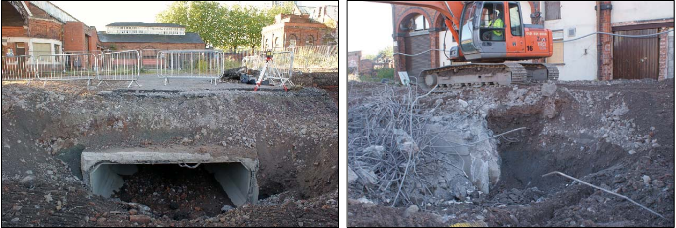
Figure 12: Large culvert running length of building footprint, looking south then north
