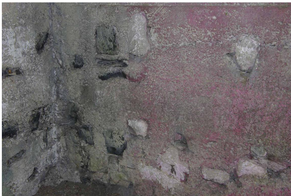
Figure 23 Granite blocks visible within wall fabric
