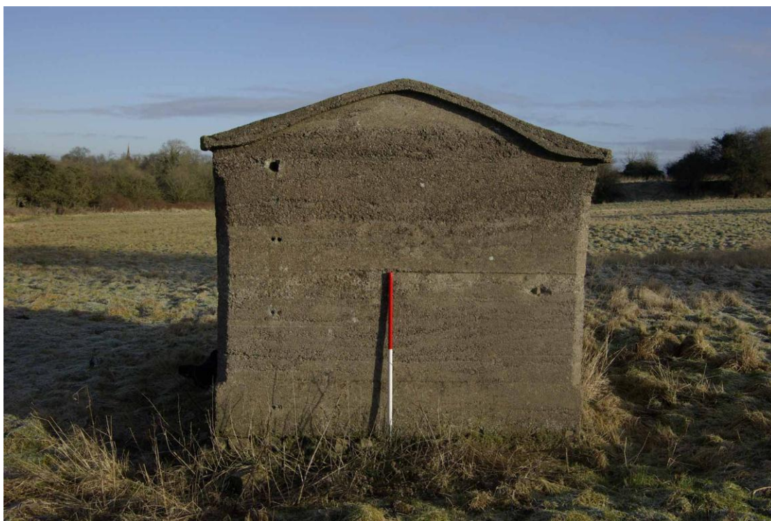
Figure 15 South-west facing elevation
