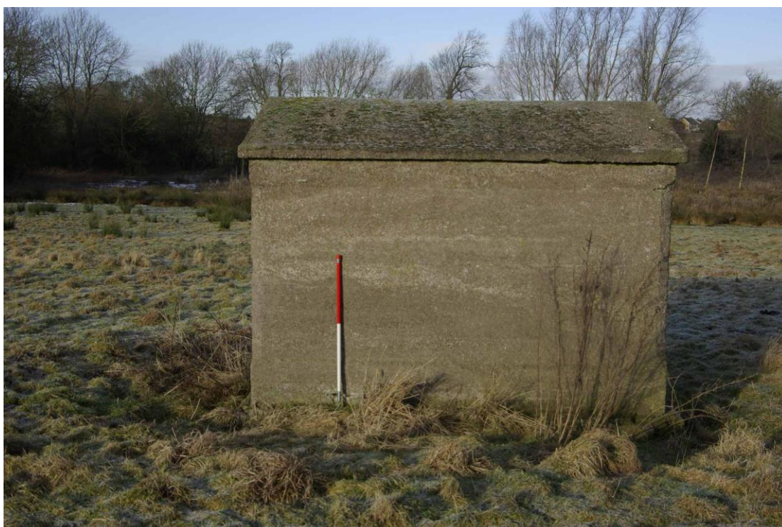
Figure 14 South-east facing elevation Looking north-west. 1m scale
