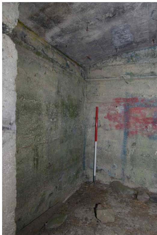
Figure 21 Internal view Looking south. 1m scale
