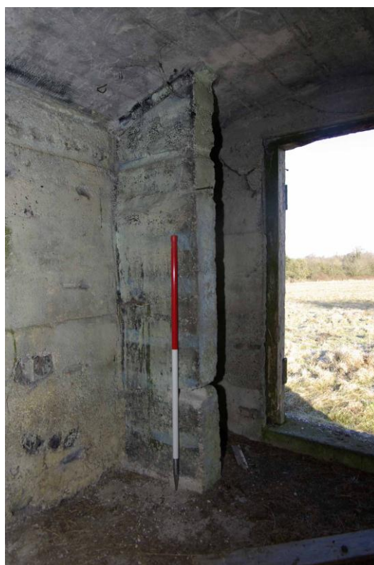
Figure 22 Internal view Looking north. 1m scale
