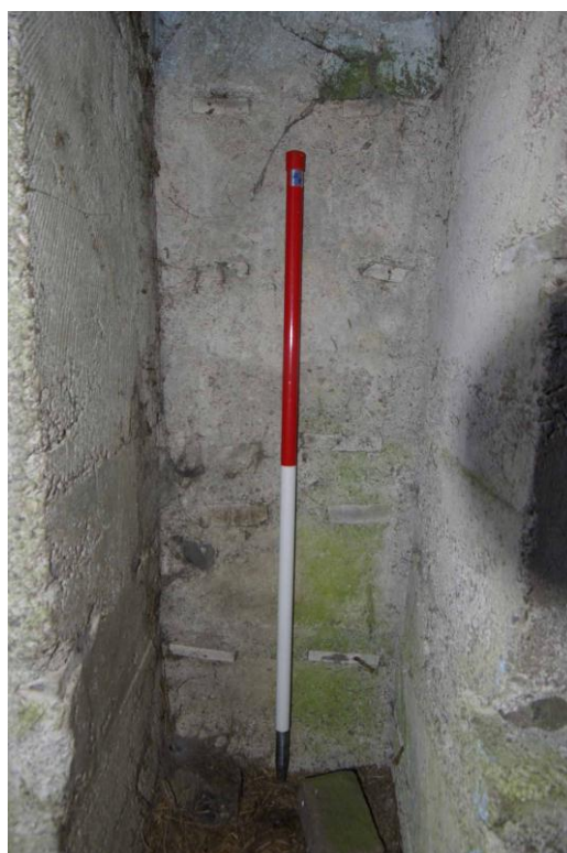
Figure 20 Alcove between inner and outer walls Looking east. 1m scale. Inserted stubs of wooden planking can be seen either side of scale
