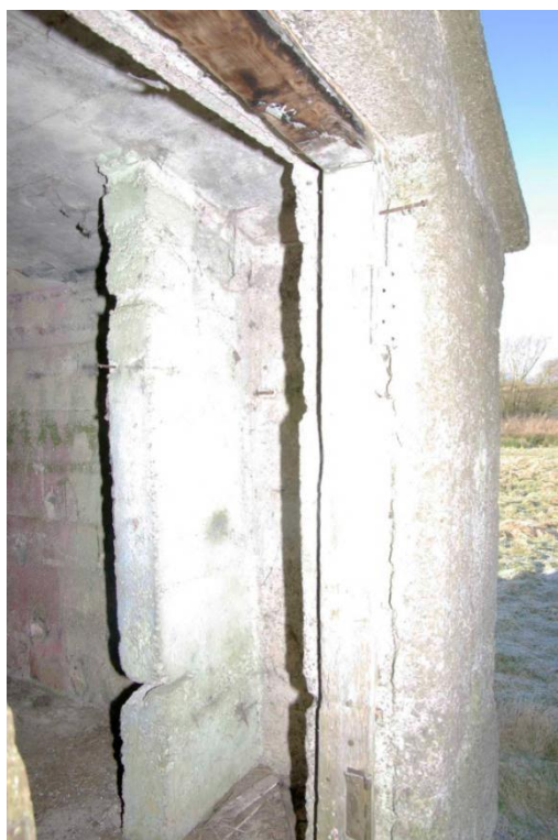
Figure 19 Internal wall Looking south-west
