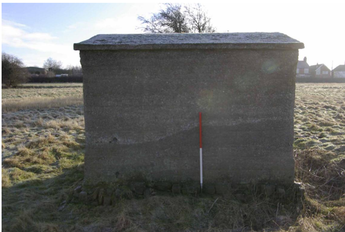
Figure 16 North-west facing elevation
