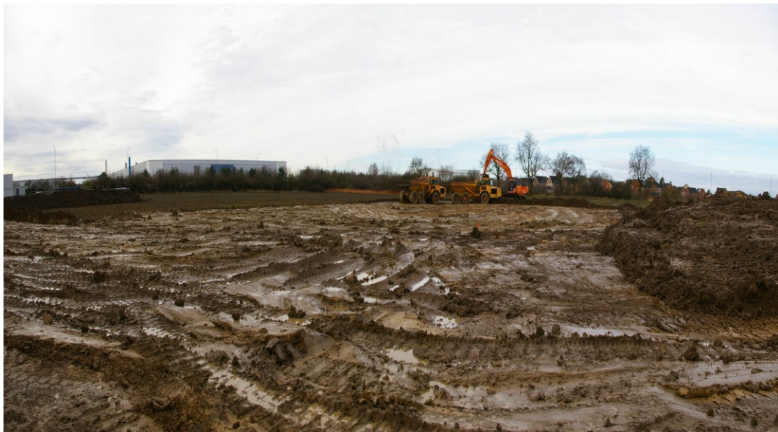
Plate 2: Stripping underway on main site, looking north
