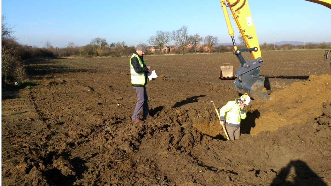
Plate 1: Test pits under excavation, looking west
