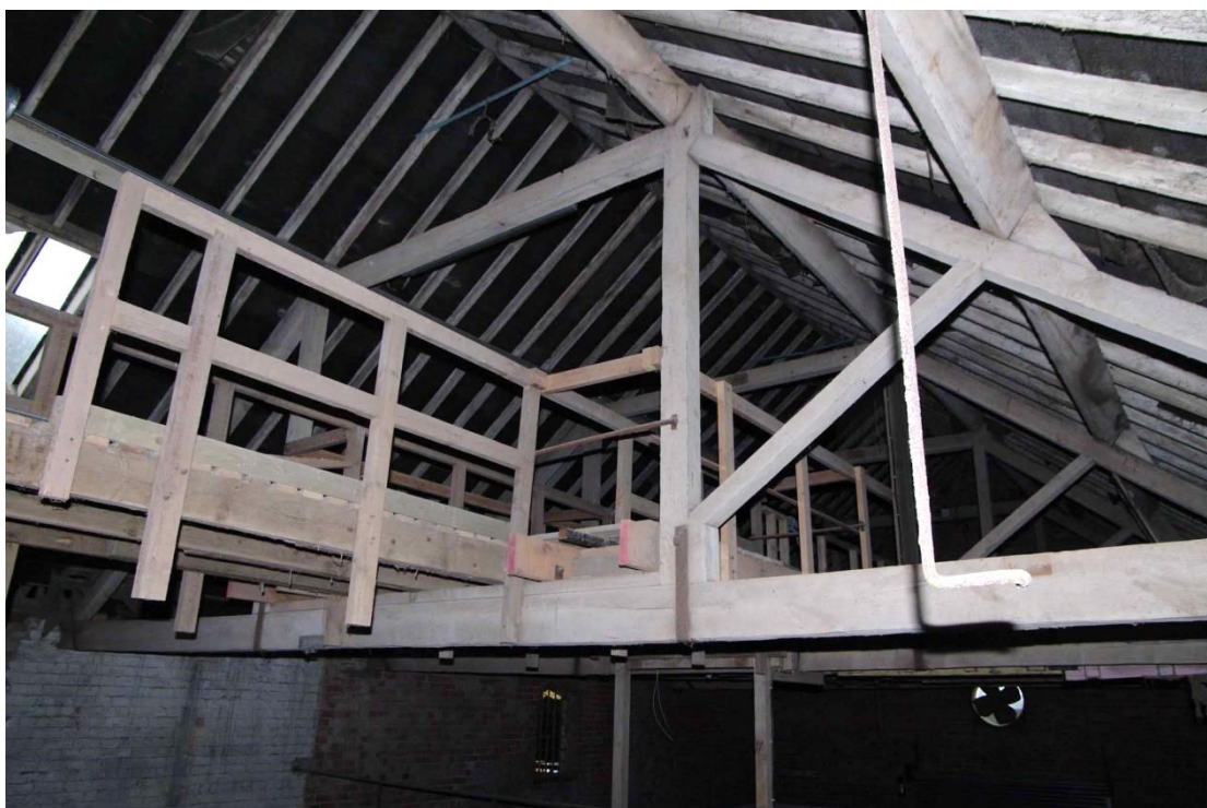
Figure 31: Granary roof structure at west end of building Looking south-west
