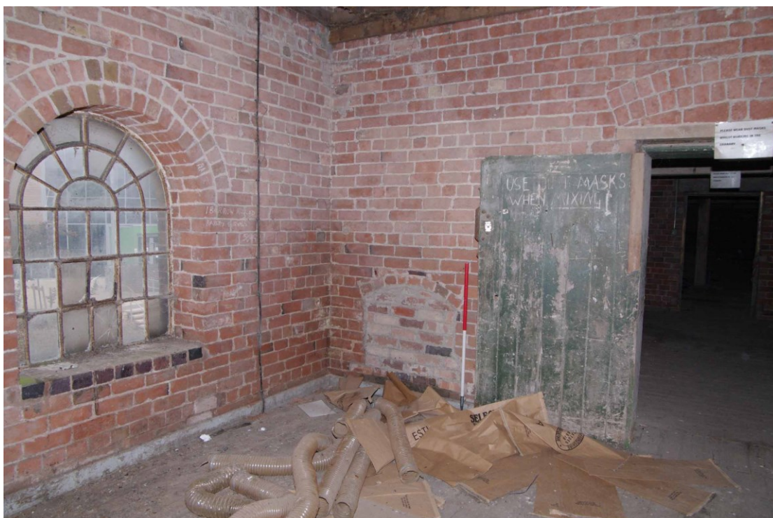
Figure 49: Granary, first floor Room F2 Looking north-east. 1m scale
