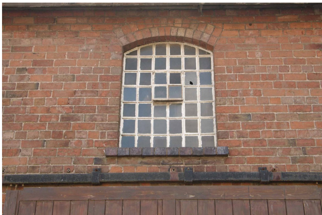
Figure 14: East facing elevation, first floor eastern end window detail Looking south
