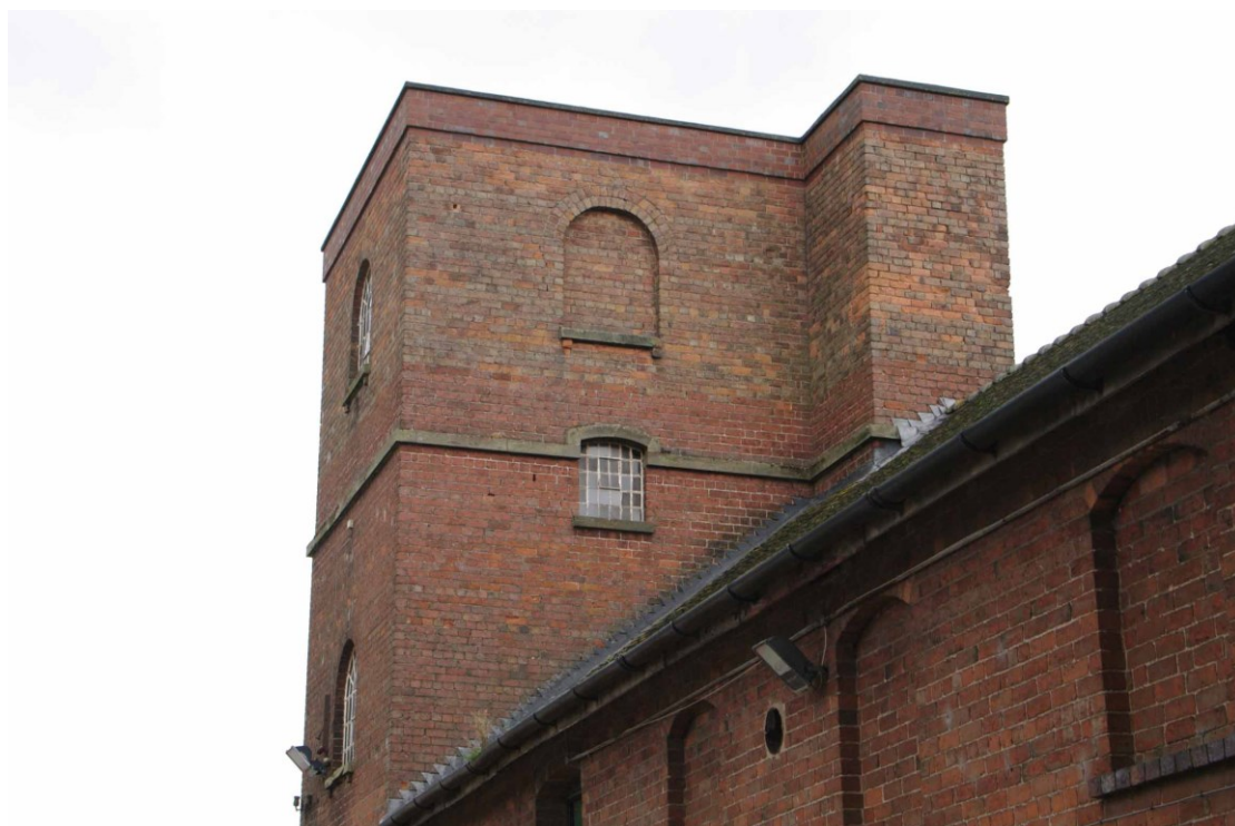
Figure 17: Granary tower, west facing elevation Looking south-east
