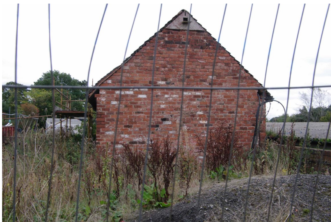
Figure 67 Gasometer building, west facing elevation Looking east
