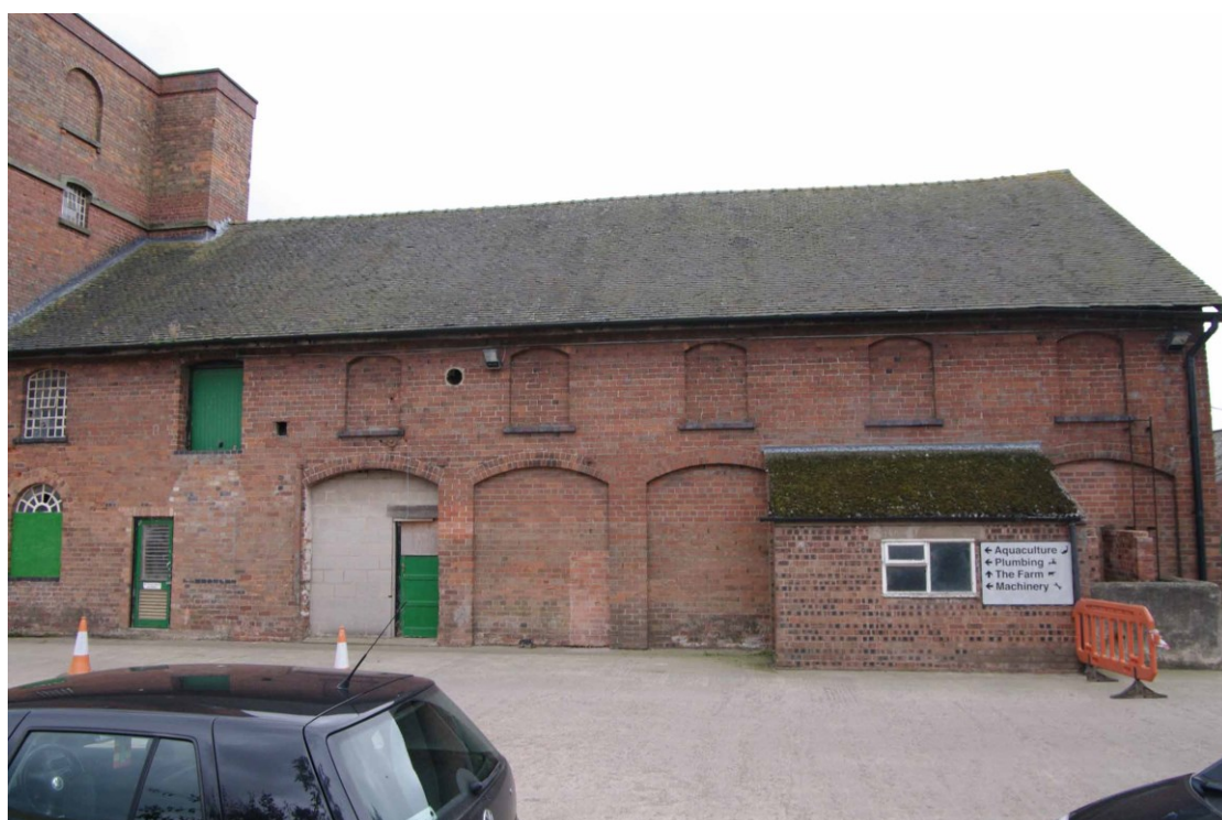
Figure 18: Granary north facing elevation, western end Looking south
