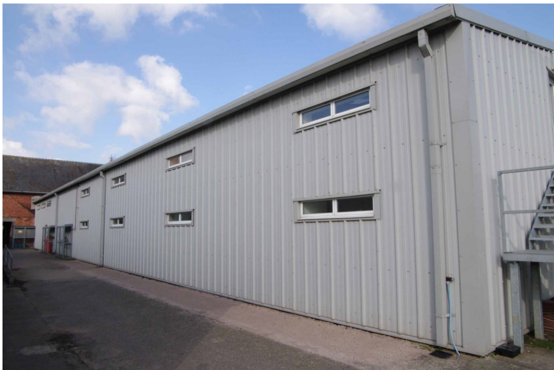
Figure 63: South-eastern rear range. West facing elevation Looking north-east
