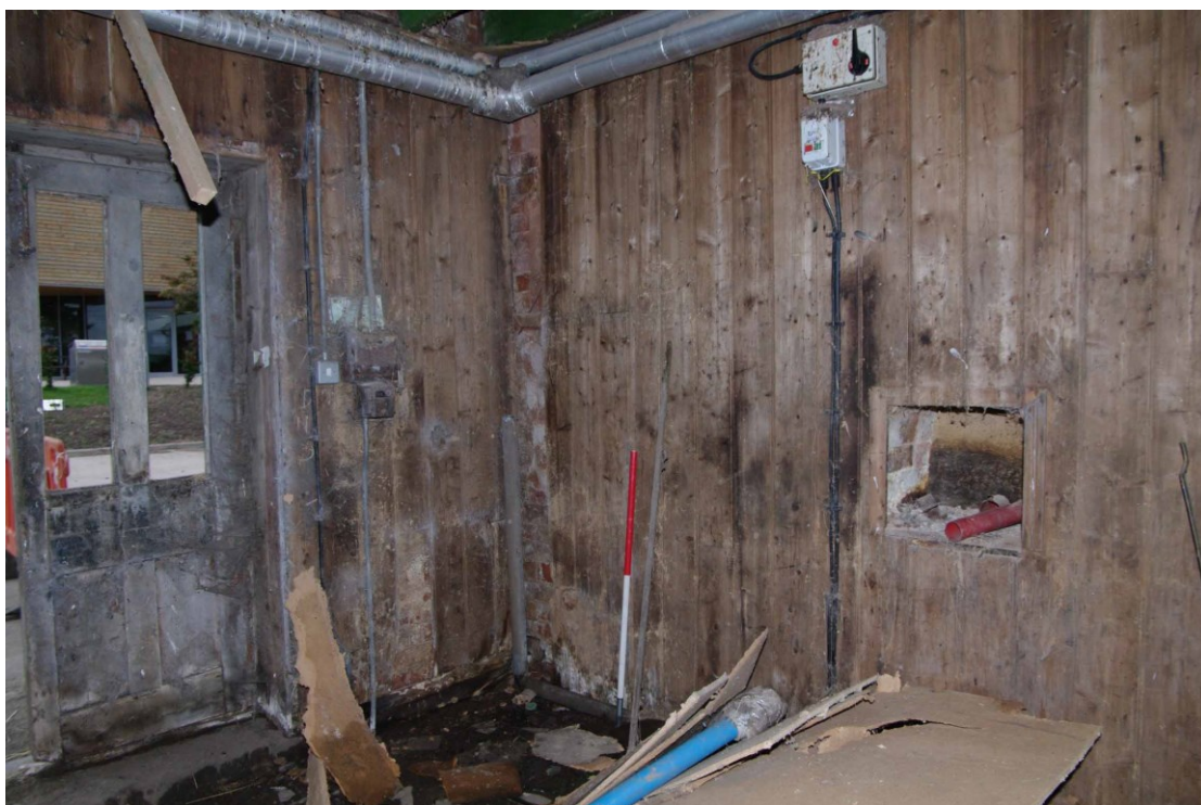
Figure 37: Granary, ground floor Room G2 Looking north-east. 1m scale
