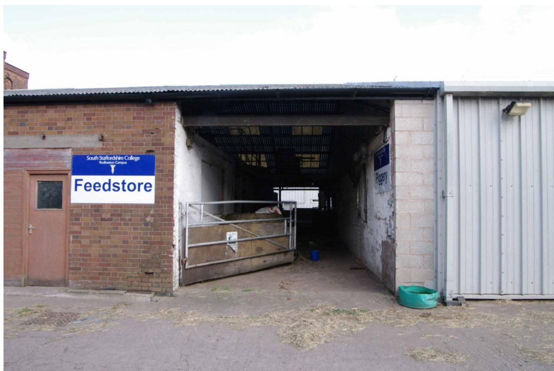
Figure 61: South-western rear range, west facing elevation Looking east
