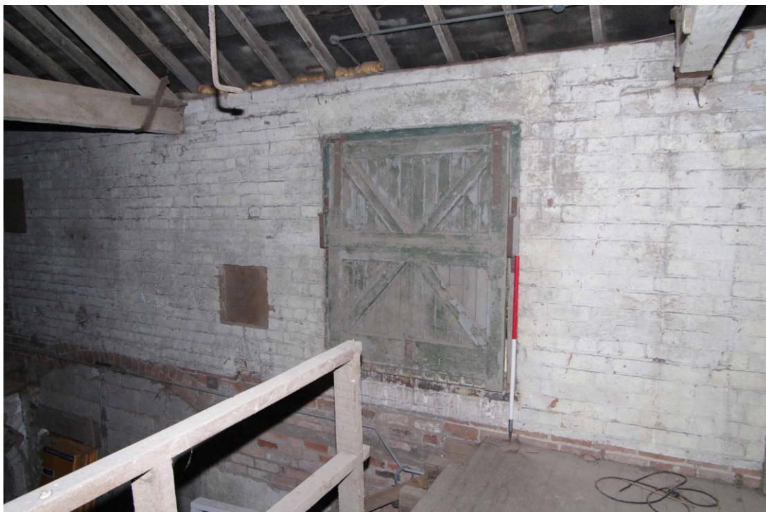
Figure 36: Granary, Room F1 north wall loading door Looking north-west. 1m scale
