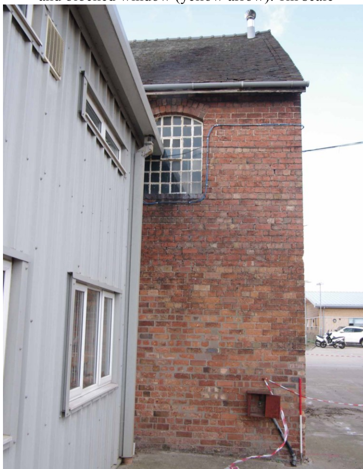
Figure 22: Granary, east end of south facing elevation Looking north. Note difference in ground floor and first floor brickwork. 1m scale
