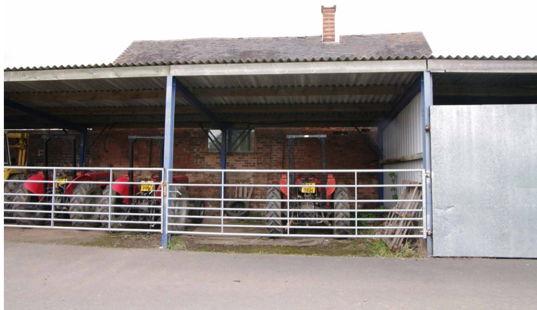
Figure 69 Gasometer building, south facing elevation behind tractor shed Looking north
