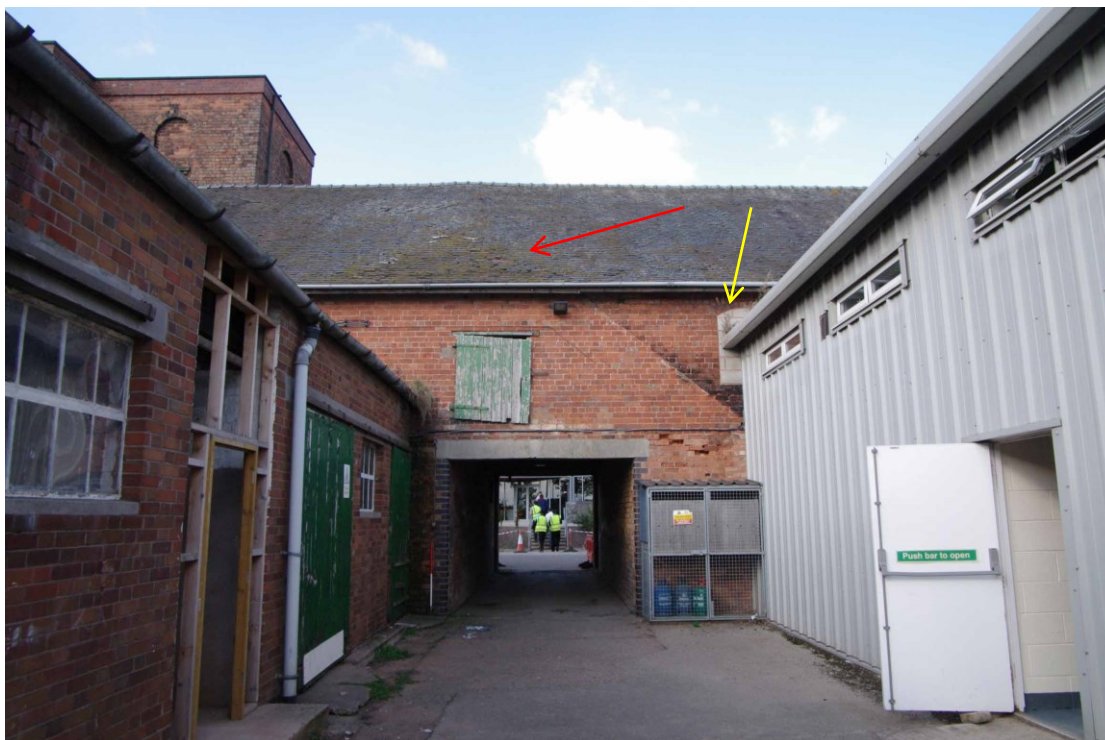
Figure 21: Granary, centre of south-facing elevation Looking north. Note scar on brickwork and roof (red arrow) from earlier rear range and blocked window (yellow arrow). 1m scale
