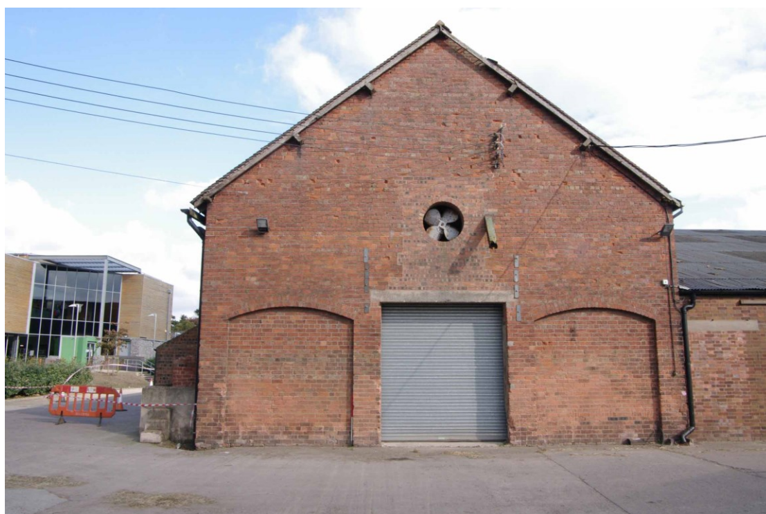
Figure 19: Granary, west facing elevation Looking east. 1m scale
