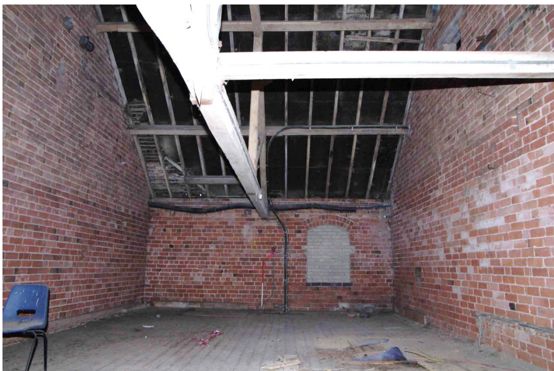
Figure 51: Granary, first floor Room F4 Looking south. 1m scale
