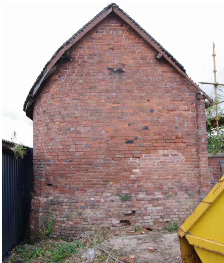
Figure 68 Gasometer building, east facing elevation Looking west
