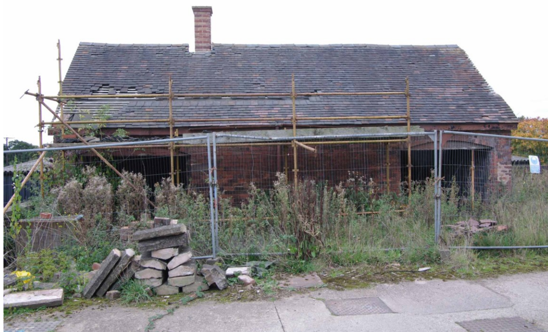
Figure 66 Gasometer building, north facing elevation Looking south
