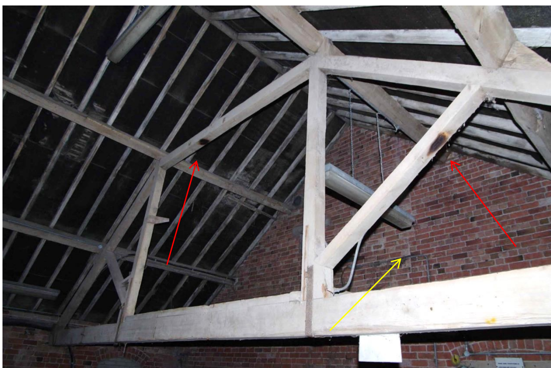
Figure 53: Granary, first floor Room F4 roof detail Looking north-west. Red arrows point to scorch marks, yellow arrow at brick joint of tower wall and room wall
