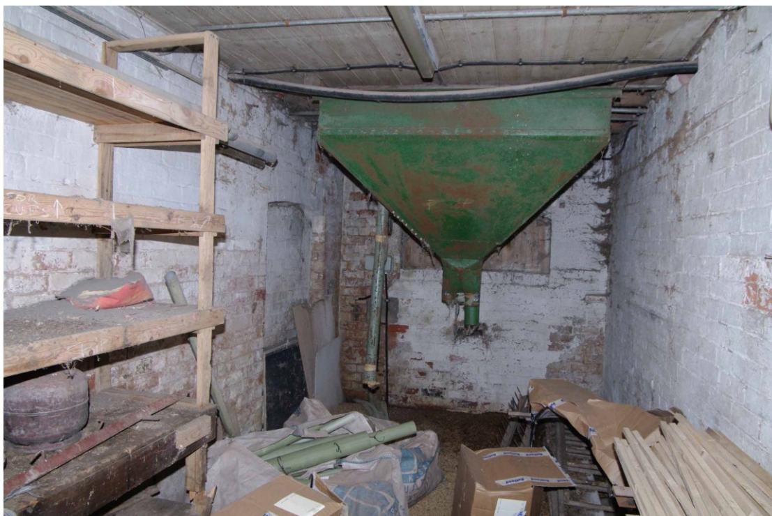
Figure 40: Granary, ground floor Room G5 Looking south-east
