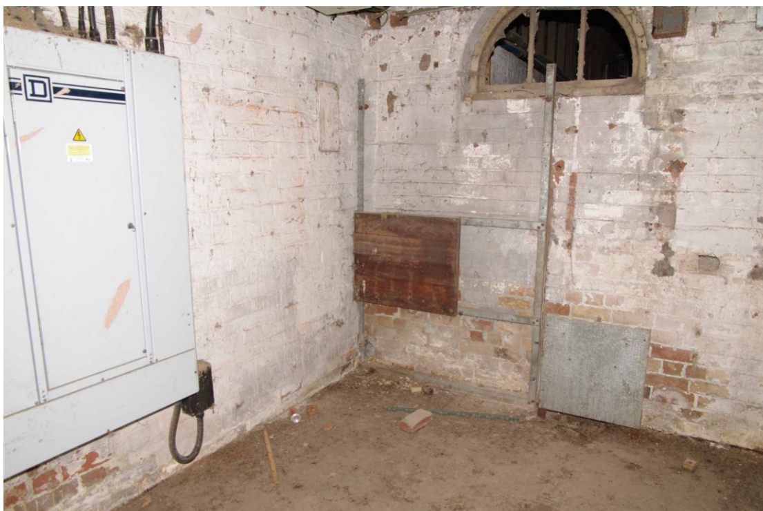
Figure 39: Granary, ground floor. South end of Room G4 Looking south-east
