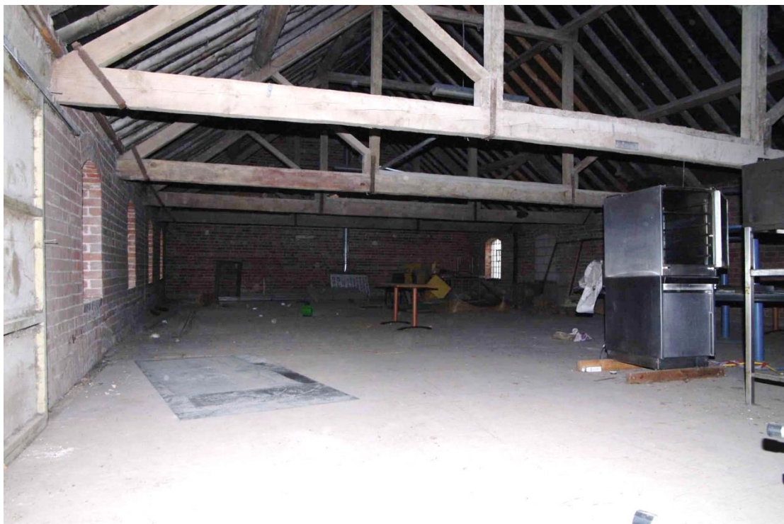
Figure 54: Granary, first floor Room F5 Looking east
