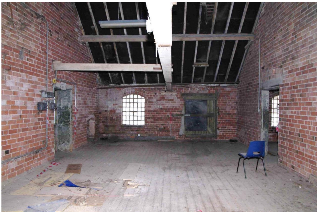
Figure 52: Granary, first floor Room F4 Looking north. 1m scale
