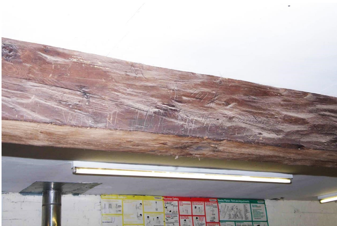
Figure 44: Granary, ground floor Room G7. Raze marks on beam
