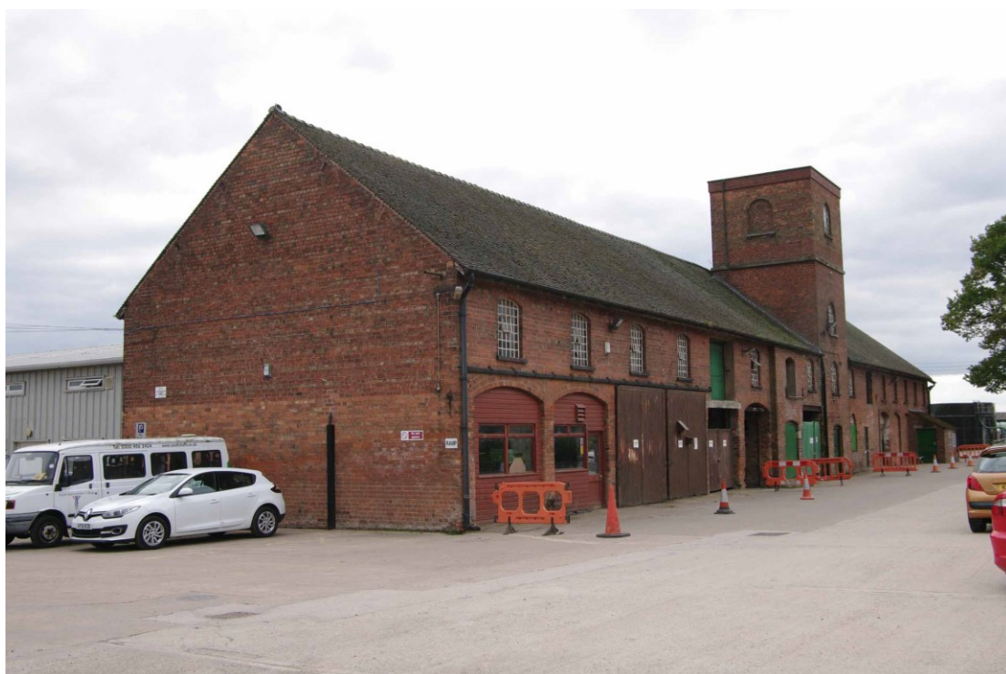
Figure 6: General view of the Granary Looking south-west. South-eastern range of Granary buildings on far left of picture
