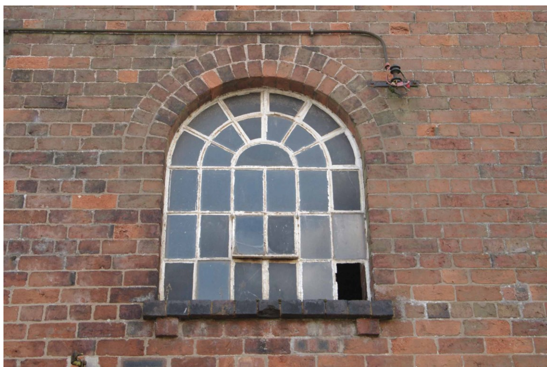
Figure 16: Granary tower window detail Looking south, First floor
