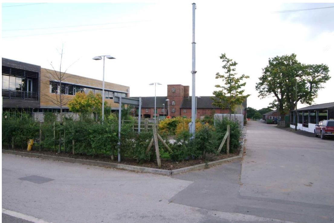
Figure 8: Granary and new building from the north Looking south
