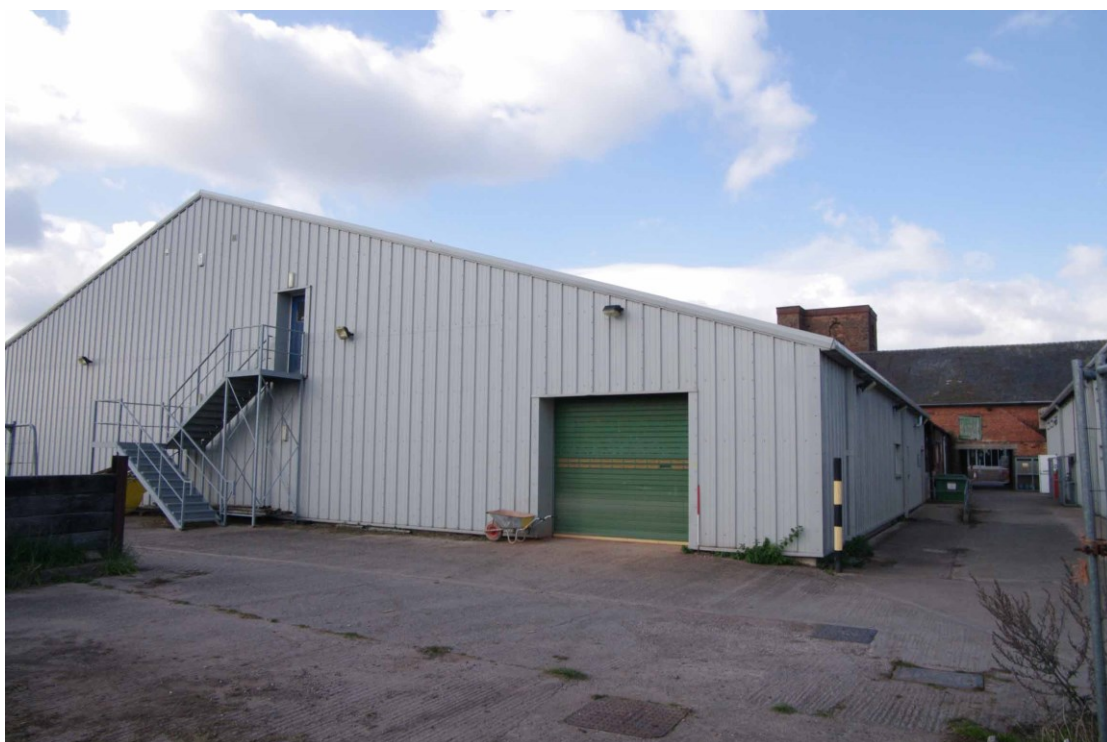
Figure 60: South-western rear range Looking north-west. 1m scale
