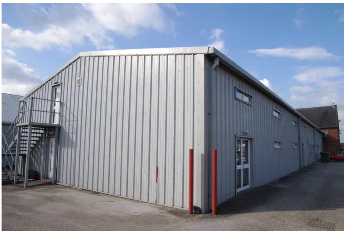
Figure 64: South-eastern rear range. South and east facing elevations Looking north-west. 1m scale
