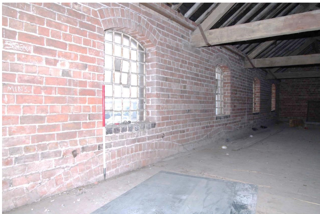
Figure 56: Granary, first floor Room F5 north wall Looking north-east. 1m scale
