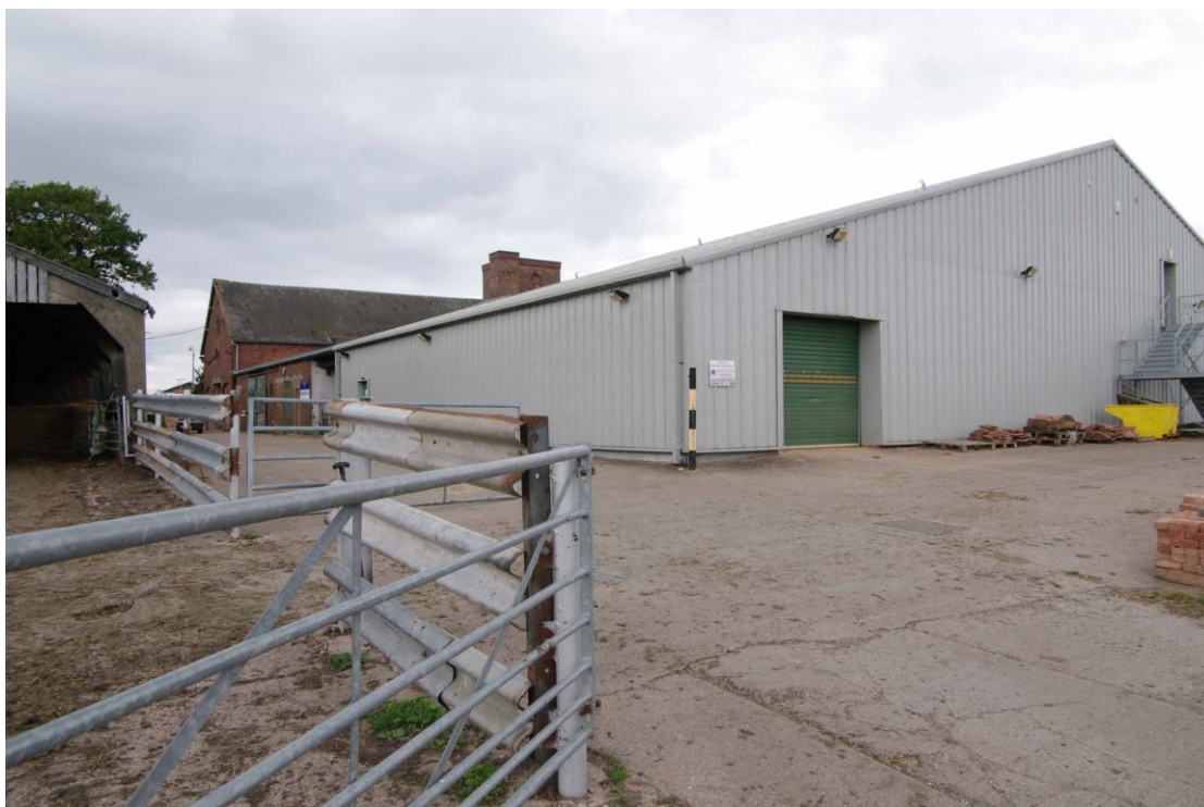
Figure 59: South-western rear range Looking north-east
