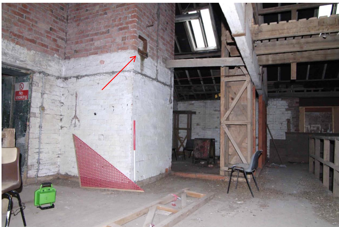
Figure 35: Granary, Room F1 mezzanine Looking south-east. Arrow shows location of bearing box. 1m scale
