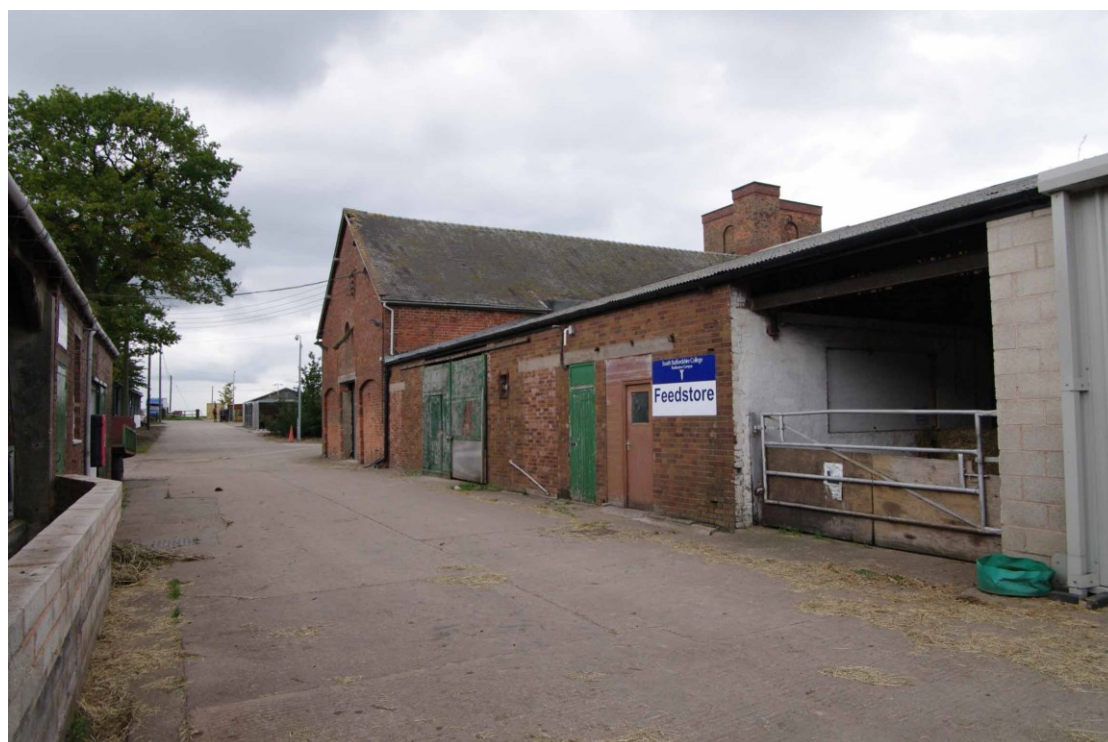
Figure 20: Granary, east end of south facing elevation Looking north-east
