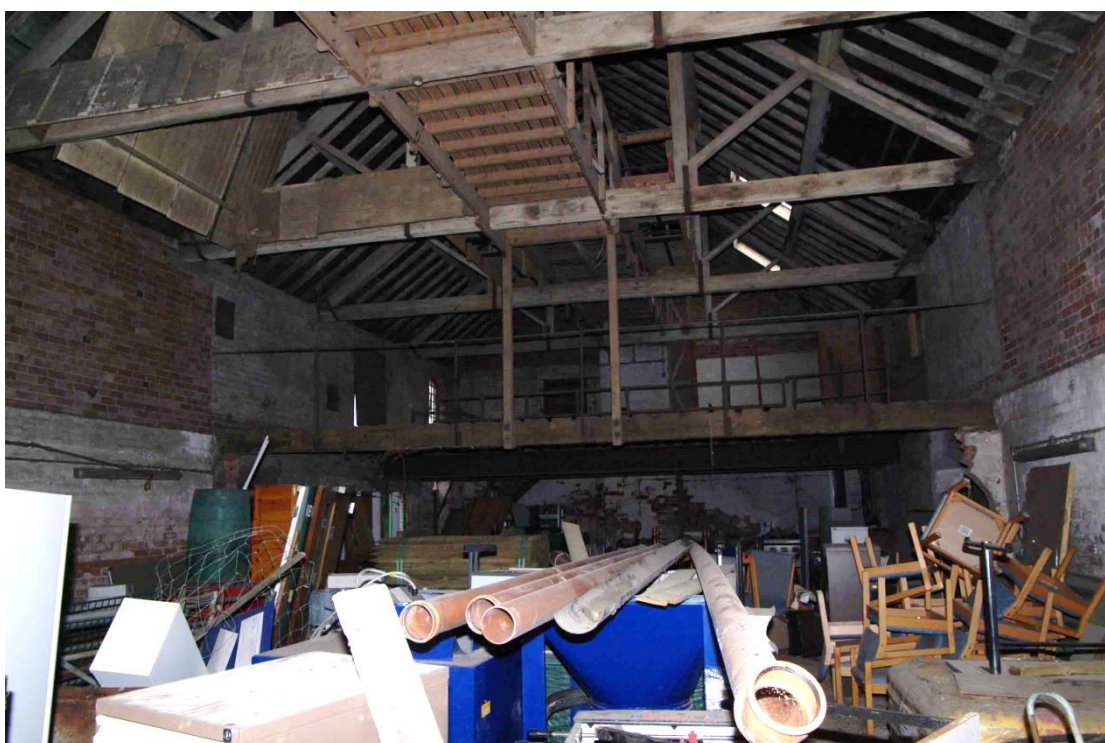
Figure 27: Granary, ground floor Room G1 Looking east
