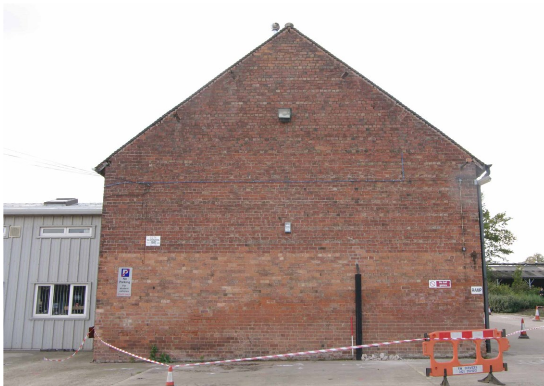
Figure 23: Granary, east facing elevation Looking west. 1m scale
