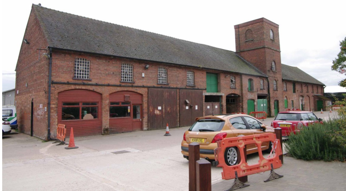
Figure 12: Granary, north facing elevation, eastern end Looking south-west
