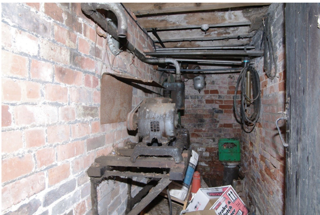
Figure 14 Unit 1, Building 1 passageway adjacent to northernmost room Looking south-east
