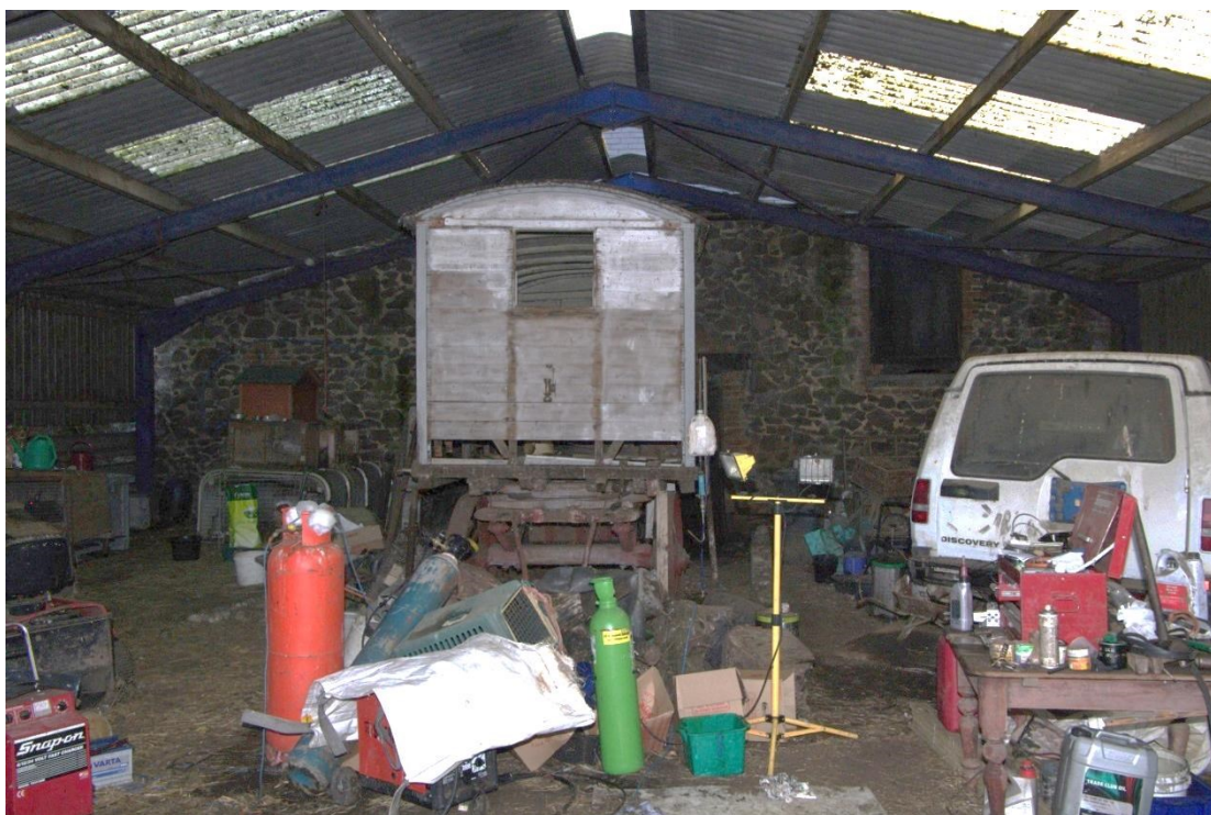
Figure 34 Unit 2, Barn north-west facing elevation Looking south-east. Central doorway is behind the living van
