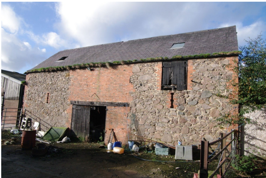
Figure 30 Unit 2, Barn south-east facing elevation Looking west
