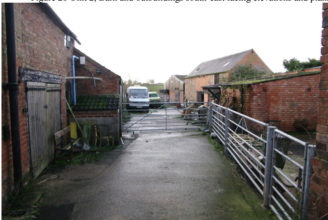
Figure 29 Unit 2 buildings seen from the yard Looking south-east. Unit 1 buildings on left of picture. Outbuildings in foreground on right of picture
