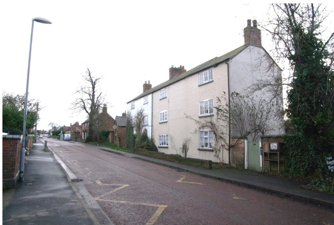
Figure 3 Limes Farmhouse Looking south-east along Main Street. Number 11 is the cream coloured building Number 15 is the white building
