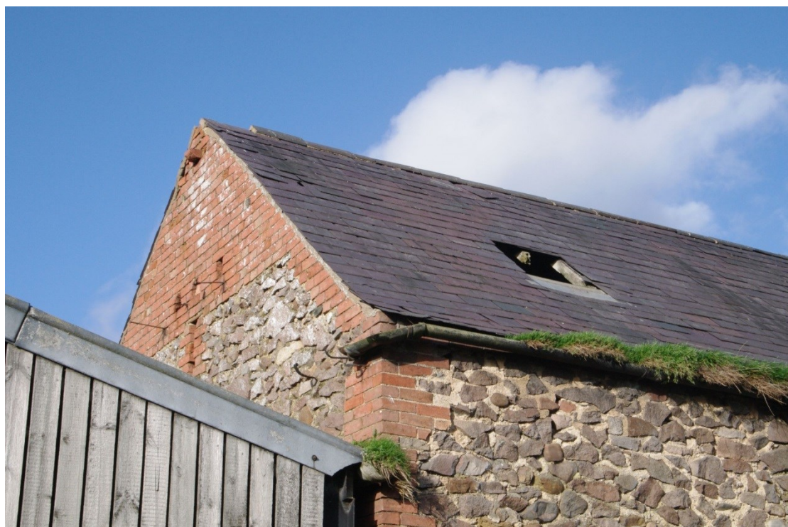
Figure 32 Unit 2, Barn south-west facing gable end Looking north
