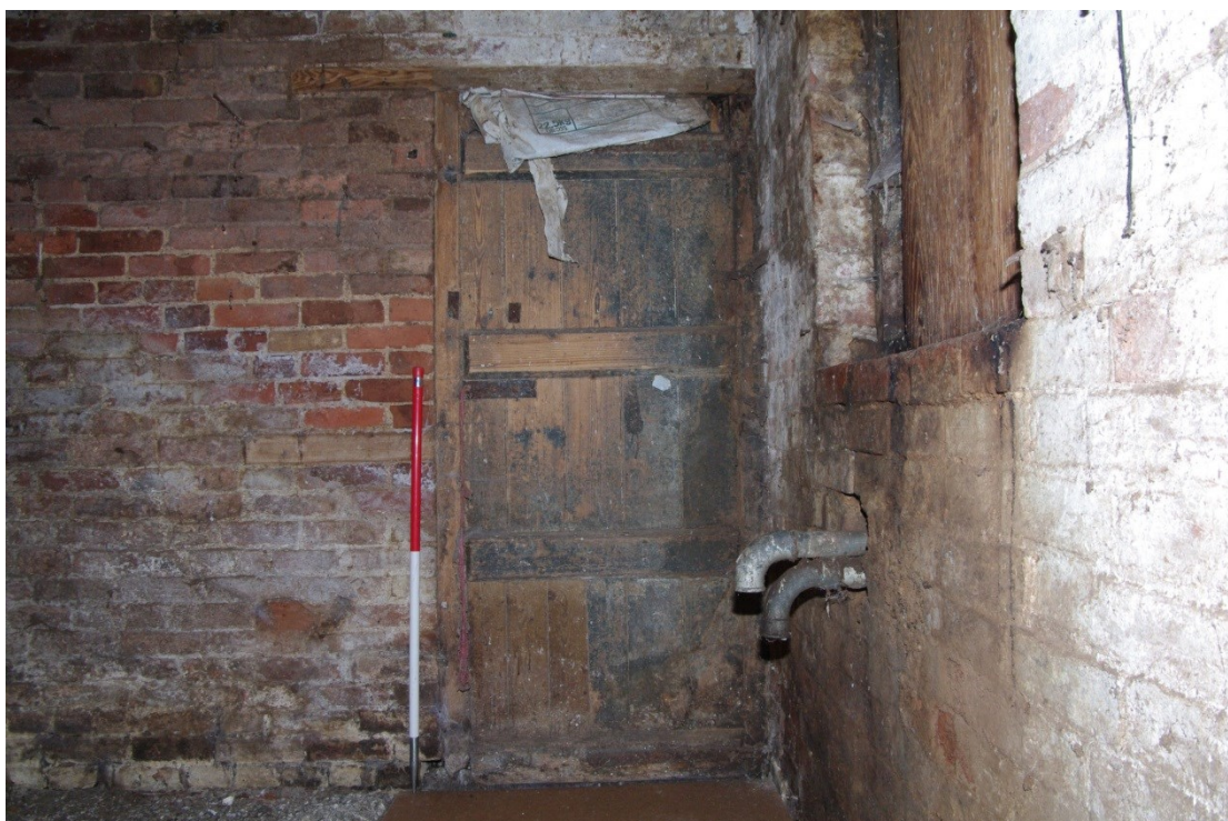
Figure 16 Unit 1, Building 1 south room. Door to Building 2 Looking south-east. 1m scale
