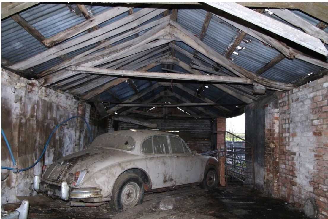
Figure 27 Unit 1, Building 4 inside Looking south-west
