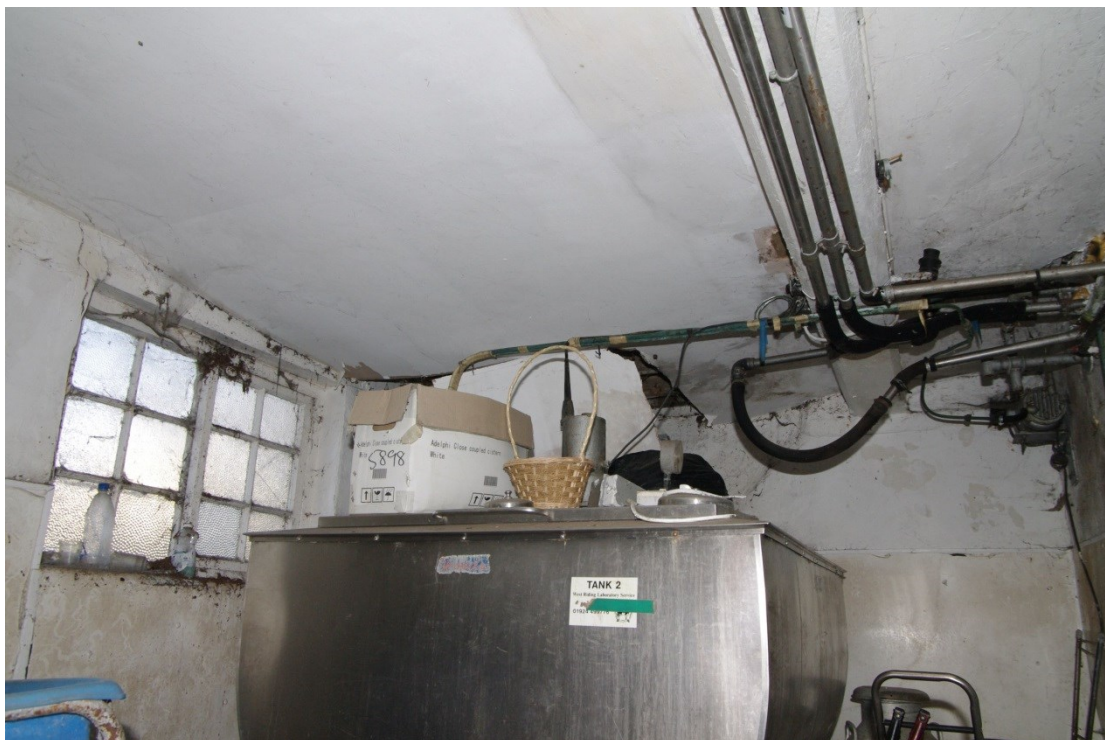
Figure 13 Unit 1, Building 1 northern room Looking east
