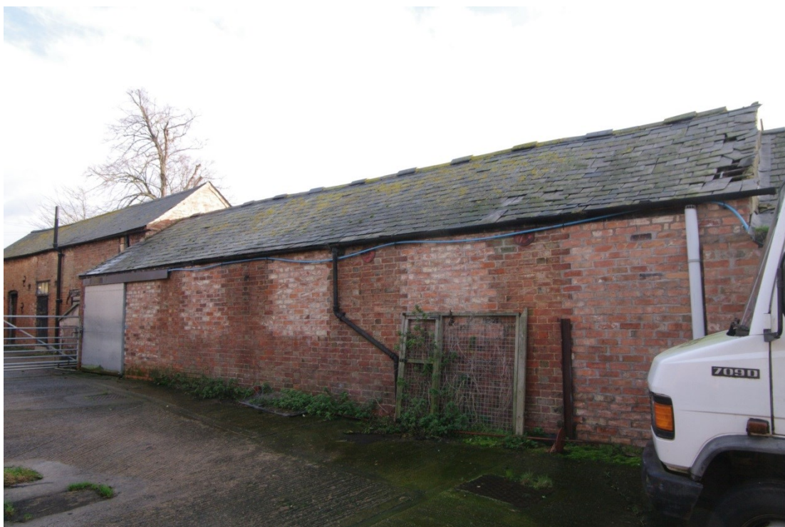
Figure 19 Unit 1, Building 2 north-west facing elevation Looking north-east
