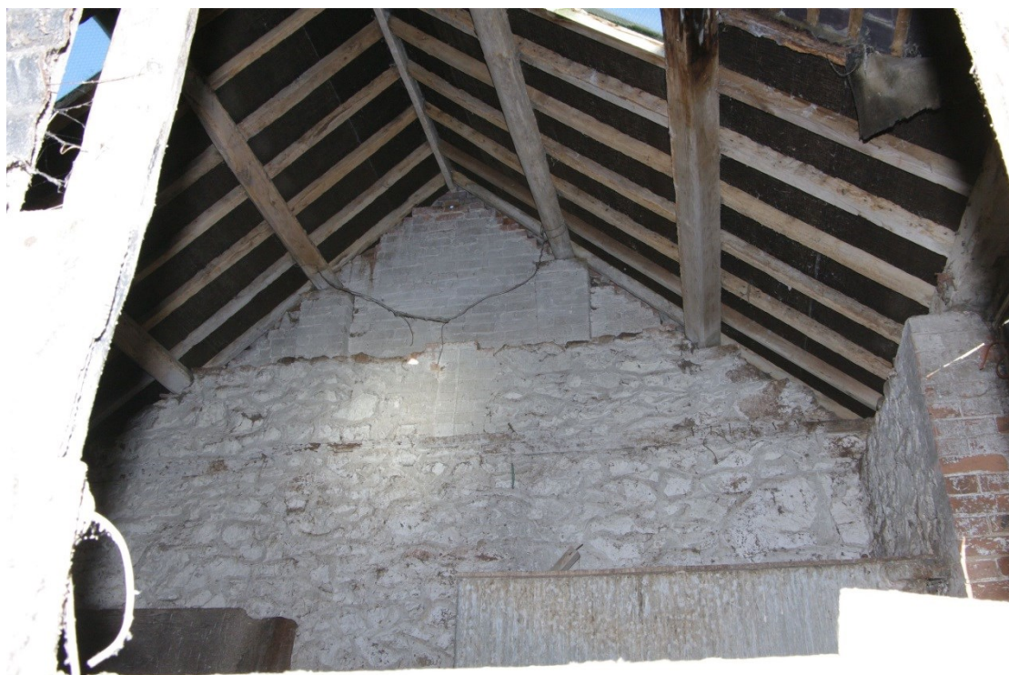
Figure 36 Unit 2, Barn mezzanine Looking north
