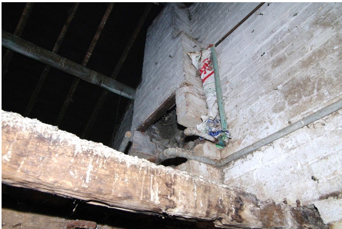
Figure 17 Unit 1, Building 1 south room mezzanine floor Looking south from ground floor
