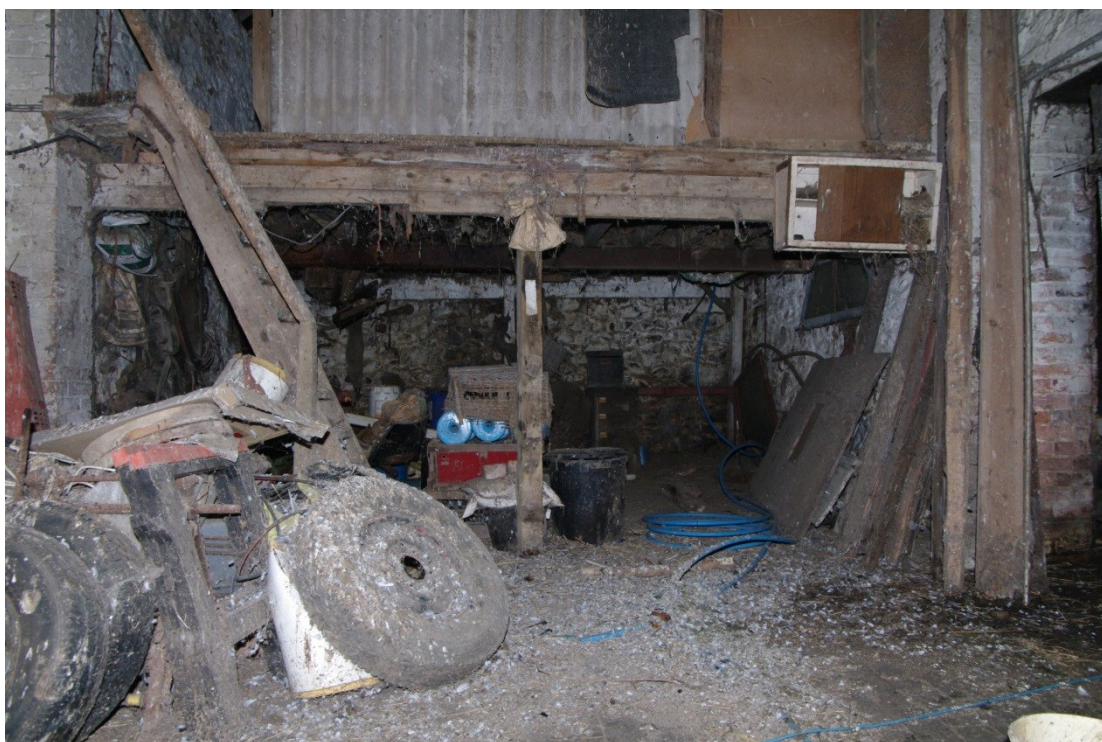
Figure 35 Unit 2, Barn ground floor Looking south-west
