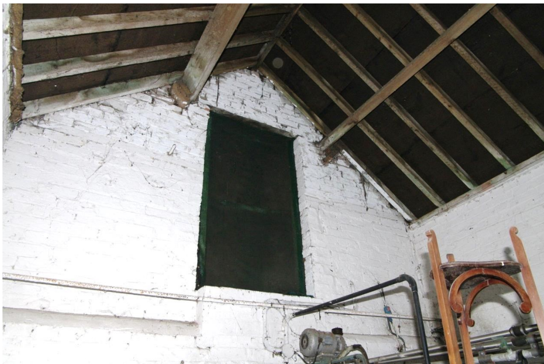
Figure 15 Unit 1, Building 1 centre room Looking north-east
