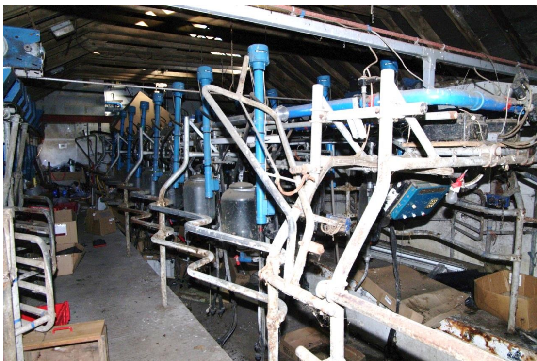
Figure 20 Unit 1, Building 2 interior Looking north-east
