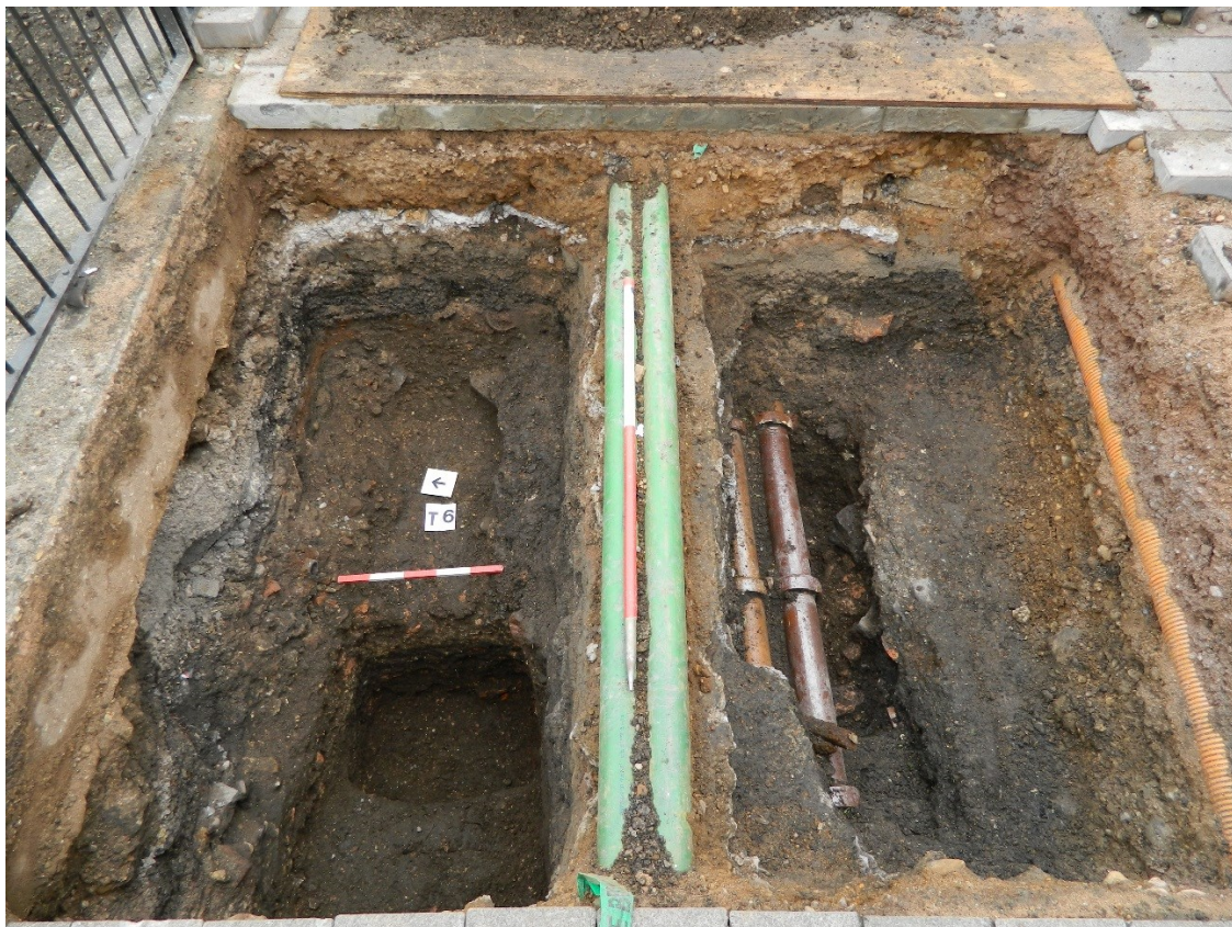
Figure 31: View of trench 6
