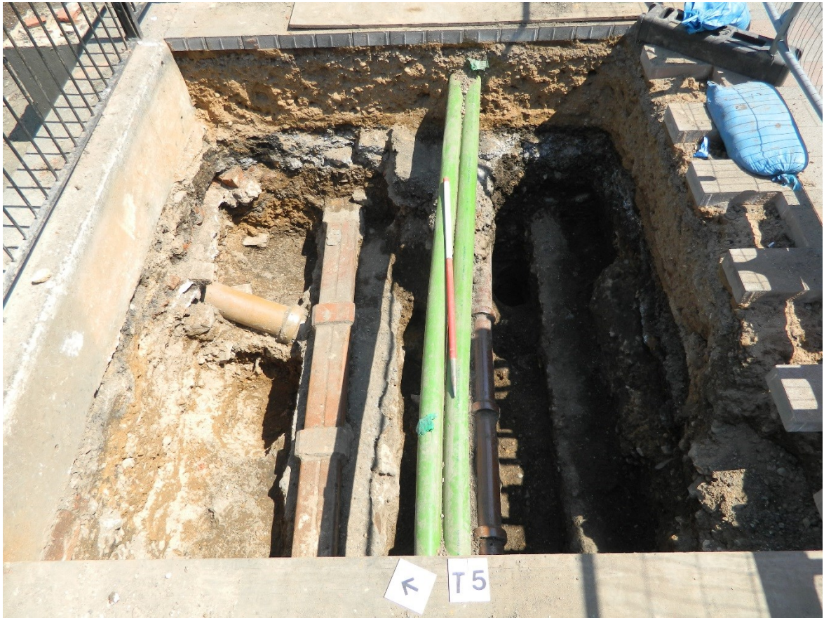
Figure 26: View of Trench 5
