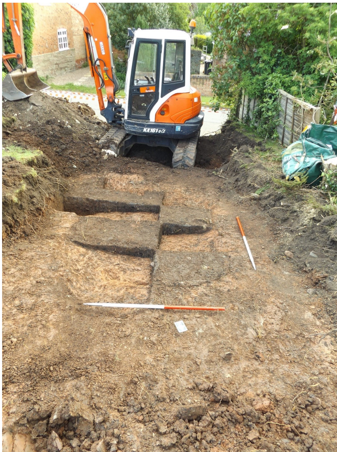
Figure 5: Pits [4] and [6], looking south, located during the initial phase of monitoring.
