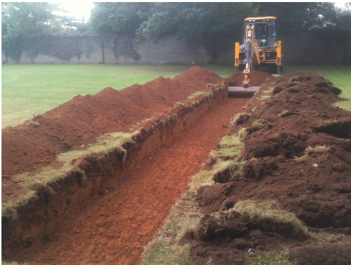
Plate 4: Work in progress on Trench 02, looking south
