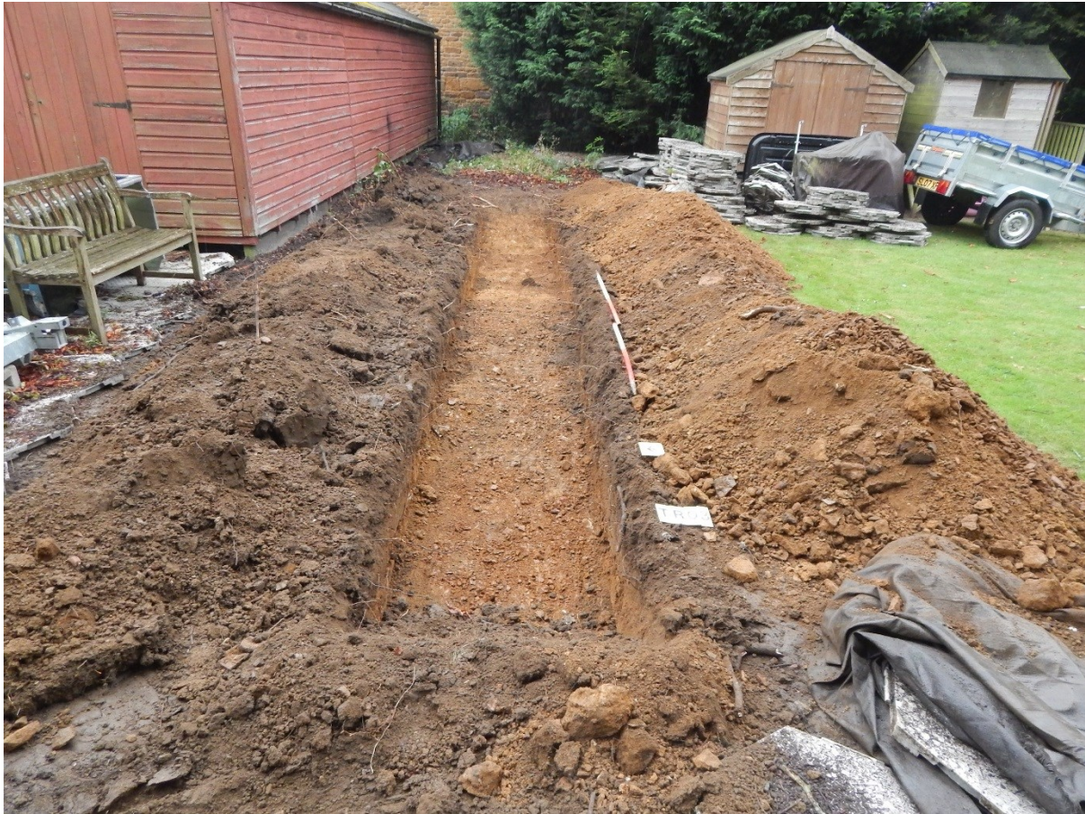
Plate 7: Post excavation shot of Trench 03, looking east
