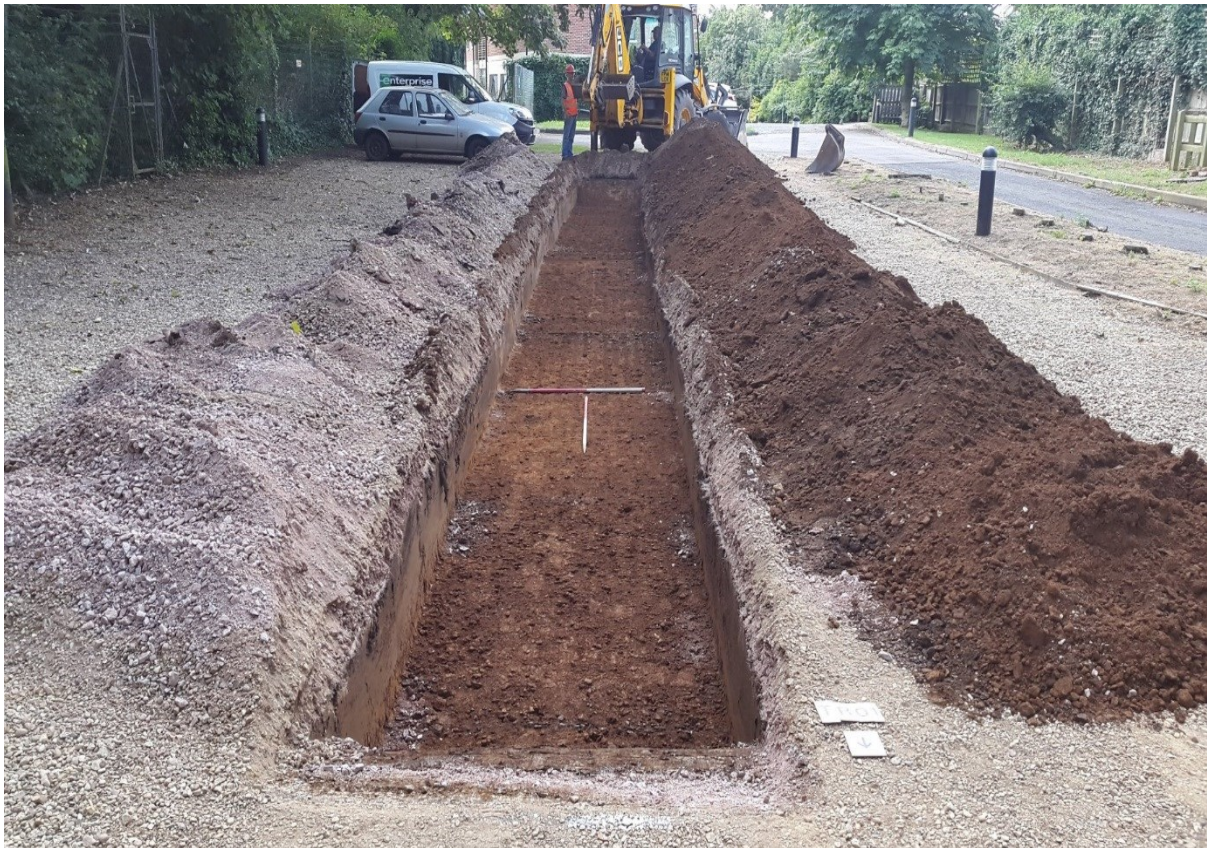
Plate 2: Post excavation view of Trench 01, looking south
