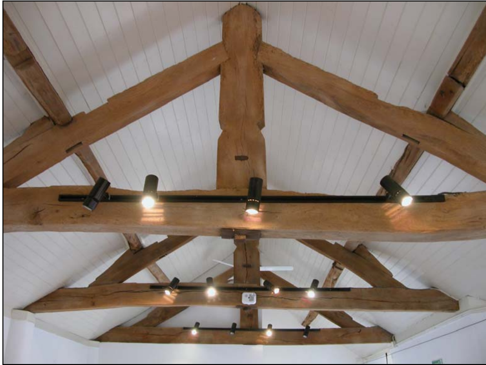
Fig. 11. King-post trusses within building A.
