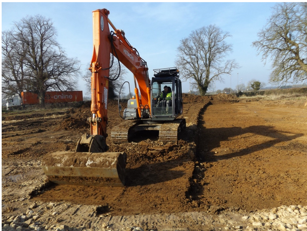
Figure 6: Stripping the eastern part of site
